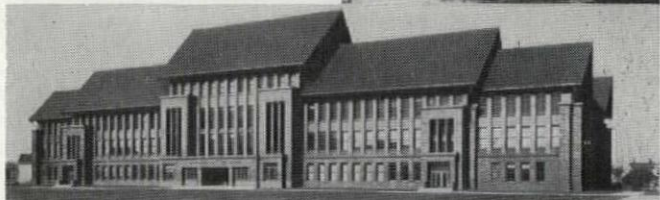
THE INCREASE IN SCALE became a problem of unprecedented magnitude. The skyscraper won world recognition as a new and characteristic American architectural form. But equally the large hotel, department store, bank, and even the large school were typical. For example—here is CARL SCHURZ HIGH SCHOOL
