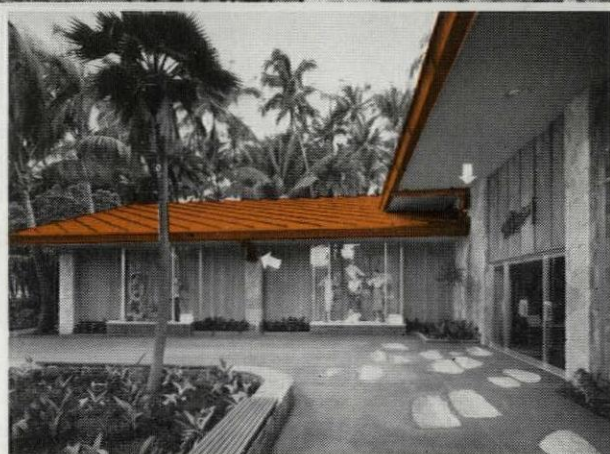
ENTRANCE TO THE fabulous McInerny Waikiki Store. Known as "The Jewel of the Pacific," it is one of the show places of the world, and is in Honolulu, Hawaii. Note how copper gutters blend into roof line; also unique treatment of down spouts (arrows).
