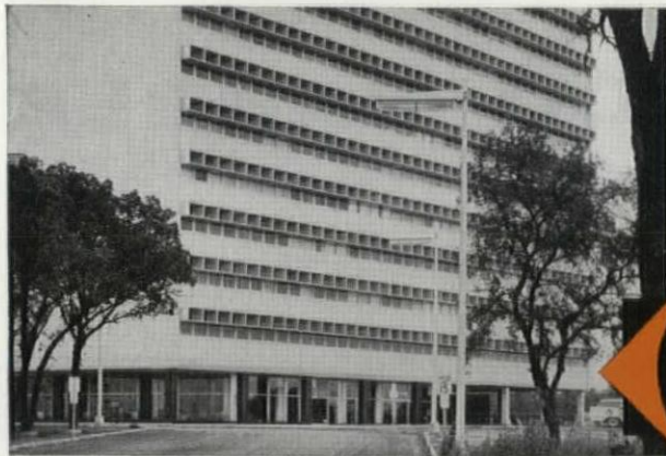
Exchange Bank and Office Building, Dallas, Tex., featuring all welded steel tube curtain wall framing. (Lane, Gamble & Assoc.)
