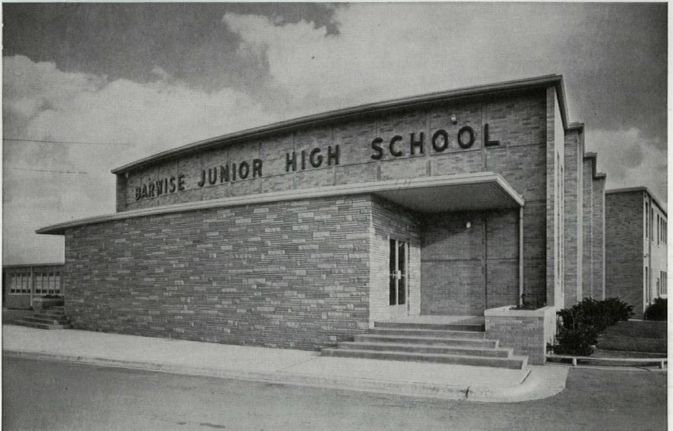
Project: Barwise Junior High School, Wichita Falls, Texas. Architects: Jesse G. Dixon, Arch., R. B. Pardue, Asso., Wichita Falls, Texas. General Contractor: W. C. Shelton, Lawton, Okla. Masonry Contractor: W. P. Howle, Wichita Falls, Texas. Dealer: Stephens Lumber Co., Wichita Falls, Texas.
