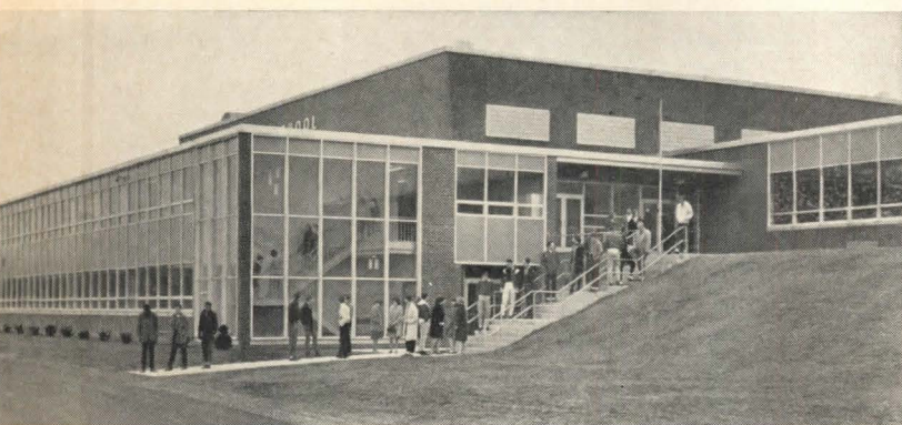
$63,000 SAVING: 675-student, 60,000 sq. ft. Hampshire High School, Romney, W. Va. Architect: Robert J. Bennett, Morgantown, W. Va. Engineer: Ballard & Mayfield, Canton, Ohio. Contractor: Baker & Coombs, Inc., Morgantown, W. Va.
