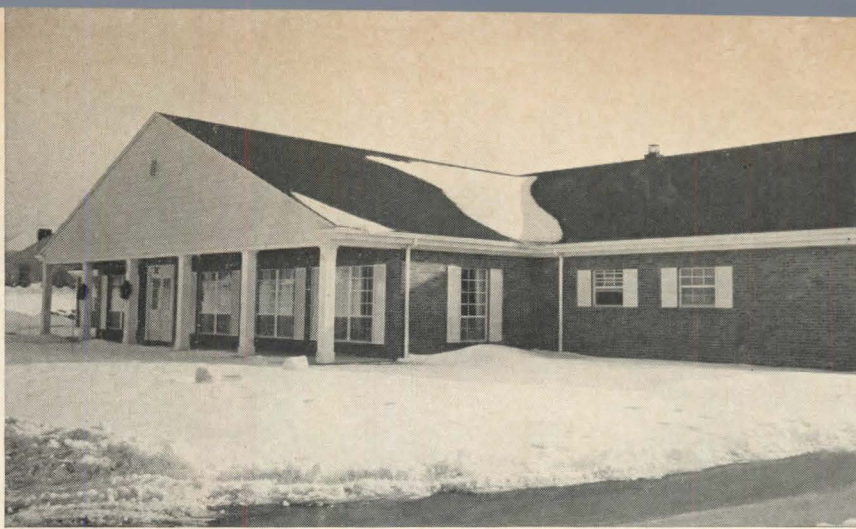
$20,000 SAVING: 19,000 sq. ft. Den-Mar Nursing Home, Rockport, Mass. Architect: Di Meo Associates, Stoneham, Mass. Engineer: Joseph Sestito & Associates, Malden, Mass. Contractor: Feldman Construction Co., Rockport, Mass.
