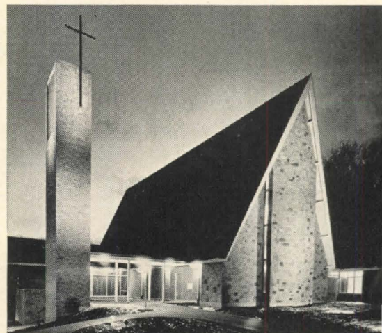
$10,000 SAVING: 18,500 sq. ft. Gloria Dei Lutheran Church, Forestville, Conn. Architect: Jeter & Cook, Hartford, Conn. Engineer: James S. Minges & Associates. Contractor: Wadhams and May Co.
