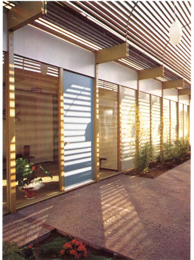
Lustrous, obscure 7/32" BURLAP glass in office building, Bellflower, Calif. Owners, Builders and Architects: Lane and Brodie Glass: Downey Glass Company Glazing: Hal's Glass Company
