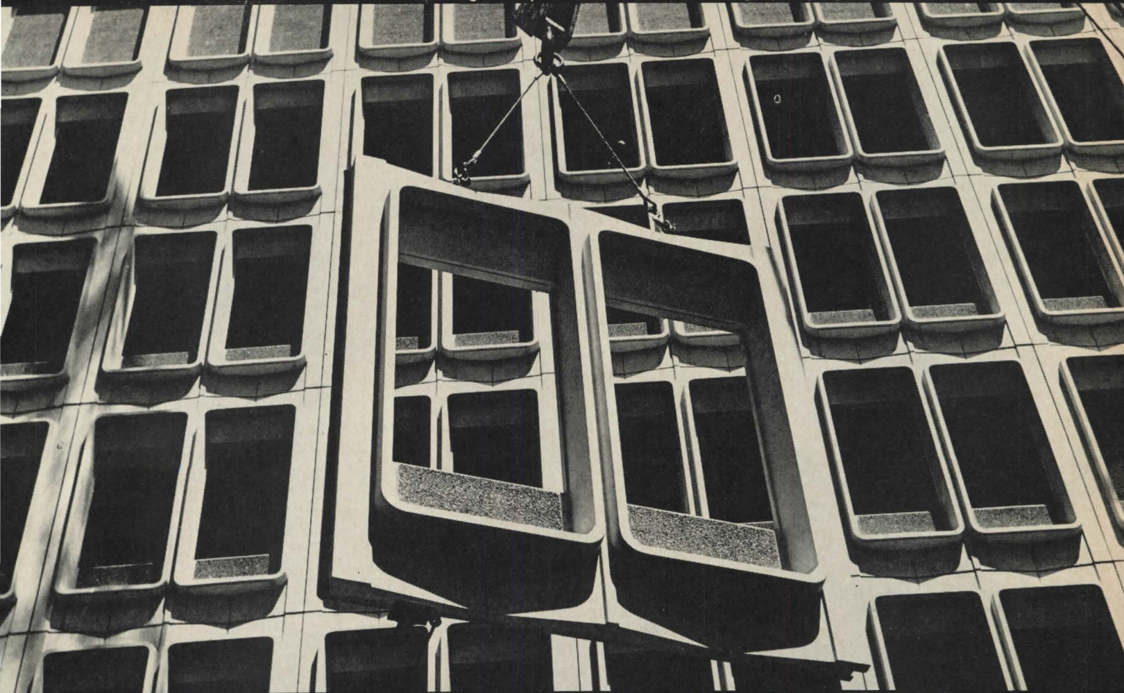
Schokbeton precast concrete double-window curtain wall unit, Sir George Williams University, Montreal, Canada Architect: Ross, Fish, Duchesnes & Barrett. Schokbeton by Schokbeton Quebec, Inc.
