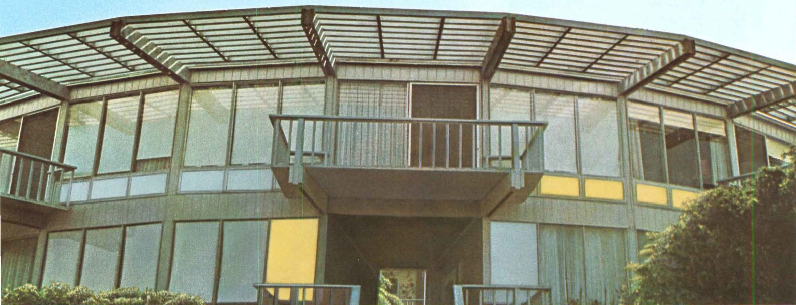
GLASWELD INSTALLED APRIL 1960, PHOTO TAKEN JUNE 1968.
