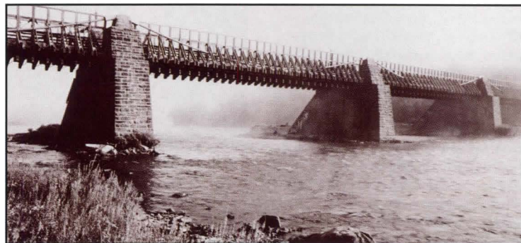
The Delaware River Aqueduct. Its restoration won a Presidential Design Award.
