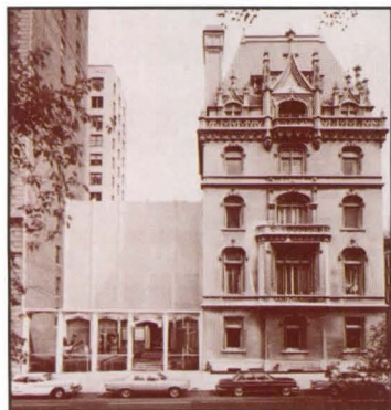
Museum with existing 1962 addition.
