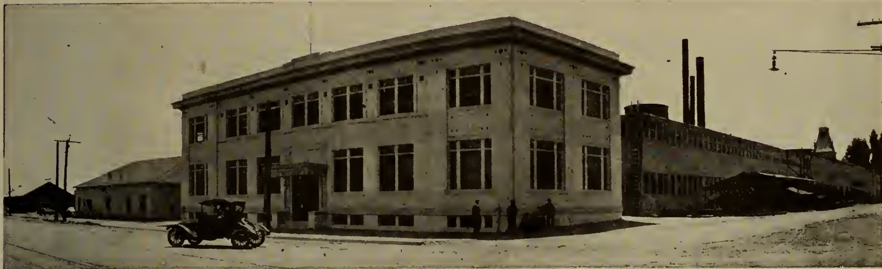
PACIFIC MANUFACTURING COMPANY PLANT, SANTA CLARA, CALIFORNIA
