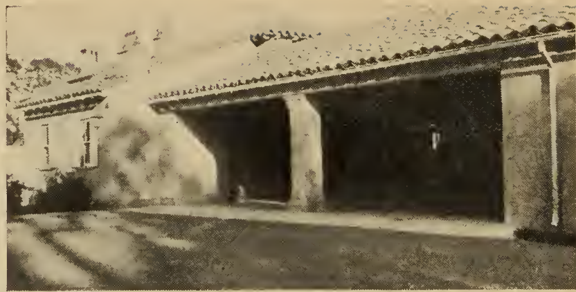
GARAGE RESIDENCE OF ROBERT S. MOORE ALBERT FARR, ARCHITECT
