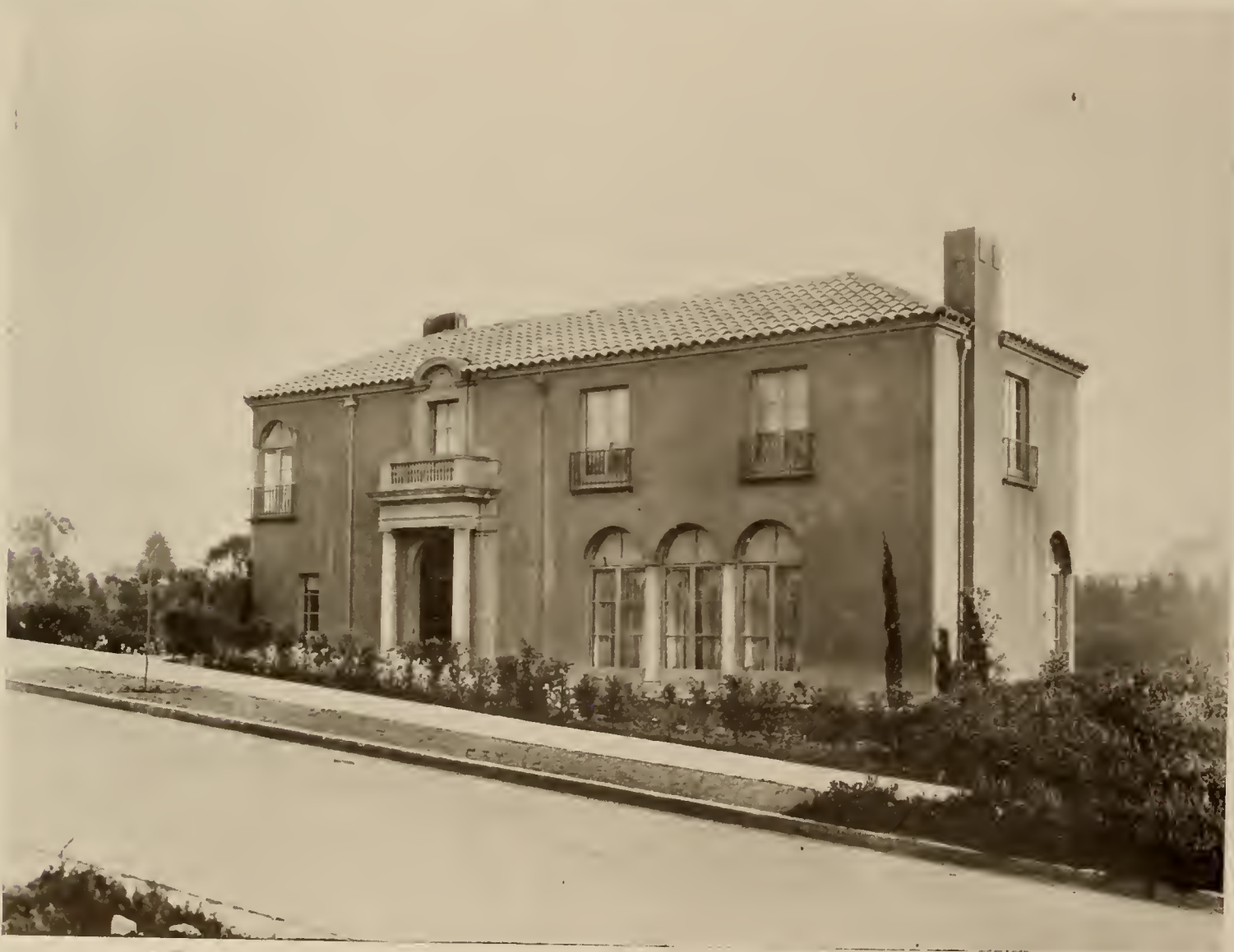
RESIDENCE OF DR. AUSTIN F. CLARKE LAKESHORE HIGHLANDS, OAKLAND, CALIFORNIA CHAS. W. McCALL, ARCHITECT
