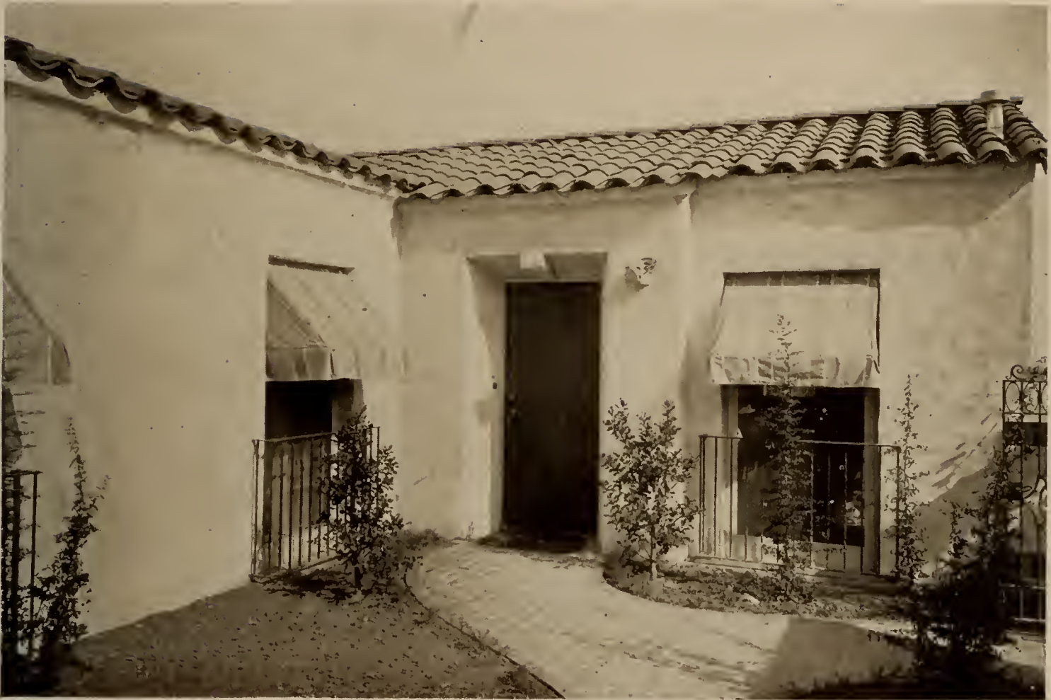
PATIO, RESIDENCE OF MR. S. W. P. STRELINGER BEVERLY HILLS, CALIFORNIA H. H. WHITELEY, ARCHITECT
