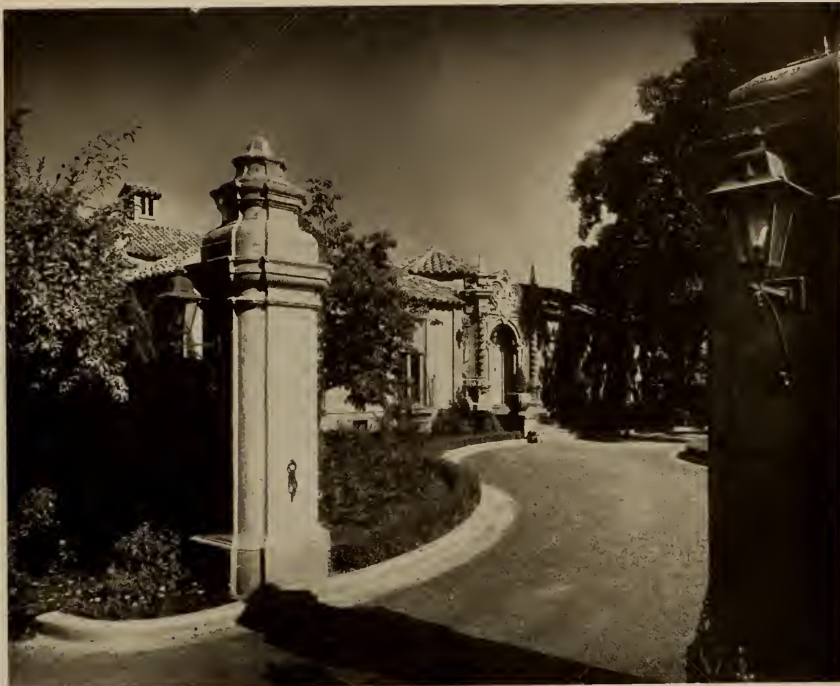
CARRIAGE COURT GATEWAY, RESIDENCE OF ROBERT S. MOORE MENLO PARK, CALIFORNIA ALBERT FARR, ARCHITECT
