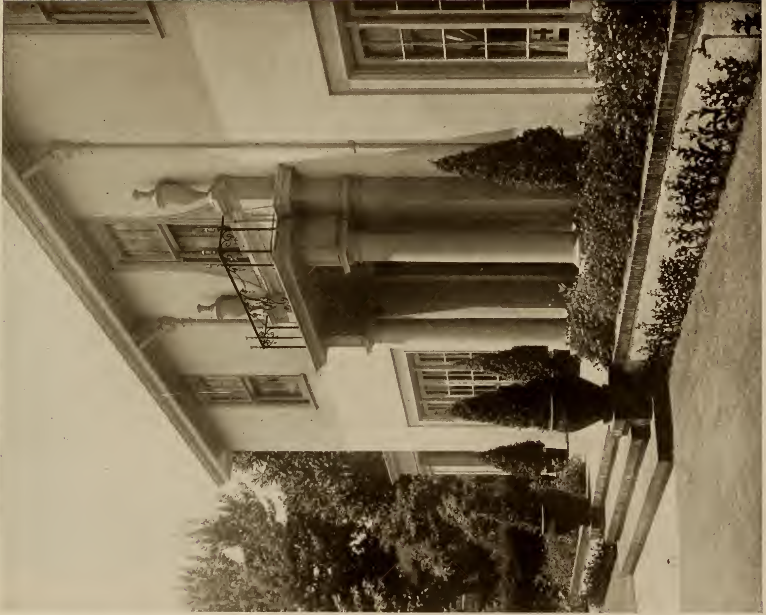
DETAIL OF ENTRANCE AND TERRACE RESIDENCE OF MRS. E. C. HUGHES PALO ALTO, CALIFORNIA J. K. BRANNER, ARCHITECT
