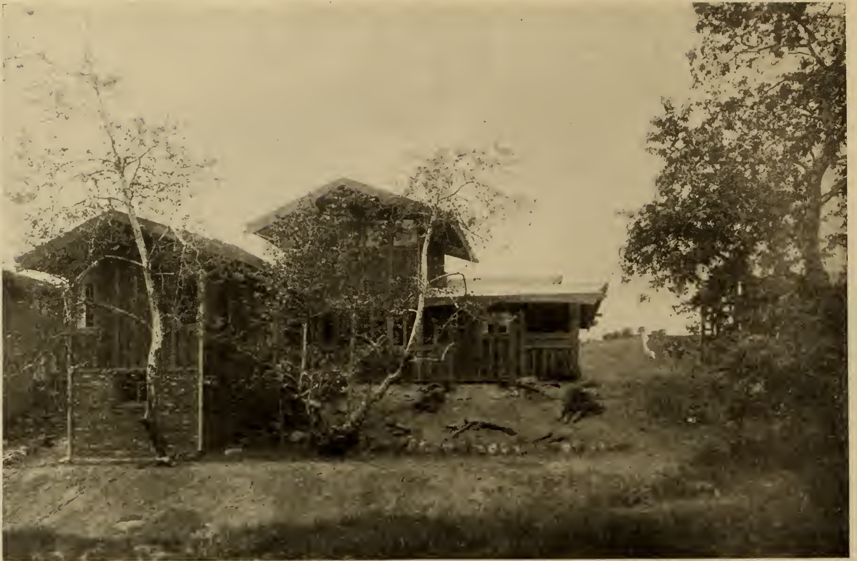
THE TREES "COMPOSE" AS THOUGH THEY HAD BEEN PLANTED PURPOSELY—BUT IT WAS REALLY THE HOUSE BUILT TO FIT THE TREES
