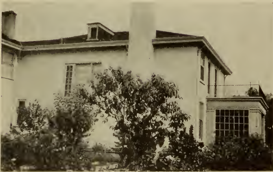
GARDEN SIDE OF MRS. HUGHES' RESIDENCE Palo Alto, California J. K. Branner, Architect
