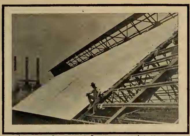
ASBESTOS CORRUGATED ROOFING BEING APPLIED
