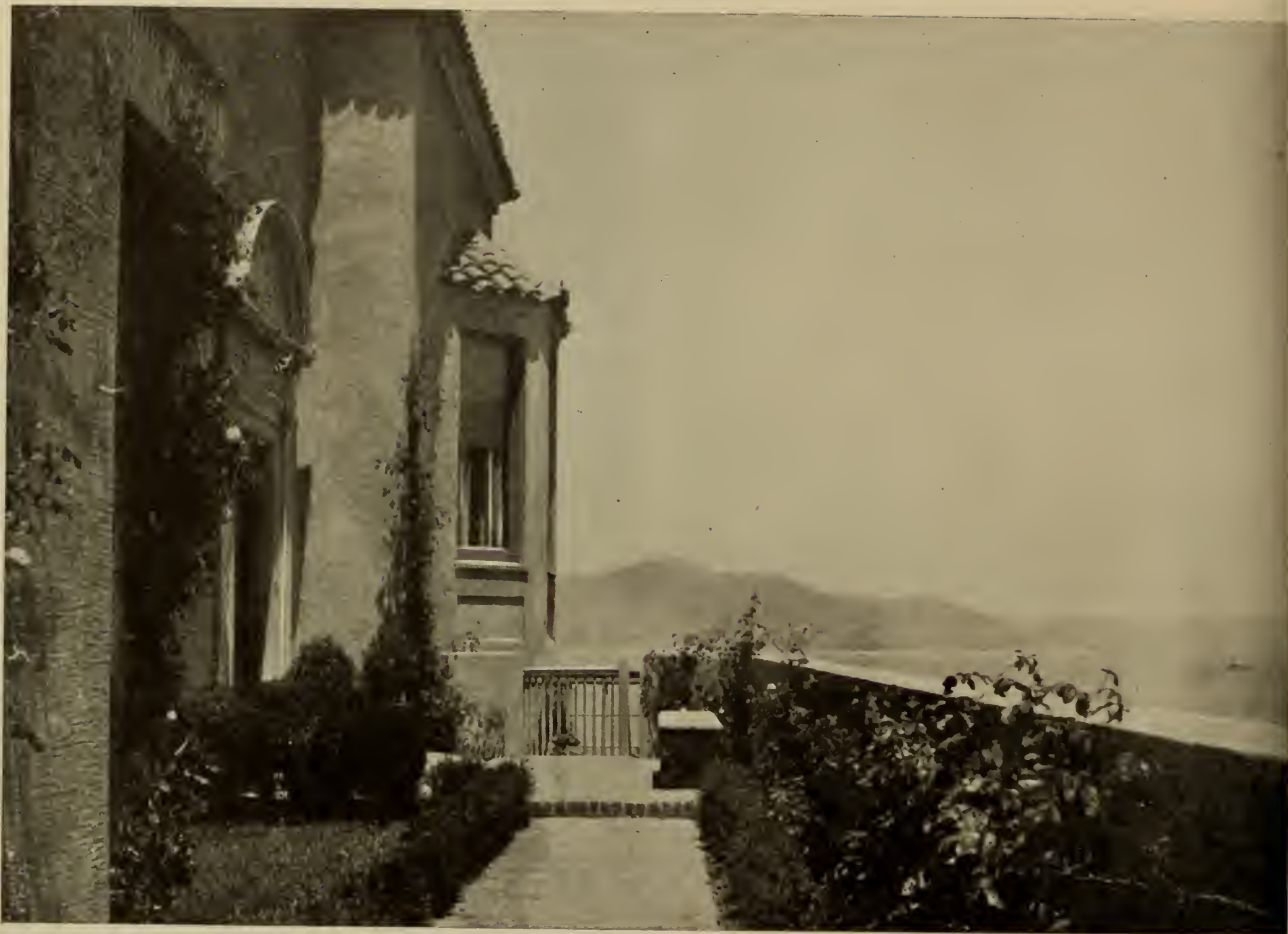
MAIN ENTRANCE WALK.
