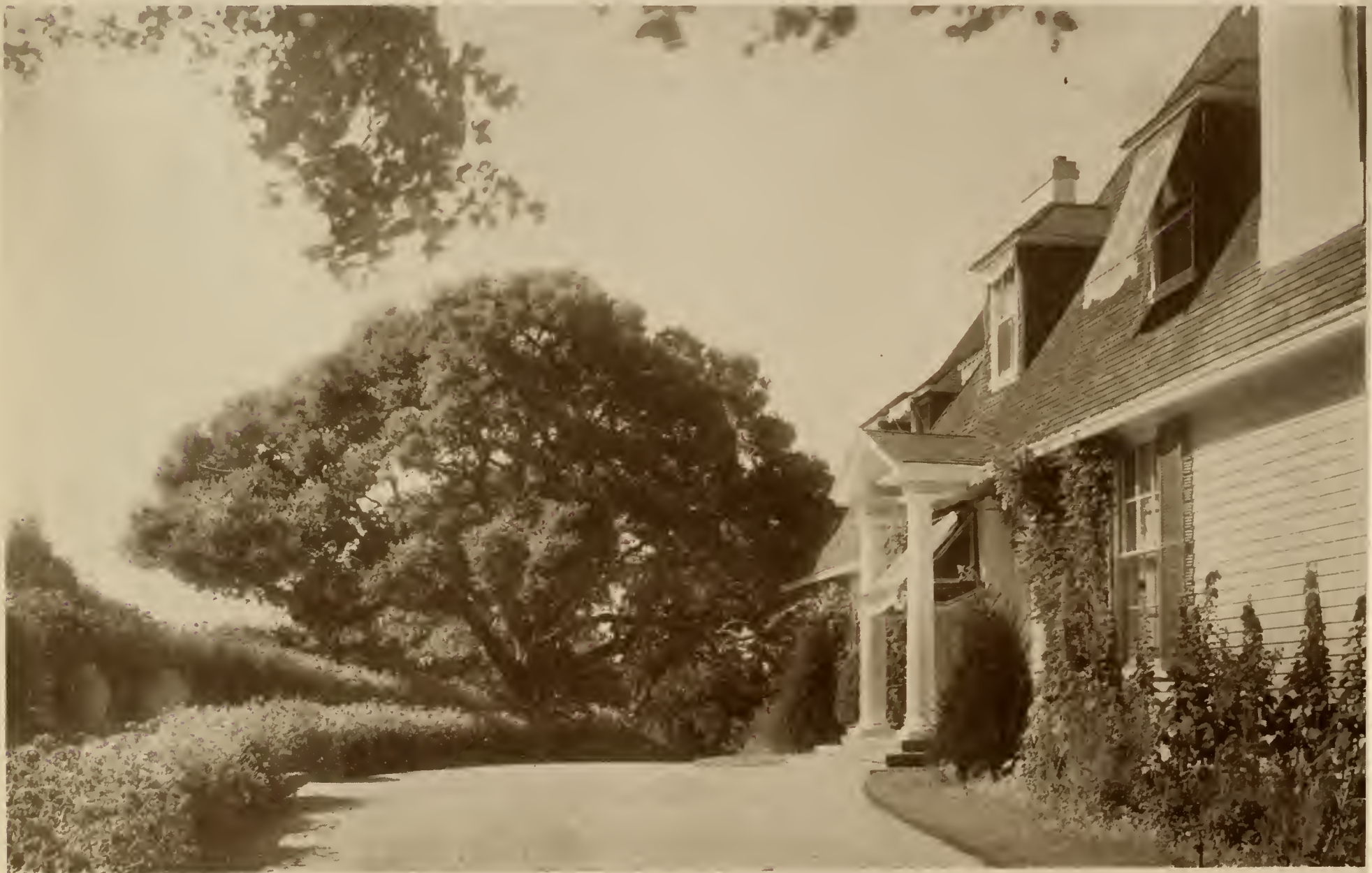
RESIDENCE ON ESTATE OF GEORGE LENT, REDWOOD CITY BAKEWELL & BROWN, Architects
