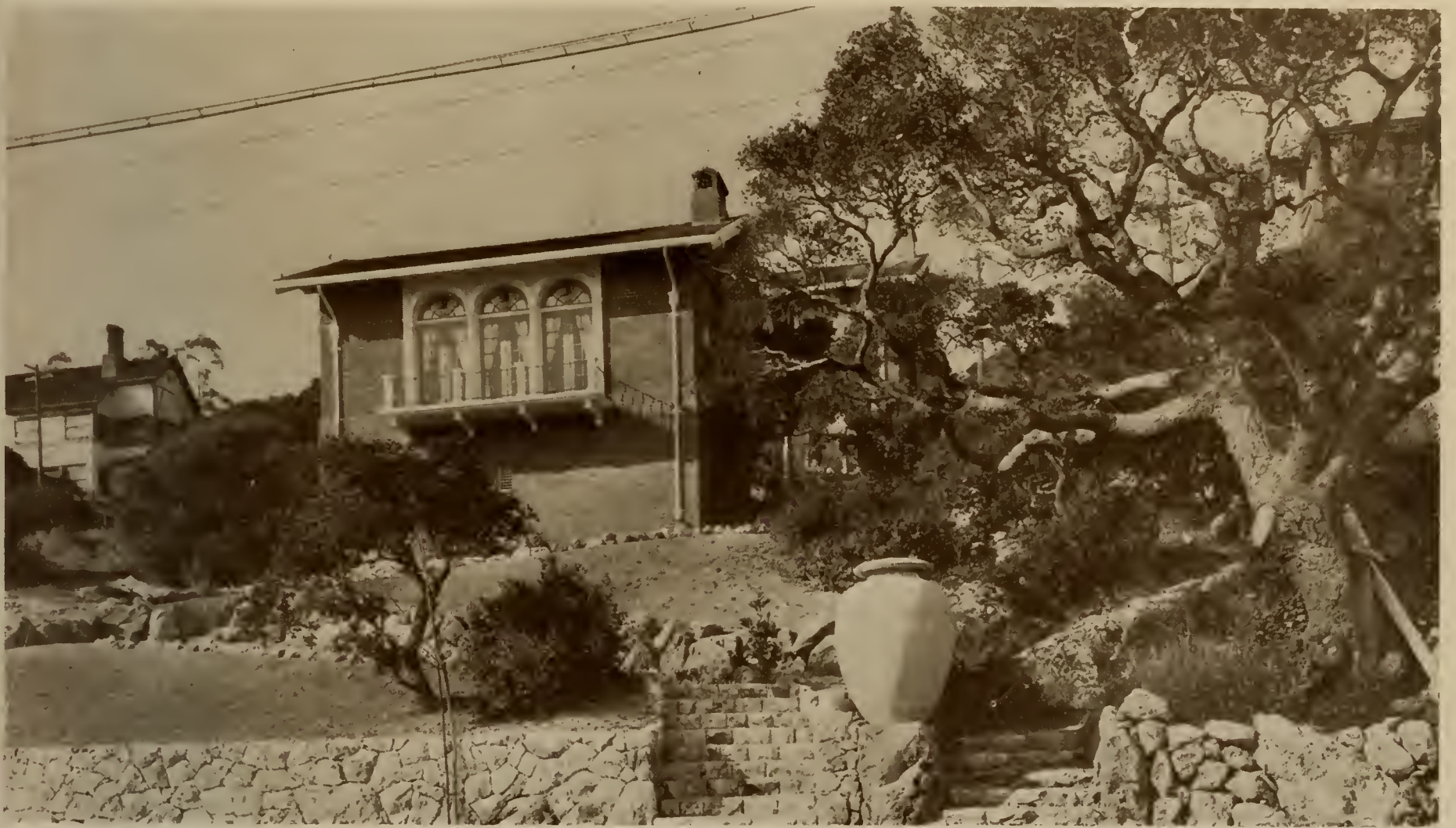
RESIDENCE OF CHARLES W. BROCK, THOUSAND OAKS, BERKELEY HENRY H. GUTTERSON, Architect
