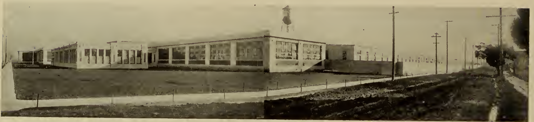
AMERICAN CAN COMPANY PLANT.
