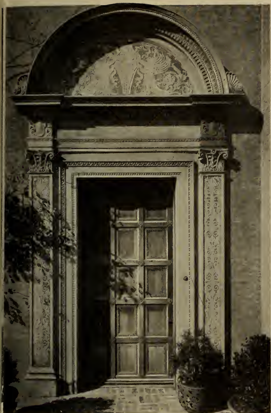
DETAIL OF MAIN DOORWAY
