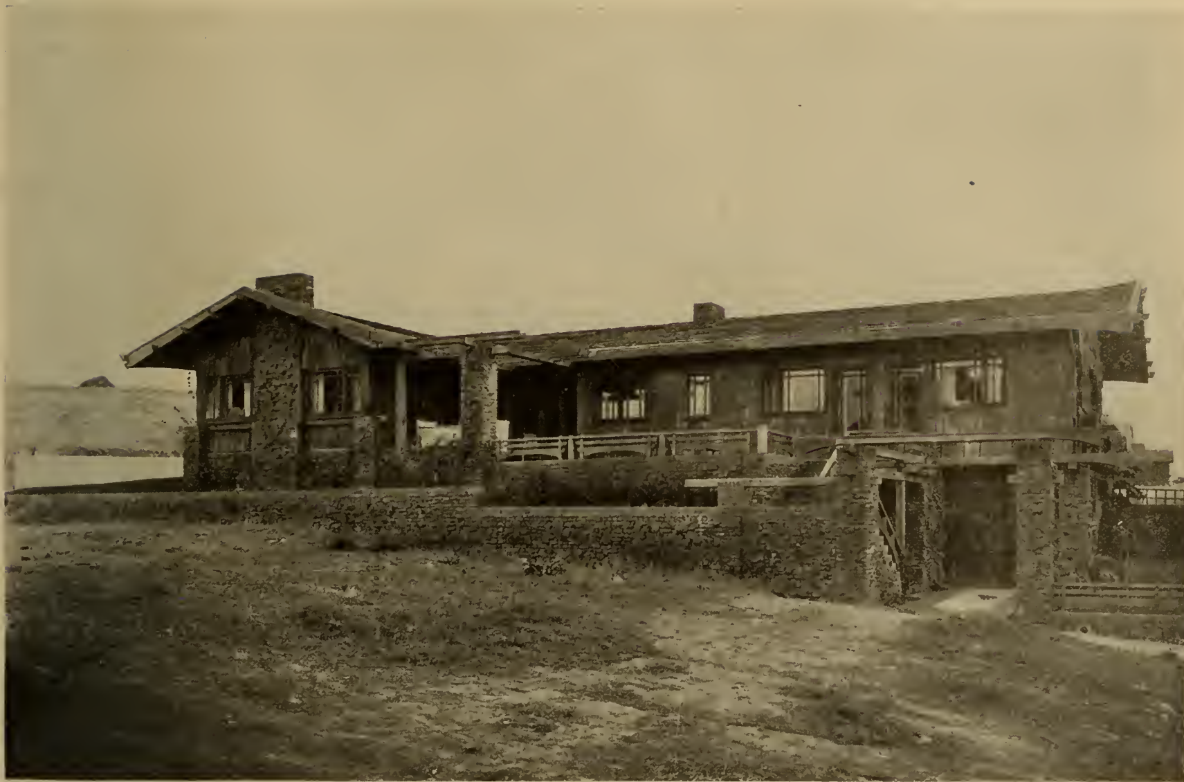
THE LONG LINES OF ROOF AND WALL ARE RESTFUL AND HARMONIOUS WALKER & VAWTER, Architects
