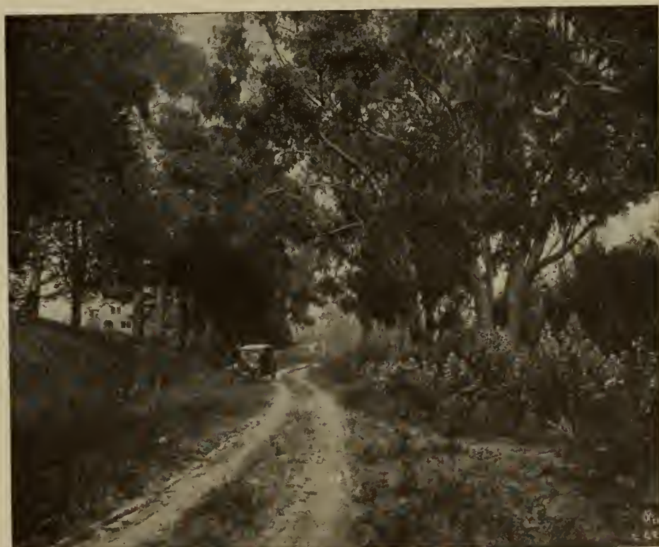
THE PROCESS OF ROAD-MAKING Lakeshore Highlands, Oakland, California
