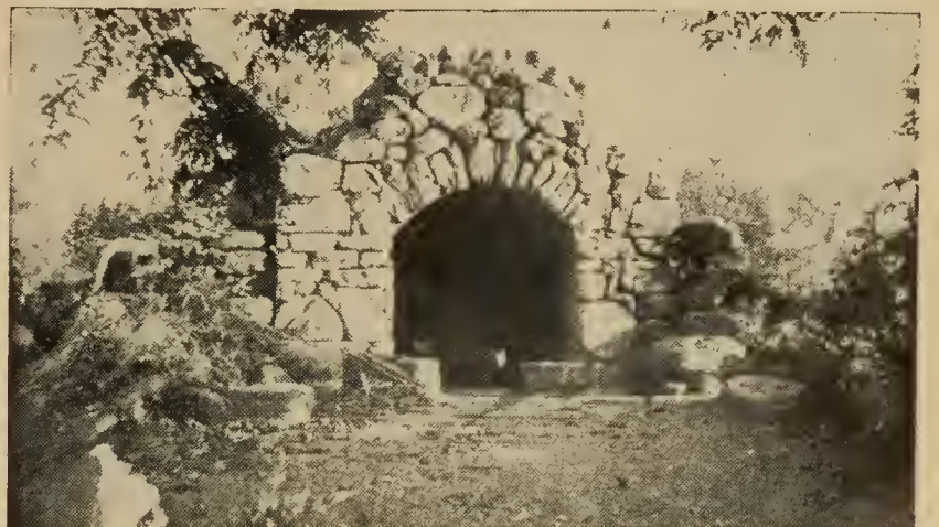
OPEN-AIR FIREPLACE RESIDENCE OF ROBERT S. MOORE ALBERT FARR, ARCHITECT
