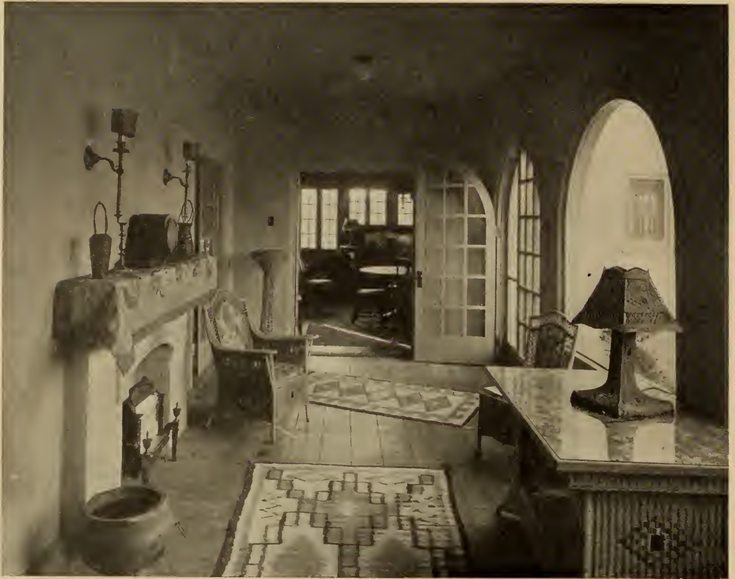
LOGGIA IN MR. VAN CAMP'S HOUSE, LONG BEACH, CALIF.
