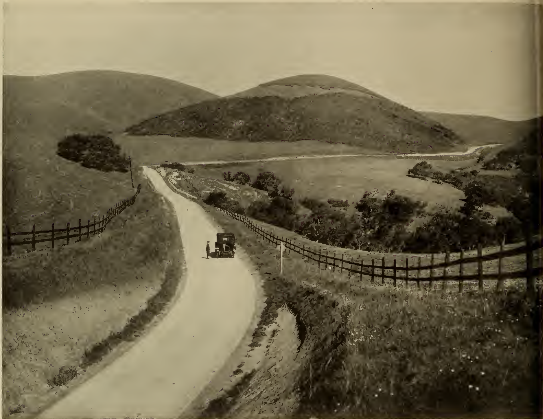
A NAKED, UNPLANTED HIGHWAY, SHOWING SCABS ON THE LANDSCAPE DUE TO CUTS IN GRADING AND LACK OF FOLIAGE ON THE SAN JUAN GRADE.
