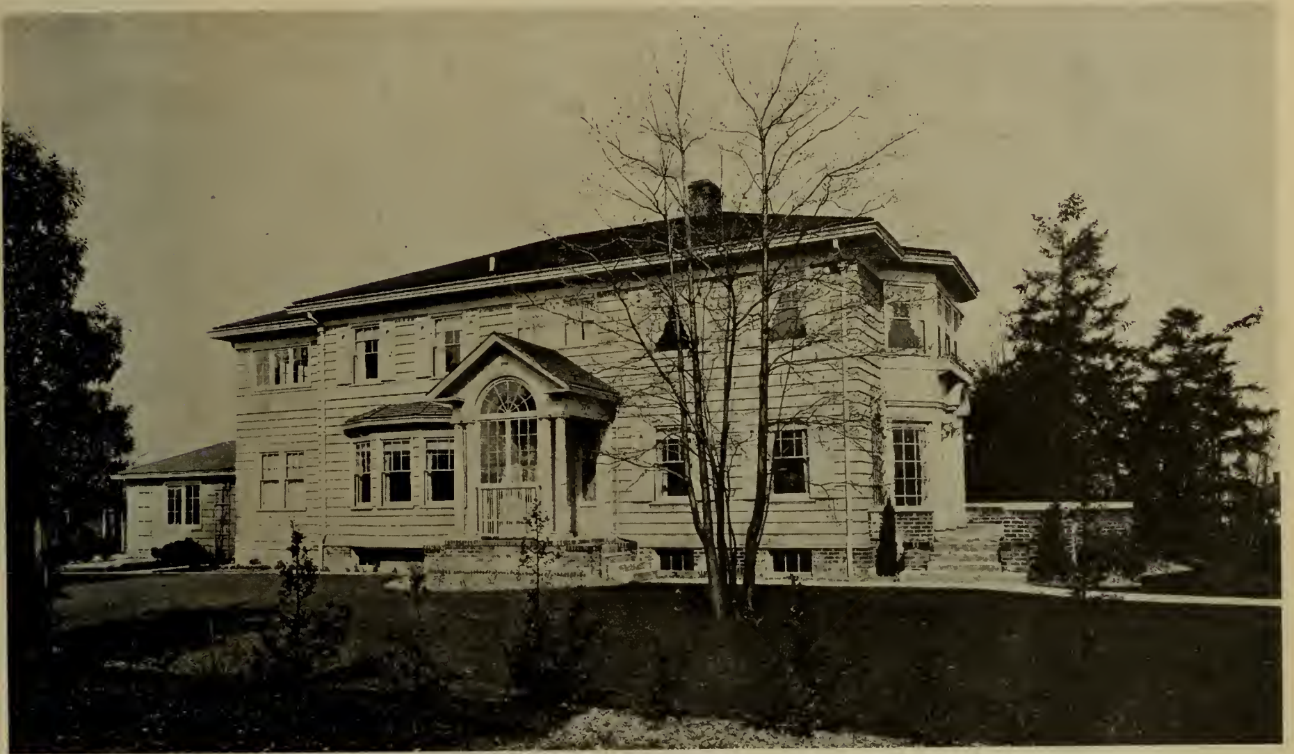
RESIDENCE OF MR. WILLIAM G. JOHN, SEATTLE, WASH. ARTHUR L. LOVELESS, Architect
