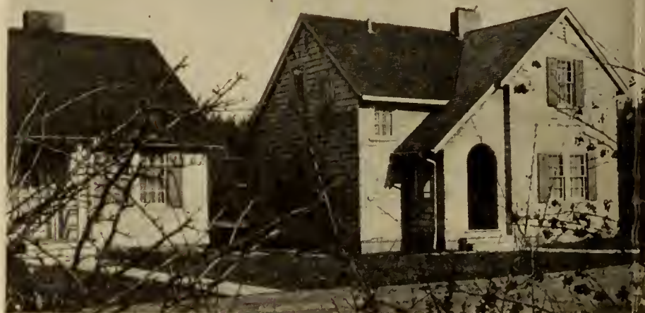
HOUSE No. 204-A, PUGET SOUND NAVY YARD
