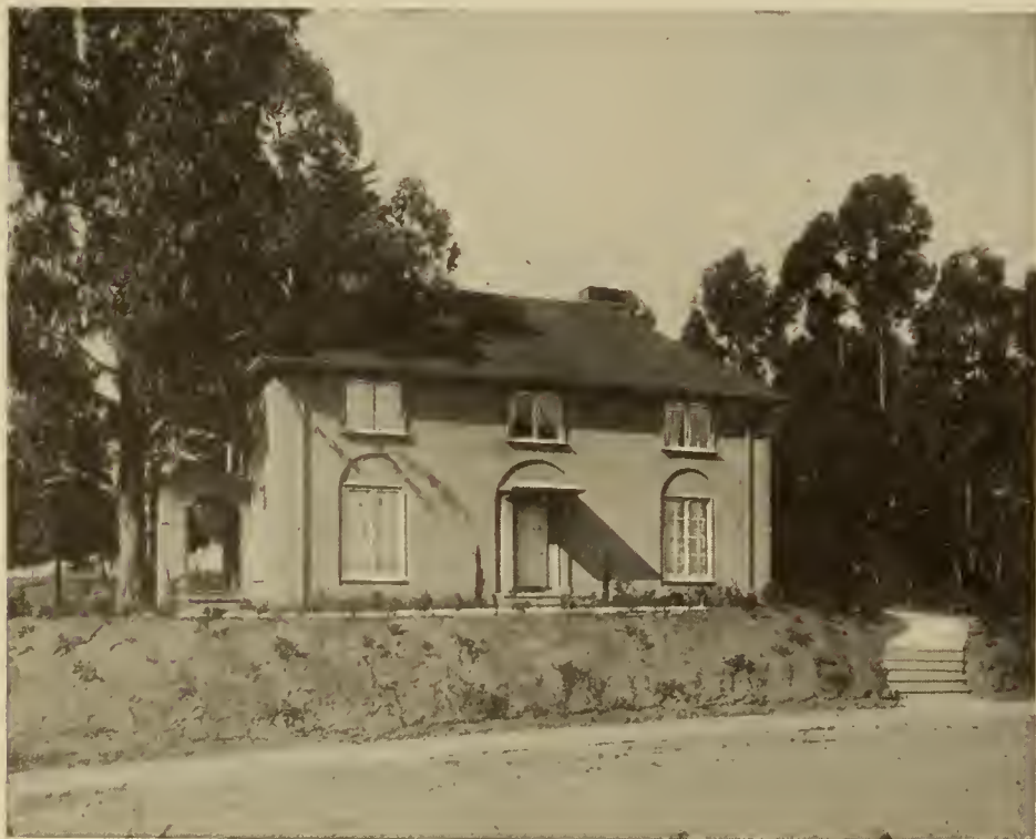
RESIDENCE OF MR. ARTHUR DAVIS Lakeshore Highlands Oakland, California Horace G. Simpson, Architect
