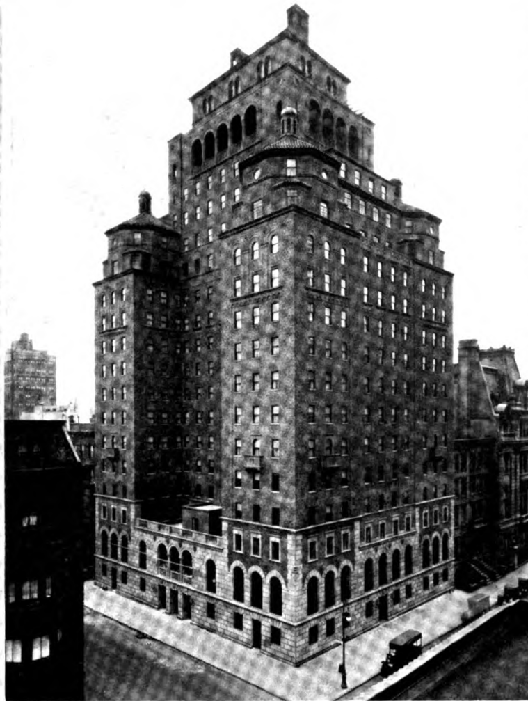
New York Fraternity Clubs Bldg., New York, Murgatroyd & Ogden, Architects Jaros & Baum, Engineers. John C. Williams, Heating Contractor Two 13,000' and one 10,000' Pacific Boilers installed
