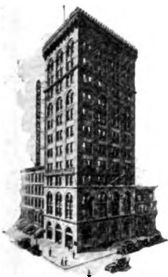
The Old Building
