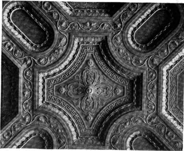
Detail, Ceiling, Board Room, New York Cotton Exchange Donn Barber, Architect
