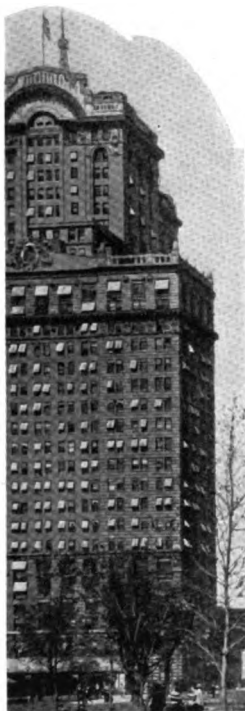
Awnings never beautified any building. They are a constant addition to fire hazard and cost of building maintenance.
