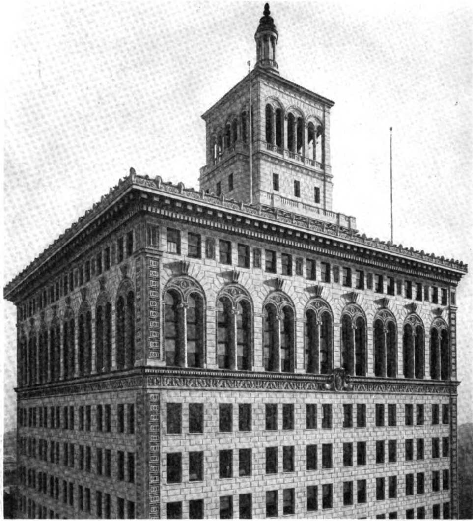
Upper stories of Matson Building, San Francisco, California. Bliss & Faville, Architects. Entirely finished in warm gray matt glazed Terra Cotta with background of ornamental features in blue green.
