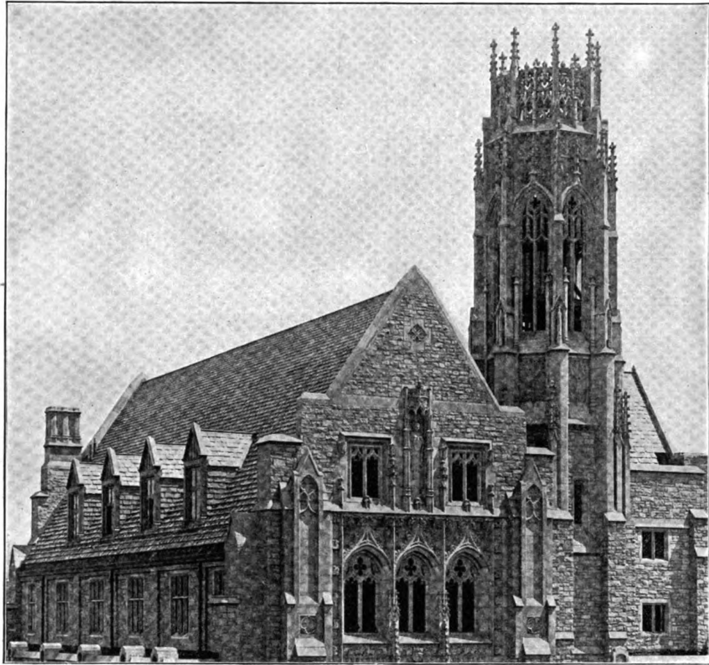
The Roof of the Park Avenue Baptist Church New York
