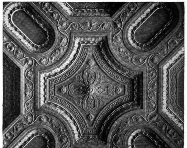
Detail, Ceiling, Board Room, New York Cotton Exchange Donn Barber, Architect
