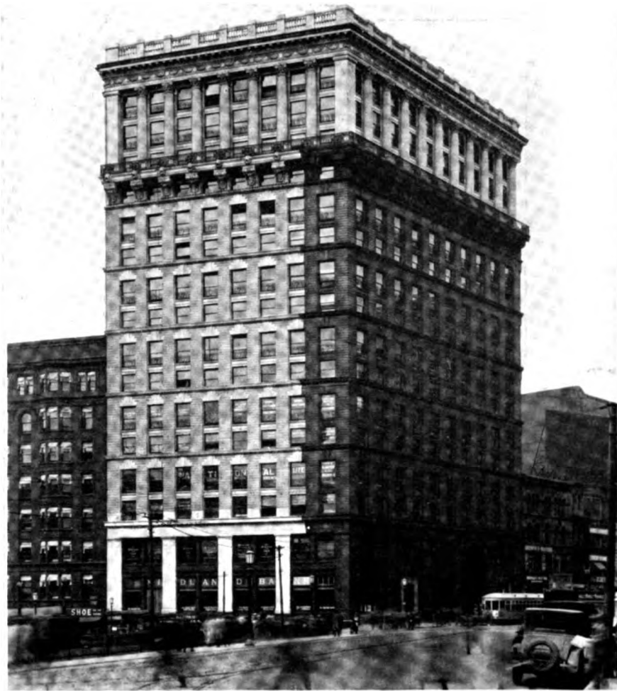
Williamson Building, Cleveland, Ohio. Geo. B. Post & Sons, Architects. Photo showing building in course of cleaning by ordinary washing process.
