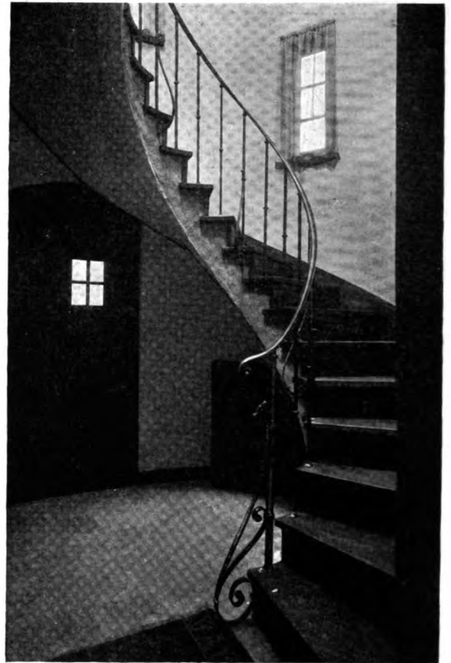
Illustration of hand-wrought iron stair railing and baluster made by us for the Residence of R. M. Brinkerhoff, Strawberry Hill, Stamford, Conn.
