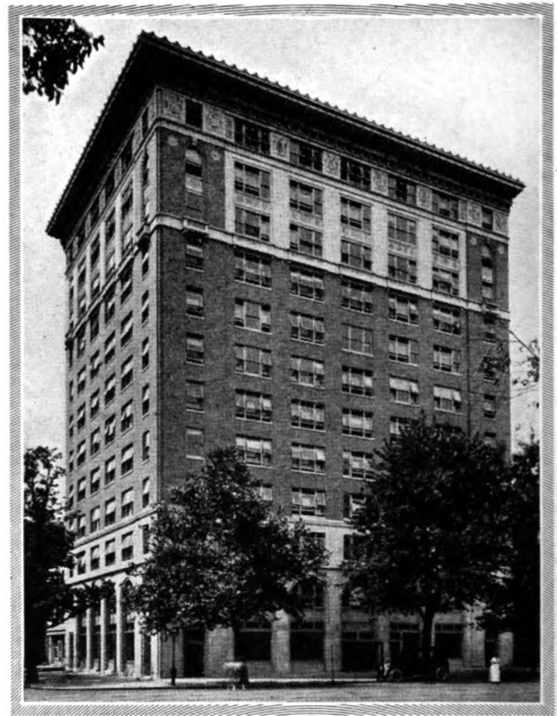
Hurley Wright Building, Washington, D. C. Clarence L. Harding, Architect
