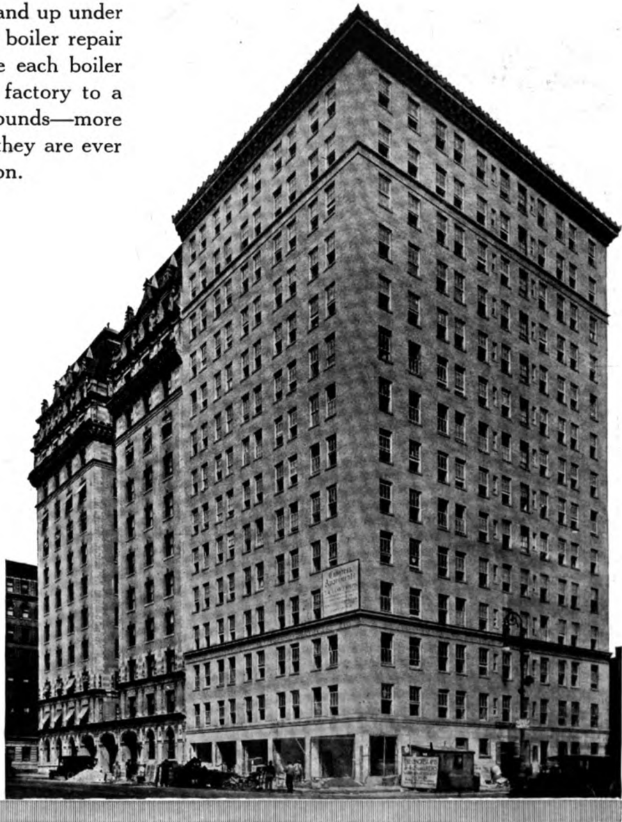
Congress Apartments, N. E. Corner 7th Avenue & 54th Street, New York, N. Y. Marcus Brown, Owner. Geo. F. Pelham, Architect. W. G. Cornell Co., Heating Contractor. Two 15000' Pacific Boilers installed.
