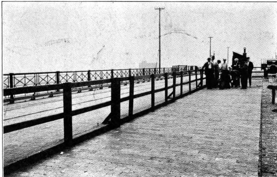
A Section of the Wright Rubber Pavement on Eads Bridge, St. Louis, Mo.
