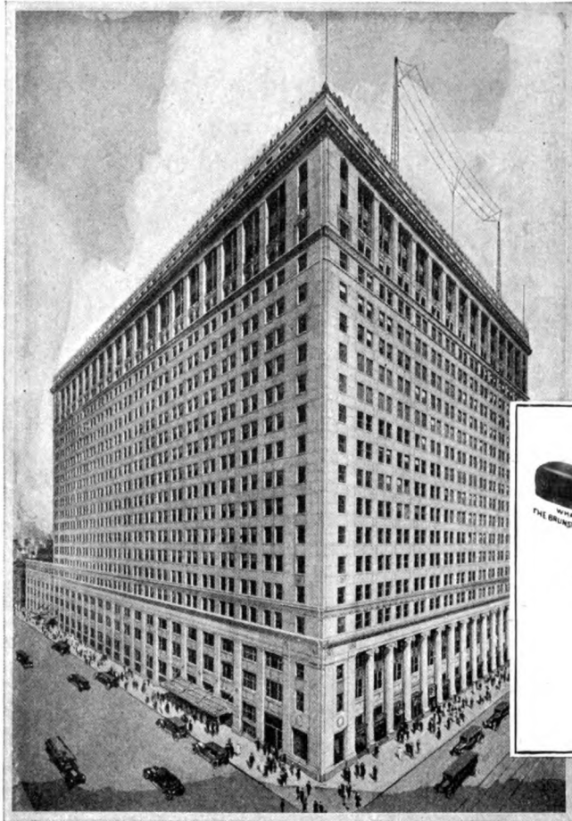
Union Trust Bldg. Cleveland, Ohio Equipped with No. 18-59 Ebony
