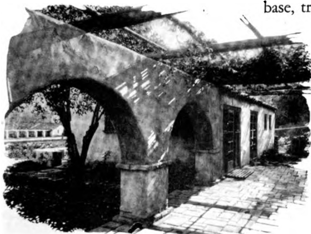
Stucco Finish Coat of "Dias Dorados" made with Atlas White Portland Cement. ARCHITECT Mr. Ray Seldon Price
