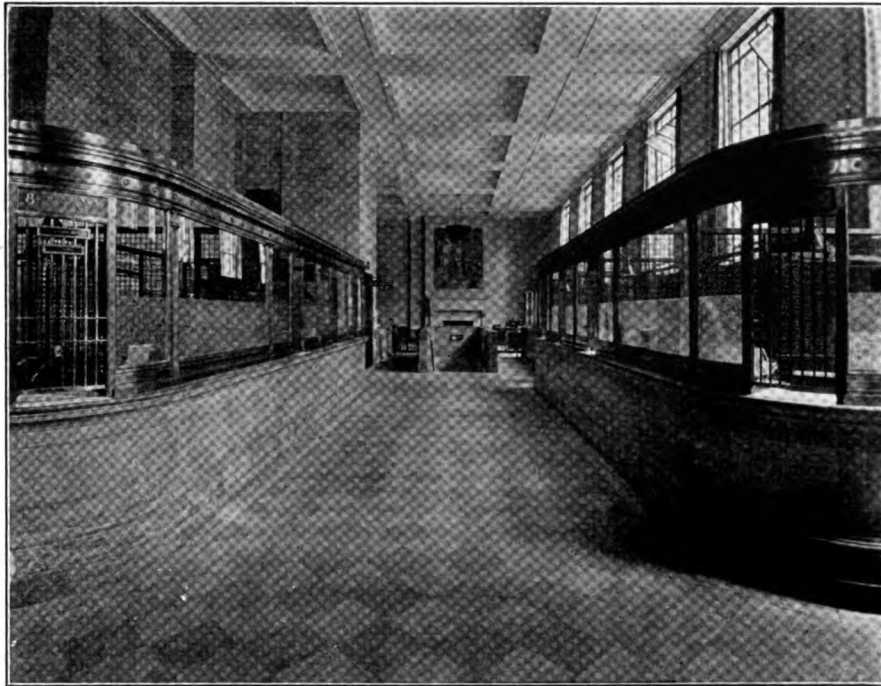
Banking space of Mutual Trust Company, Philadelphia, Pa. Walls to ceiling of Imported T. K. Travertine. Floor of Travertine and T. K. Tennessee Blocks. Bank screen of Yellow Kasota. Heacock & Hokansen, Architects. Glenwood Tile Company, Contractors
