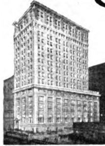
42nd St. and Vanderbilt Ave., New York City Warren & Wilson, Architects Dought P. Robinson & Co., Builders
