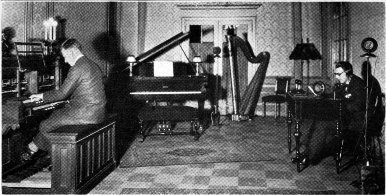
Broadcasting Studio for pipe organ, Lyon & Healy, Chicago, Ill. Acousti-Celotex Type B, decorated, used on ceiling. Type D entirely covers the side walls, the open spaces into the organ chambers being covered with stretched silk panels. This is stenciled in an Adam pattern. The only broadcasting studio in the world which efficiently broadcasts pipe organ music
