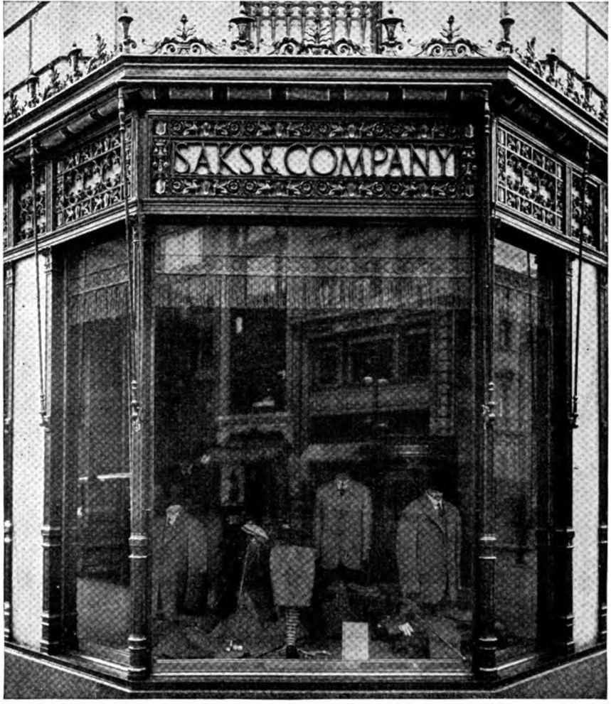
THROUGH THE USE OF ANACONDA ARCHITECTURAL BRONZE EXTRUDED SHAPES, MESSRS. STARRETT AND VAN VLECK SECURED FAITHFUL REPRODUCTIONS OF THEIR DESIGNS IN THE ENTRANCES AND DISPLAY WINDOWS OF SAKS & COMPANY'S NEW FIFTH AVE. STORE, NEW YORK.
