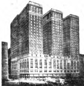
Palmer House, Chicago, Ill. Richard & Rorke, Architects Thompson-Harrott Co., Builders
