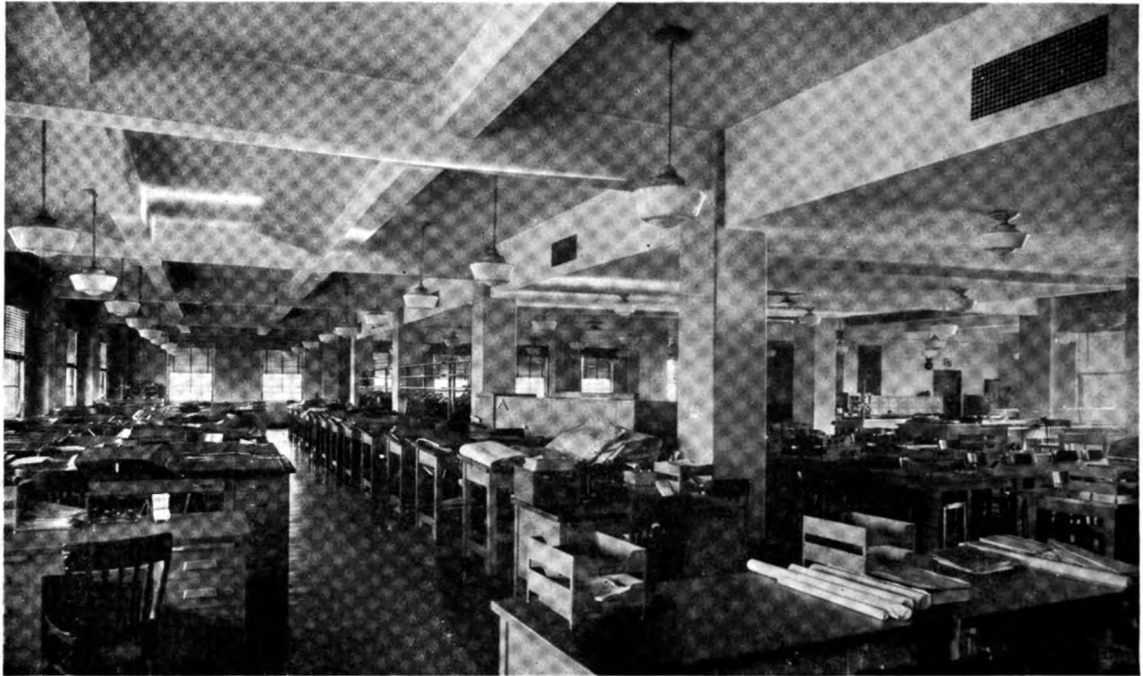
TYPICAL OFFICE FLOOR, BROOKLYN EDISON CO., BROOKLYN, N. Y. McKenzie, Voorhees & Gmelin, Architects S. G. Hull & Son, Painting Contractor
