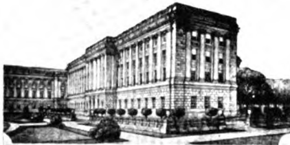
West Virginia State Capitol, Office Building No. 1, Charleston, W. Va. Chas. Gilbert, Architect George A. Fuller Co., Builders
