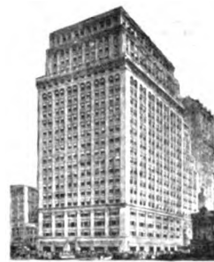
40th Street and Broadway, New York City Marrett & Lee, Architects S. S. Roth & Sons, Builders
