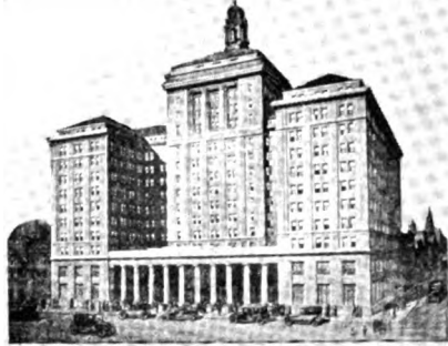
Municipal Building, Brooklyn, N. Y. McKean, Vanhook & Gmelin, Architects Caldwell-Wiggin Company, Builders
