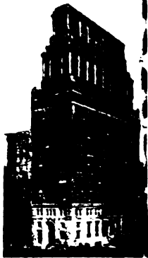
Bank of America, New York City Trembridge & Livingston, Architects Chas. F. White, Inc., Builders
