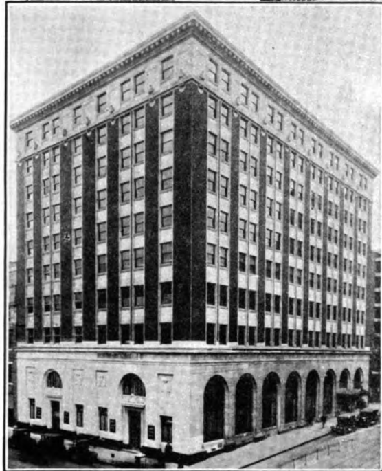
First National Bank Bldg., Tulsa, Okla. Architects: Rush, Endicott & Rush. Jobber: Kellogg MacKay Co. Plumber: Dunbar Plbg. & Htg. Co. Equipped with No. 21-9 Seats
