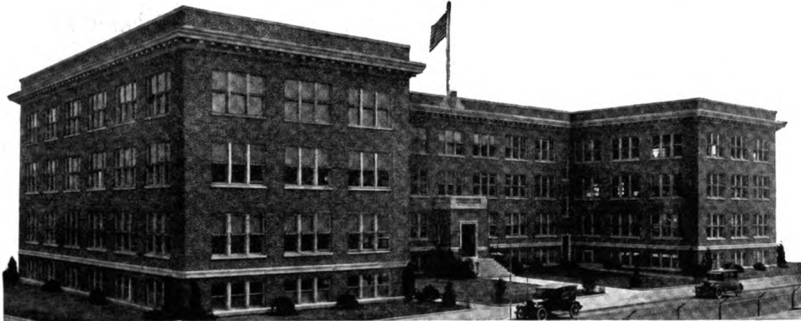
New office building of Jeffrey Manufacturing Co., Columbus, Ohio, with Lupton Double Hung Windows throughout. Stone & Webster, Architects and Contractors
