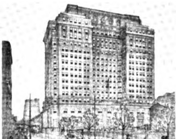
Insurance Company of North America Building, Philadelphia, Pa. Simpson & Fox, Architects How & Whitt, Builders
