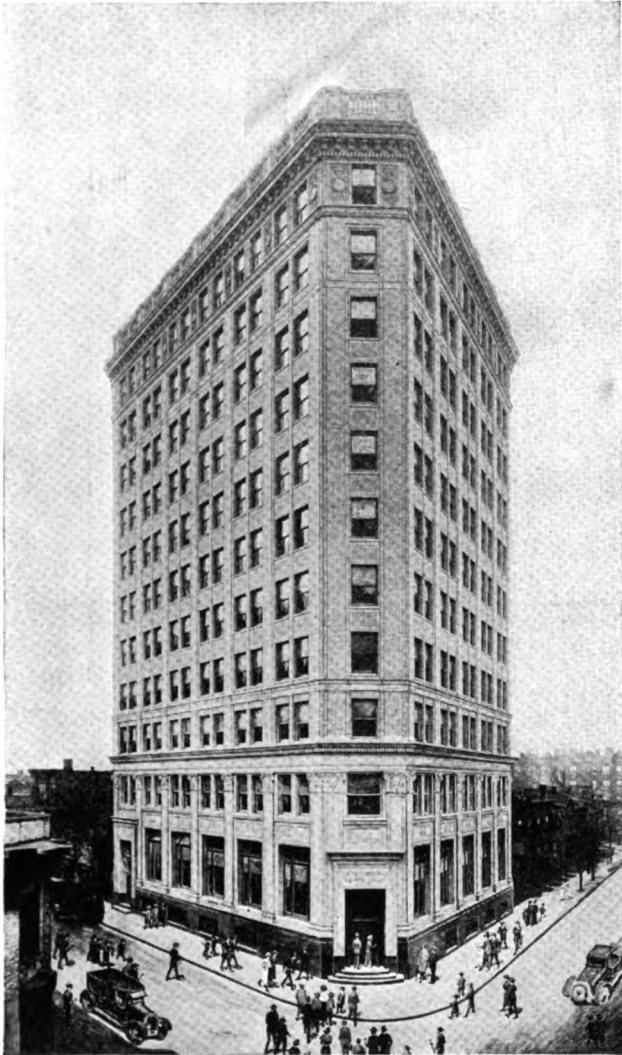
TRUST COMPANY OF NEW JERSEY BLDG., JERSEY CITY, N. J. Clinton & Russell, Architects
