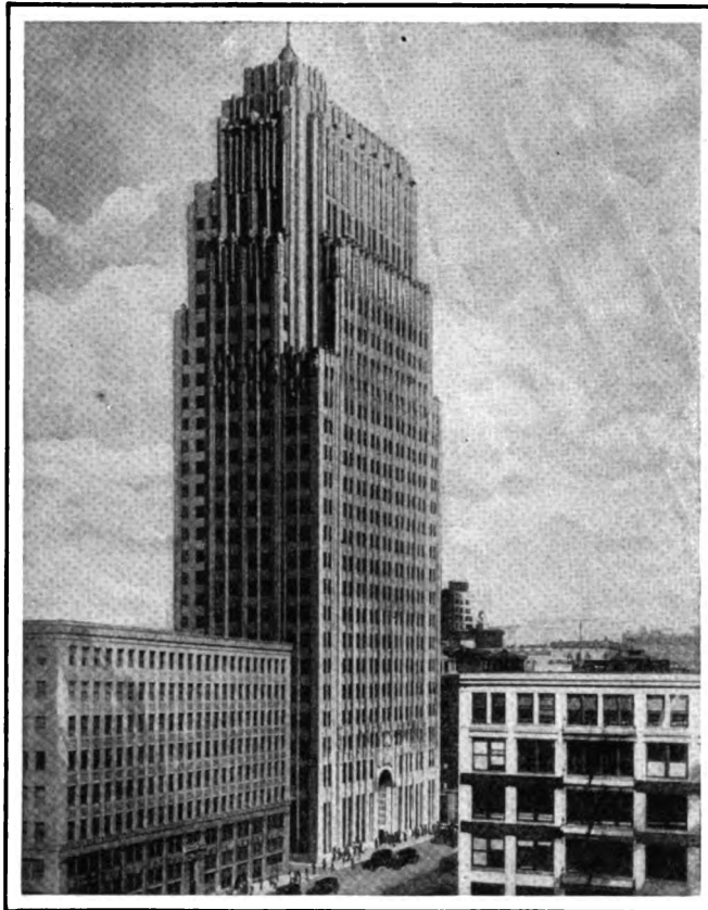
The new Pacific Telephone & Telegraph Building, San Francisco. Crane plumbing materials are installed throughout. J. R. Miller, T. L. Pfueger, and A. A. Cantin, Associated Architects. Atkins & Parker, Mechanical Engineers. Lindgren & Swinerton, Builders. Alexander Coleman, Plumbing Contractor.
