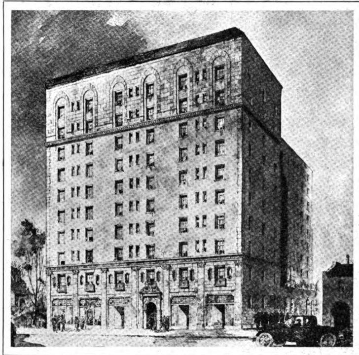
HOLLYWOOD PLAZA Hotel, Hollywood, Cal.: Walker and Eisen, Los Angeles, Architects; N. O. Nelson Mfg. Co., Los Angeles, Plumbing Jobbers; Arthur Hess Corporation, Los Angeles, Plumbers
