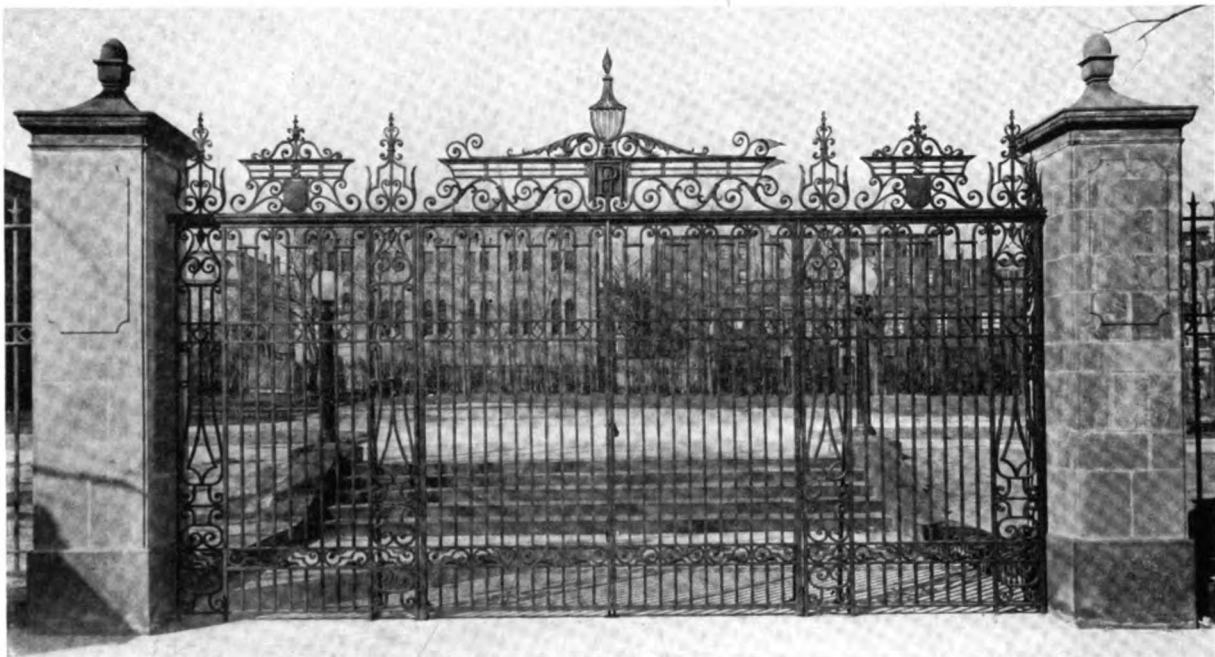
WROUGHT IRON PARK ENTRANCE (SIZE 20' x 10'), EXECUTED FOR THE PRATT INSTITUTE, BROOKLYN John Mead Howells, Architect
