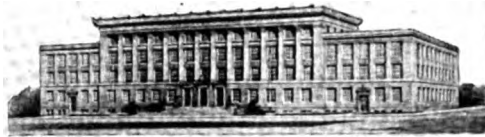
Girls' Catholic High School, Brooklyn, N. Y. Robert J. Egan, Architect W. L. and G. H. O'Brien, Builders
