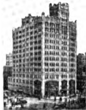
Metropolitan Building, Detroit, Mich. Wason & Ellington, Architects Walbridge-Aldinger Co., Builders
