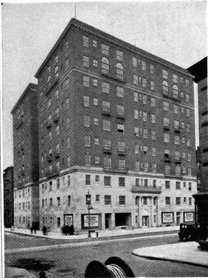
PAULDING APARTMENTS · NEW YORK CITY Louis Eden, Sanitary Engineer Tarcho Bros., Plumbing Contractors
