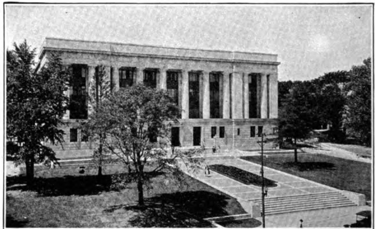
Kansas City Life Insurance Bldg., Kansas City, Mo. Architects: Wight & Wight. Jobber: U. S. Water & Steam Supply Co. Plumber: McMahon Plbg. & Htg. Co. Equipped with No. 18-59 Seats
