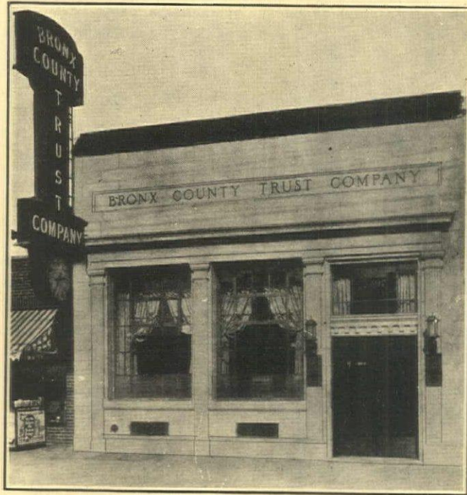
Bronx County Trust Company, Tremont Ave. and Eastern Blvd., New York City. William M. Husson, Architect. Sash by David Lupton's Sons Co.
