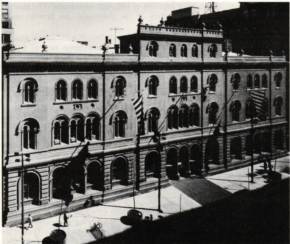
To restore the facade of the New York Public Theater, Mesick/Cohen/Waite used newly quarried sandstone and a team of expert stone carvers to replace deteriorated and missing brownstone elements.
