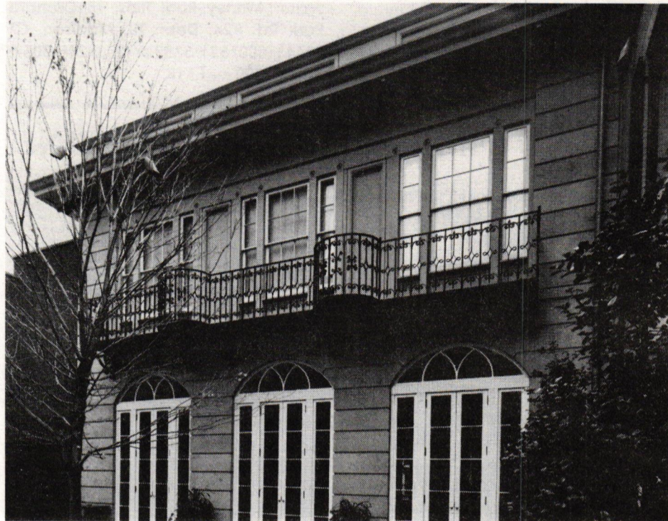
Besides restoring the historic sections of Blair House in Washington, D.C., Mesick/Cohen/Waite designed this new addition that serves as the President's accommodations for official state guests.
