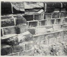
When historic brickwork is repointed with hard portland-cement mortar, serious spalling and brick deterioration can result, as shown in this photo. GENLIME GROUP, L.P., has reintroduced prepackaged lime putty, making it simple to create the soft lime mortars that are best for repointing historic brick masonry. Write in No. 450
