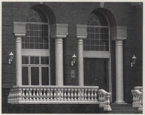
Balustrades and columns from ROYAL CORINTHIAN are made from a synthetic polymer stone that eliminates rot and is lighter than cast stone. Write in No. 76
