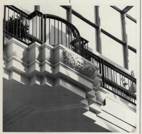
ARCHITECTURAL REPRODUCTIONS, INC., is experienced in simulating terra cotta in a variety of materials, including glass-reinforced gypsum, as shown in this photo. This gargoyle balcony facing was molded in gypsum for the Rouse Company's Pioneer Place project in Portland, Oregon. Write in No. 6130
