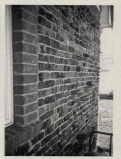
THE BRICKYARD, INC., recovered these authentic antique clinker bricks from an abandoned brickyard in Missouri. Clinkers come in colors ranging from orange-red to purplish black. Write in No. 3960
