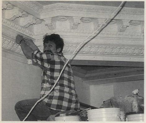
SALDARINI & PUCCI did all the ornamental plasterwork for this high-end residence in Long Branch, New Jersey. The plasterer, perched on a catwalk in the 45-ft.high octagonal entryway, is concealing fluorescent lighting in the center of this complex frieze. The company has a large inventory of plaster molds in classic styles. *Write in No. 24*
