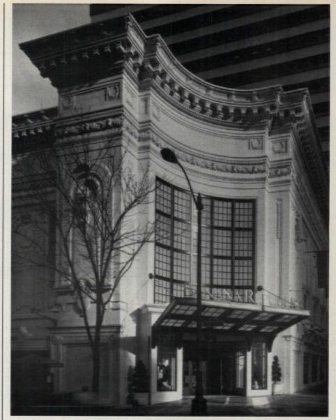
The terra-cotta replacements for Seattle's Coliseum Theater renovation utilized both individual precast concrete units and larger moldings of multiple block assemblies using glassfiber-reinforced thinshell techniques.
