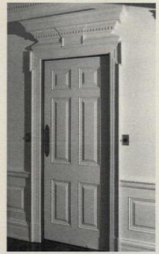
AMERICAN CUSTOM MILLWORK panels, dentils, and egg-and-dart moldings are some of the molded wood elements combined on this classic doorway. Write in No. 6780
