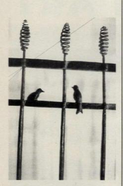
This forged-iron entrance gate was fabricated for a commercial site by KAVIAR FORGE. The top ornament is forged in a reverse taper, and the castiron birds include relief details. Write in No. 9840
