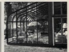
This house is illuminated by the "SOL-AIRIUM," an UNDER GLASS MFG. CORP. creation. The sun space offers an insulating air barrier sandwiched between two pieces of safety glass, and a ventilating sash that can be thermostatically controlled. The solarium is available in white or bronze finish. Write in No. 3510
