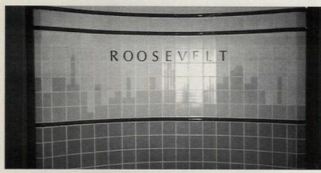
The "Roosevelt" subway station of the Chicago Transit Authority uses ELGIN-BUTLER BRICK COMPANY's 8-X-8-in. glazed bricks, which are fire-resistant, moisture-impervious, color-fast, and virtually maintenance-free. The "Roosevelt" letters were glazed on, and the skyline reflection of Chicago was created by stenciling one color upon another. Write in No. 36
