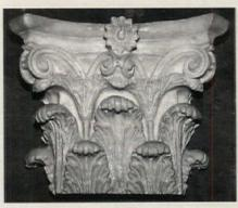
This fiberglass-reinforced, polymermodified, concrete Corinthian capital was cast as part of a larger restoration project by FREEDMAN STUDIOS. Write in No. 6390
