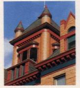
■ The Romanesque-style Monroe County Courthouse, built in 1896, had its slate roof replaced with asbestos shingles in 1929, at which time its original gutter was also covered over. More than 60 years later, the asbestos had deteriorated and lichen was covering much of the roof. Weak flashing, a dearth of gutters, and decades of freeze-thaw cycles had caused water damage to the sandstone walls.
