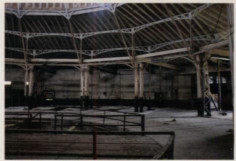
This view of the roundhouse shows the deceptively delicate cast-iron elements that compose its structural framework.
