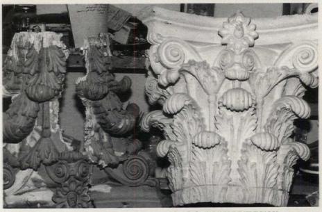
When major water damage destroyed the capital at left, RORY BRENNAN/ PRESERVATION PLASTERING was called in to cast and create a replacement element, right. *Write in No. 2980*
