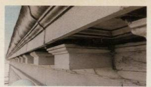
THIS CLOSE SHOT REVEALS THE DISPLACEMENT OF THE CORNICE FROM THE MODILLION UNITS; THE ORIGINAL JOINT WIDTH WAS ABOUT ONE THIRD OF THE GAP SEEN HERE.
