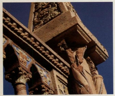
a \$4.5 million restoration plan. While other areas were also in need of conservation, including roof-replacement work and work on the leaded-glass windows, the failing terra cotta was considered the single-most significant threat to the building and to passersby.
