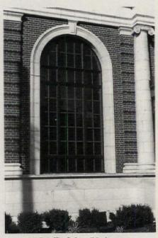
ARCHITECTURAL REPRODUCTIONS replicated the original limestone columns and cornice of this 1919 building using GFRC for the columns and sheetmetal for the cornice; various decorative elements were reproduced with cast aluminum and fiberglass parts. *Write in No. 6130*
