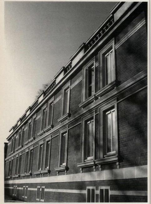
CAPE STONEWORKS utilized C.N.C. profile saws and traditional hand-carving skills to fabricate the Indiana limestone detailing on this classical building. Write in No. 449
