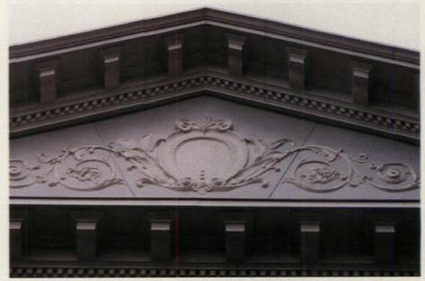
The subsequent FRP pattern was sculpturally recreated in modeling clay, in a 30-ft.long by 7-ft.-high flat panel that was then cast in a hard mold.
