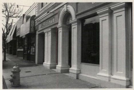
Fiberglass columns fabricated by SEAL REINFORCED FIBERGLASS replicated the original terra-cotta columns of this storefront business. *Write in No. 4620*
