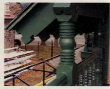
Consolidation and epoxy patching materials were used on the exterior wood at the Undine boathouse, primarily on larger members and where exposed end grain conditions increased susceptibility to rotting. The turned members — newel posts, balcony railings and porch columns — had sharp edges as a result of Furness's fondness for bold geometric form. Much of this detail had become badly checked or was missing. Where necessary, new turnings were made from laminated mahogany.
