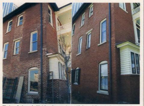
Tinting of mismatched brick and mortar is provided on a full-service basis by Nawkaw Corp. They use a water-based stain, which is mixed on site by Nawkaw personnel and can be thinned and continually color-adjusted as needed during the course of the job. Write in No. 206
