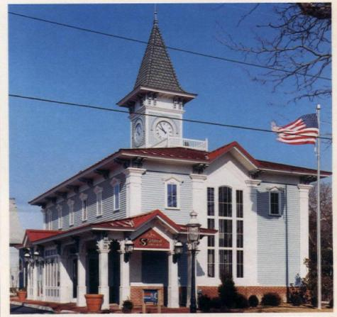
AFTER RESTORATION, THE TURRETS WEAR THE SAME ROOFING AS THE REST OF THE COURTHOUSE: SLATE, THE MATERIAL INTENDED WHEN THE STRUCTURE WAS BUILT IN 1896. Architecture Network, Inc., removed the asbestos shingles and the roof flare that covered the original built-in gutter. The roof was then covered with contin-
