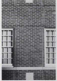
The waterstruck-brick method used by VERMONT BRICK MFG. involves water and sand in the molding process, resulting in a uniquely textured brick suitable for renovation and restoration, as well as new construction with a traditional look. Write in No. 765
