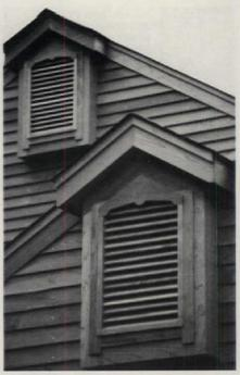
Country-style redwood louvers from AWSCO MILLWORK have a square inside jamb, S4S 3/4 exterior casing, front trim boards, pitched topboard, and scalloped board. They are available as "Rain-Gard Baffle" or "Facade Construction" units. Write in No. 5064
