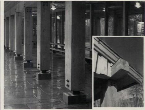
The architects of the visitor center at Minnesota's Gooseberry Falls State Park used DULUTH TIMBER CO. Douglas fir posts and beams, with the natural materials complementing the contemporary design. Write in No. 112
