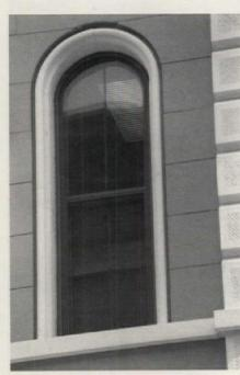
The 4th and Plum building in Cincinnati, Ohio, utilizes ALLIED WINDOW HOL-B Historic-One-Lite storm windows, designed for exterior installation, with trim lines that are practically invisible, and window projections of just 3/8 in. Write in No. 690
