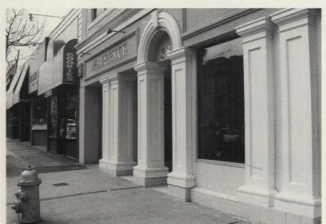
SEAL REINFORCED FIBERGLASS replicated pilasters in fiberglass for this storefront, substituting for original terra-cotta units. Write in No. 4620
