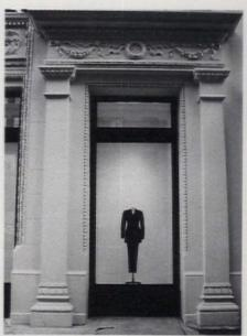
ESSEX WORKS re-created and replaced the ornamentation of this commercial storefront with pre-cast concrete and GFRC. Write in No. 7200
