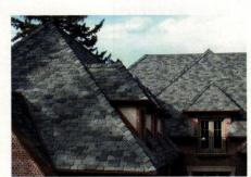
This roof in Denver, CO, is comprised of a three-color, random-width, domestic slate blend from Source Products Group.
