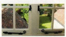
The design of this malleable-iron window hardware, hand cast by Kirkpatrick, was based on patterns that date back to 1855.
