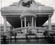
Cast-polymer/stone columns and balusters from Royal Corinthian were used to create this entryway.
