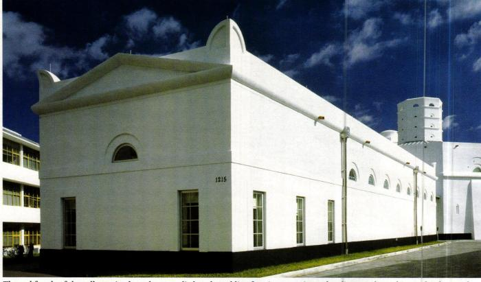
The end façade of the gallery wing has a large applied ovolo molding forming a cornice and pediment. Above this, on the short end wall, are abstracted antefix-like corner details. Beyond is one of the International Style former dormitories housing the School of Architecture offices and studios.
