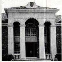
Stonex's line of cast-stone architectural elements includes columns and pilasters.
