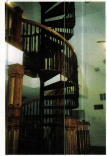
Goddard Mfg. fabricates steel, wood and combination steel/wood spiral stairs.
