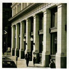
The original limestone columns of this 1919 building were replicated in GFRC by Architectural Reproductions.
