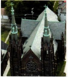
The Durable Slate Co. repaired the slate roof and replaced copper valleys, the ridge roll and the copper work at the base of the steeples of this century-old church and rectory in Ohio.
