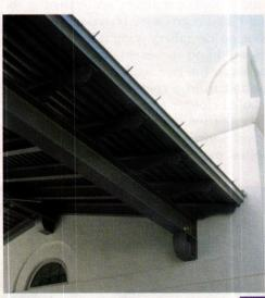
Above: The gallery wing is separated from the octagon by a delicately-scaled, gable-roofed breezeway, in which the steel roof structure is exposed to exterior view. The overhanging webs of the wide-flange steel rafters are shaped to resemble timber rafter tails. *Photo: Steven W. Semes*
