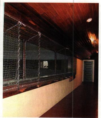
The corridors' tongue-and-groove ceilings have been brought back to their original high-gloss varnish. Sound insulation has been installed above them, where the original builders had stuffed bagfuls of sawdust.
