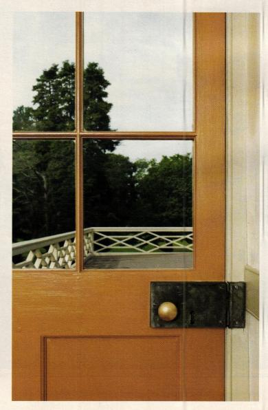
This hand-forged two-bolt iron rim lock leads from a bedroom to the second floor roof of the 1809 wing; all brass knobs were provided by another manufacturer.
