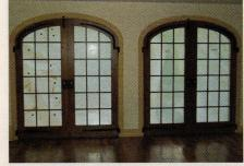
These eliptical arched-top french doors with double pane insulated glass were fabricated by Illingworth Millwork.
