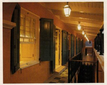
The upper porch of the building opens into the courtyard and into the building. Taylor reintroduced the masonry anchoring elements removed in the 1970s. The windows feature exterior and interior shutters.
