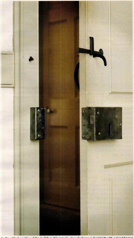
In the oldest section of the building, this interior door features a dead bolt with a hand-forged thumb latch. The metal was left unfinished for an aged appearance.
