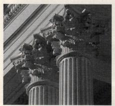
DeAngelis Iron Work, Inc. supplied and installed 12 cast-iron capitals for the exterior restoration of the Massachusetts State House.
