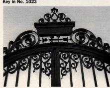
gate with hand-forged scrolls for a project at Harvard Yard in Cambridge, MA.
