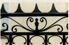
This detail shows the restoration work of Fine Architectural Metalsmiths on a gate featuring a sawtooth "loafer's rail" and typical Vitruvian scrollwork.
