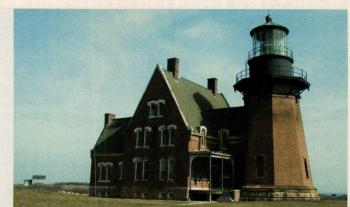
In 1993, the Southeast Lighthouse was hauled away from an eroding cliff, and then its nonprofit owners fundraised for a few years to solve structural and cosmetic problems. Porch gingerbread was missing, chimneys truncated, tower windows boarded up, and granite coping failing. Photo: courtesy of Dr. Gerald F. Abbott, Southeast Lighthouse Foundation
