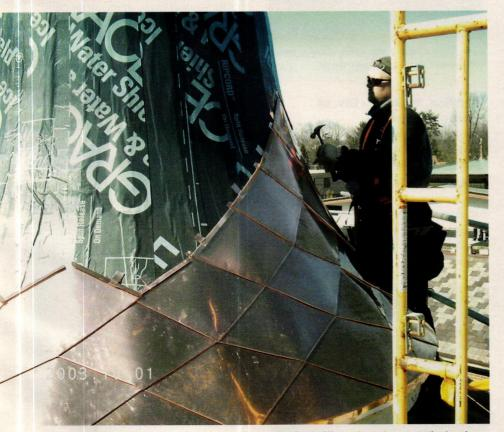
Each row of the diamond-patterned copper panels is sized differently and was meticulously measured and cut in a basement workshop. During installation only three panels were resized onsite with hand tools while the rest snapped on with ease.
