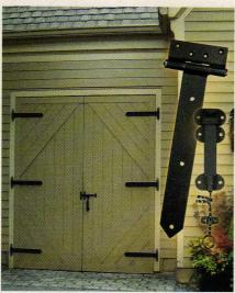
Heavy-duty hinges, latches and handles from Richards-Wilcox were used on this traditionally styled carriage house door.
