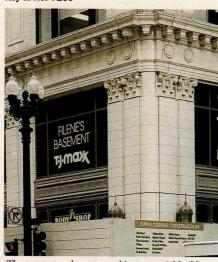
The terra-cotta elements on this commercial building in Chicago were replicated with GFRC elements with technology provided by Ball Consulting.
