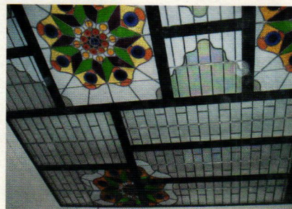
Based on a window by Gaudi, this medallion-design skylight by Michael Davis Stained Glass measures 30x10 ft.
