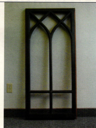
This Kalamein bronze window was fabricated by Heather & Little.
