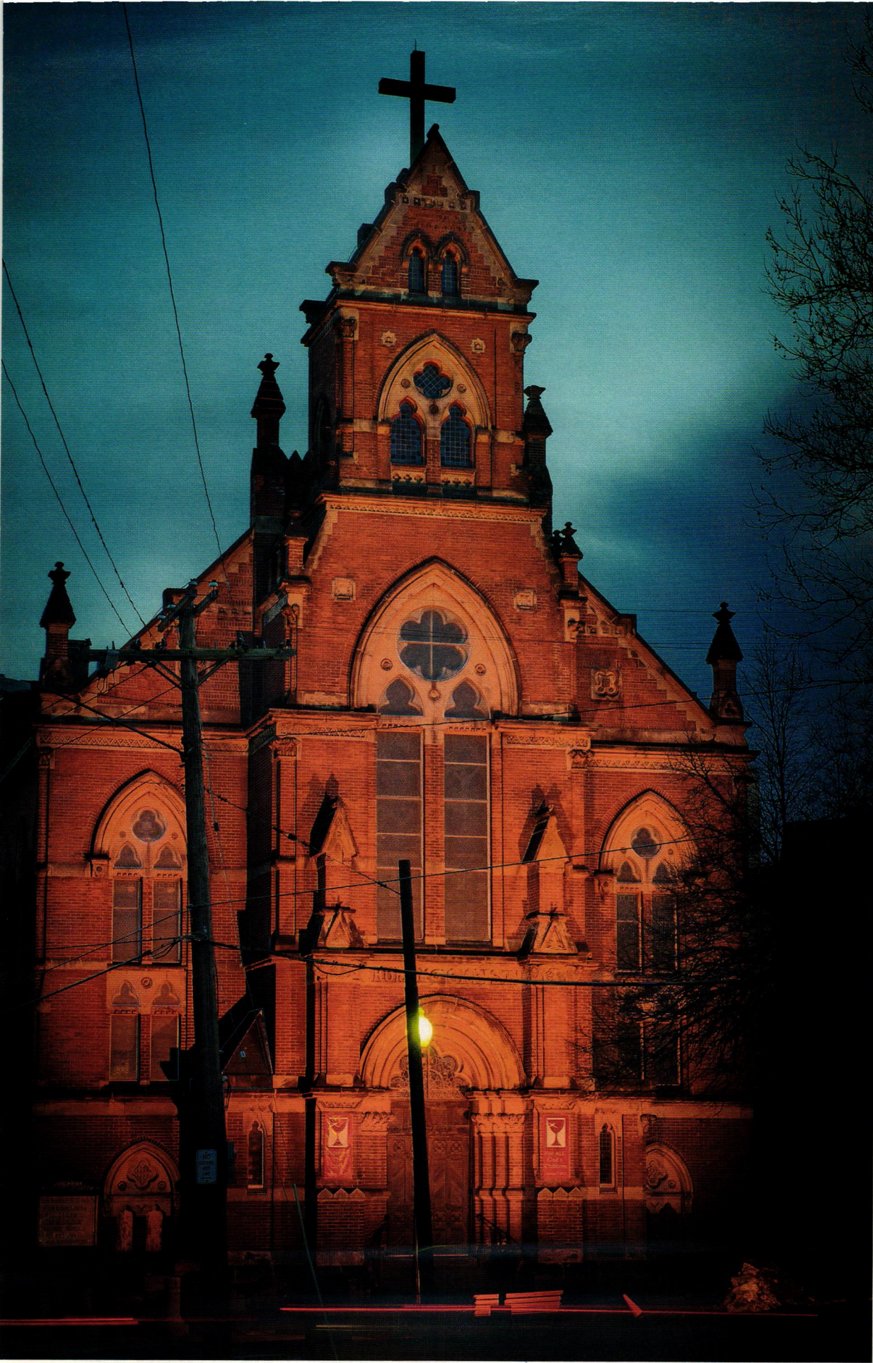
Franklin Circle Christian Church (1874) in Cleveland's Ohio City neighborhood is one of the best examples of High Victorian Gothic architecture in the city. The towers were repaired and illuminated through a $35,000 grant from Cleveland Restoration Society in 2012. Photo: Greg Hildebrandt
