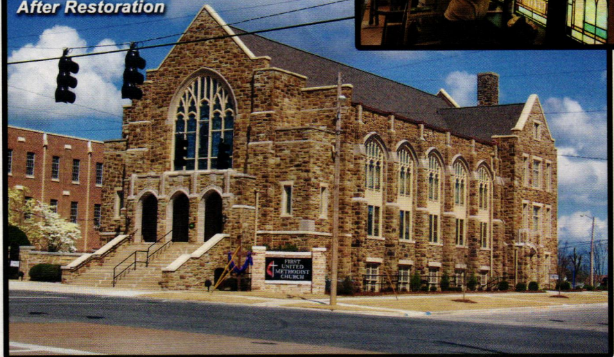
Before and after photos of the F4 tornado damage to the First United Methodist Church of Cullman, Alabama restored by Bovard Studio Inc
