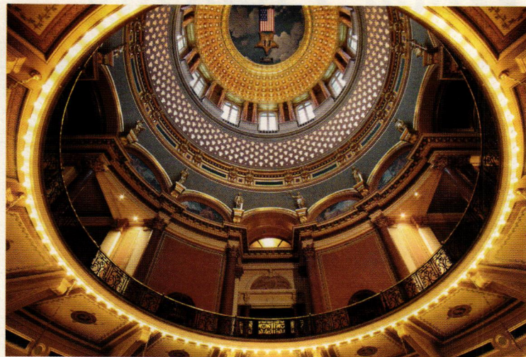
EverGreene restored the interior and exterior of the Iowa State Capitol dome in Des Moines, IA; work included paint analysis, replicated historic finishes, new application of aluminium leaf, replication of the sky mural and restored scagliola columns.
