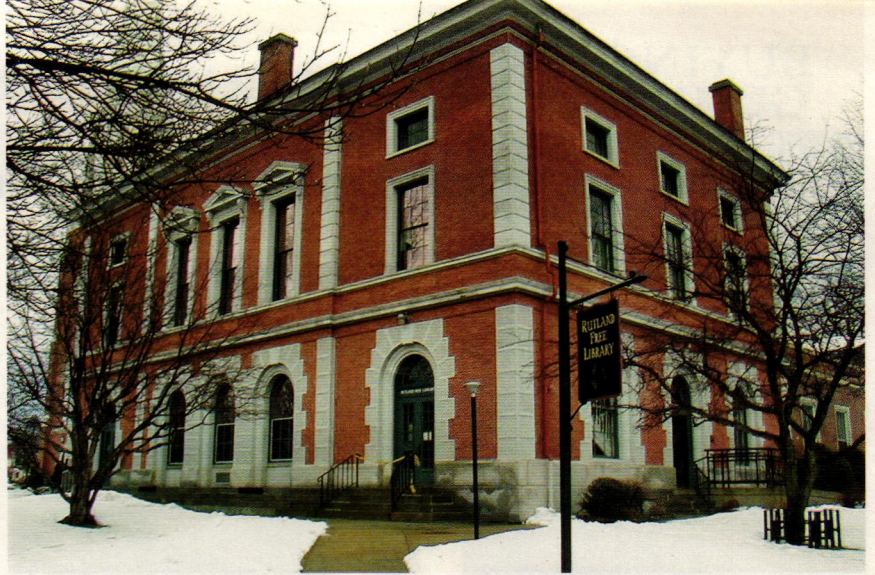
Innerglass Window Systems supplied interior glass storm windows for this historic building.
