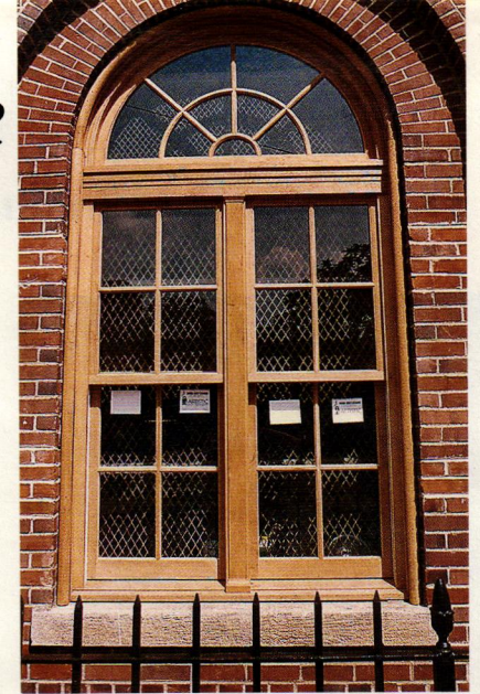
This double-hung window unit with a fixed-arch fan was constructed by Artistic Doors & Windows with mortise-and-tenon joinery.
