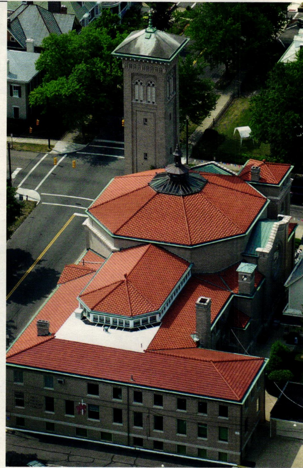
The Durable Slate Co. supplied the tile for the roof of this historic building.
