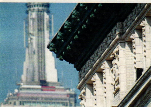
This ornate cornice was fabricated by Gotham Metalworks for an historic building.
