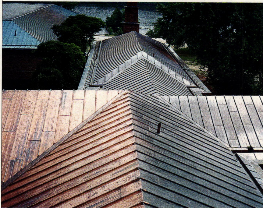
NIKO Contracting Co., Inc. installed this batten-seam and flat-lock copper roof.
