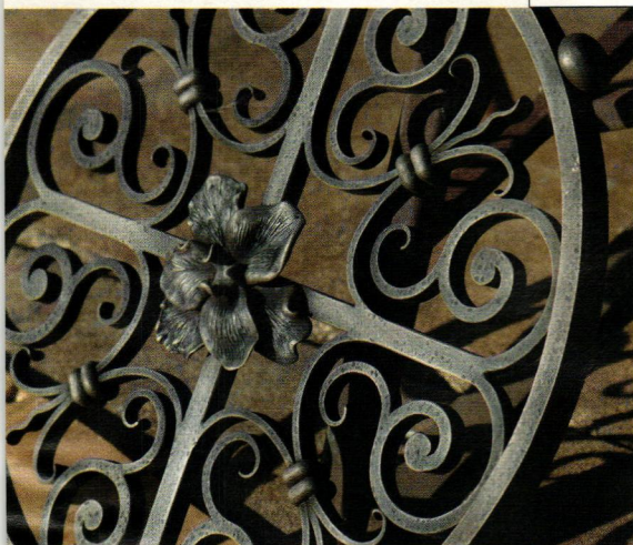
Designed by Curtis and Windham Architects, this forged-bronze grille was fabricated by Wiemann Metalcraft.
