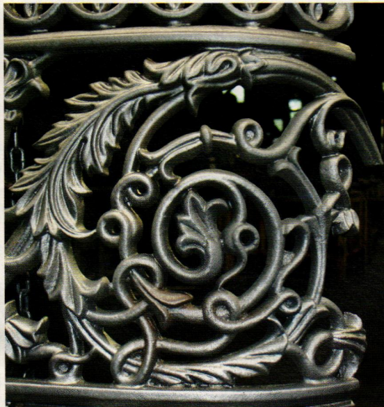
This curved section of fence was cast by O. K. Foundry to match the curbing of the Palmer fence at Hollywood Cemetery in Richmond, VA.
