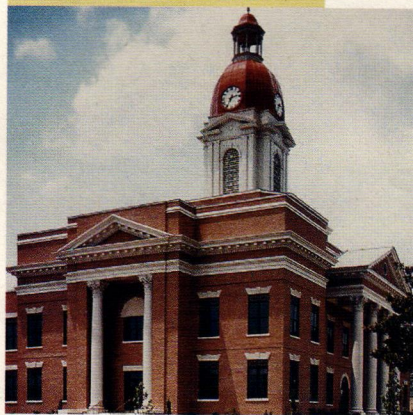
This aluminum cupola, with a 6-ft.-dia. clock and aluminum cornice, was created for the Worth County Courthouse in Sylvester, GA, by Campbellville Industries.
