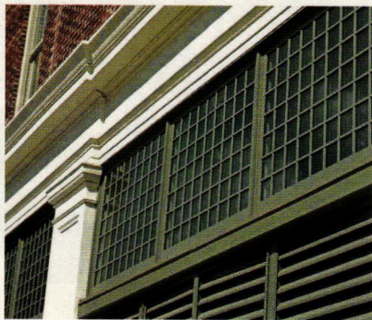
Parrett fabricated these historically styled windows for the Saenger Theatre in New Orleans.
