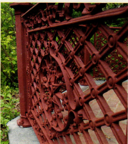
This detail is from a cast-iron gazebo that was recast and fabricated by Wiemann Metalcraft.
