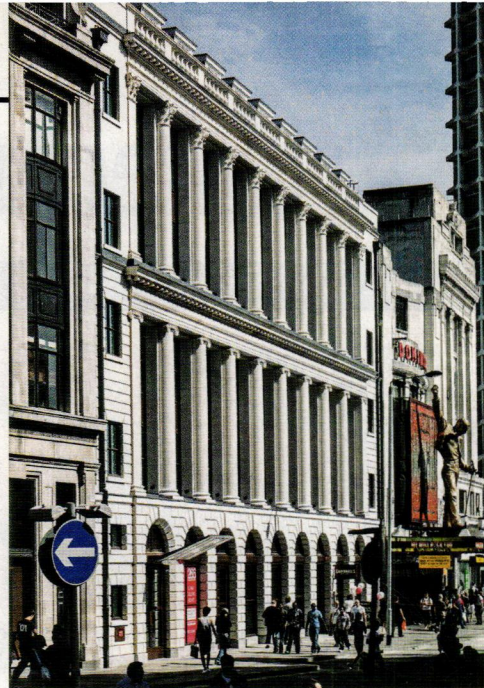
RIGHT: London, England: For this new mixed-use building on Tottenham Court Road, Quinlan & Francis Terry Architects designed a nine-bay façade – 100 ft. wide – in natural limestone, bronze and glass.
