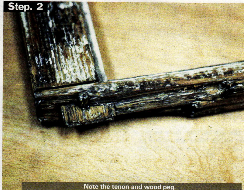
Note the tenon and wood peg.
