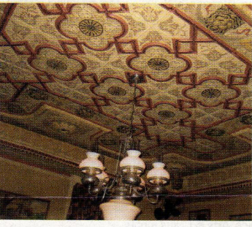
This Oriental-style ceiling was created using pressed-tin panels from W.F. Norman Corp.
