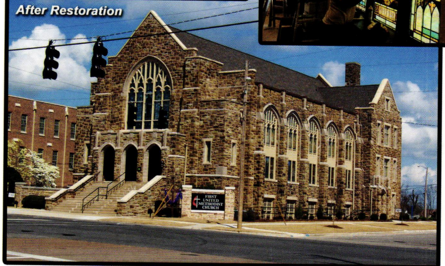
Before and after photos of the F4 tornado damage to the First United Methodist Church of Cullman, Alabama restored by Bovard Studio Inc
