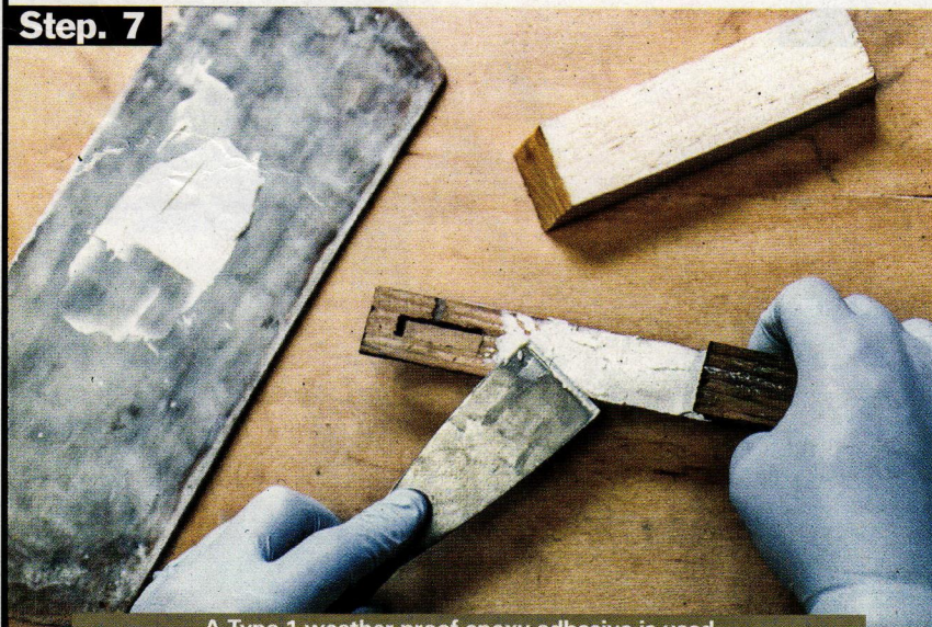
A Type 1 weather proof epoxy adhesive is used.
