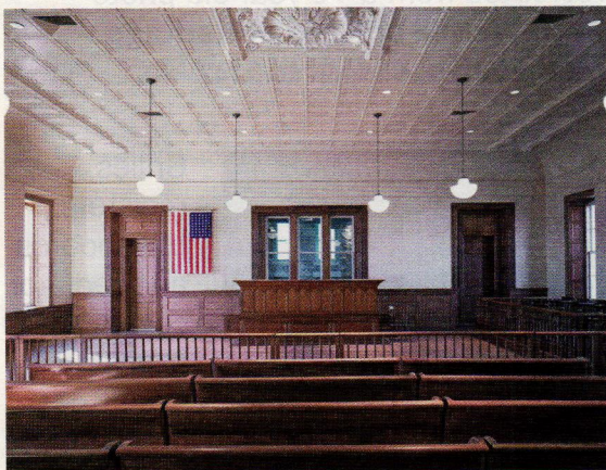
NIKO Contracting fabricated and installed custom pressed-metal wall and ceiling panels to match the originals in the Hunderton County Courthouse in New Jersey. Click on no. 8300.
