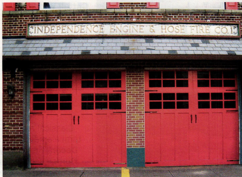
This extra wide door from Fimbel Architectural includes a concrete center post made to match the historic exterior of this fire house. The original building's openings could not accommodate the width of new fire trucks. Click on no. 1953.
