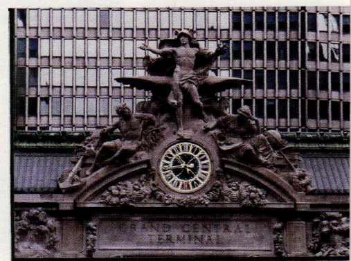
Rohlf's removed and restored the Tiffany clock at Grand Central Terminal NYC, replicating missing parts. Click on no. 6240.
