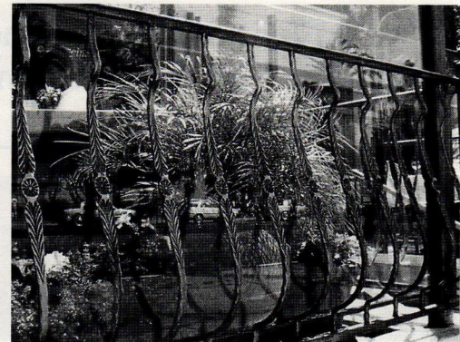
Forged-steel bowed balusters created by King Architectural were used to construct this fence. Click on no. 418.
