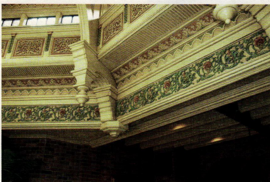
Composition lineal scroll work and plaster ornamental grille work from Decorators Supply Corp. were applied to these walls. Click on no. 210.
