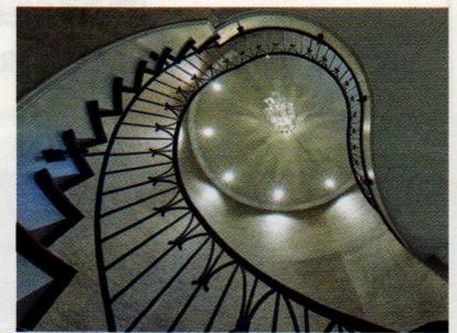
Heritage Metalworks executed this project that features Gothic arches and a hammered finish. The custom designed and forged wrought-iron staircase railing wraps around an eight-ft. long vintage Murano glass chandelier, fusing Cottage Gothic and Modern Glamour inspirations. (Designed by Eric Rymshaw of Fury Design; Photo by Don Pearse Photography, Inc.)
