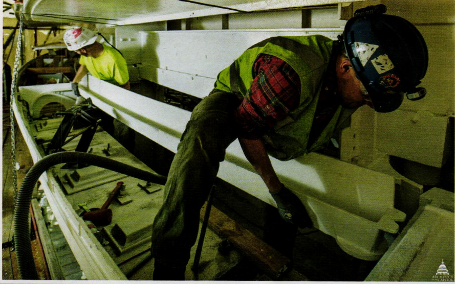
LEFT: The gutter had filled with rust and had to be completely rebuilt and re-assembled.
