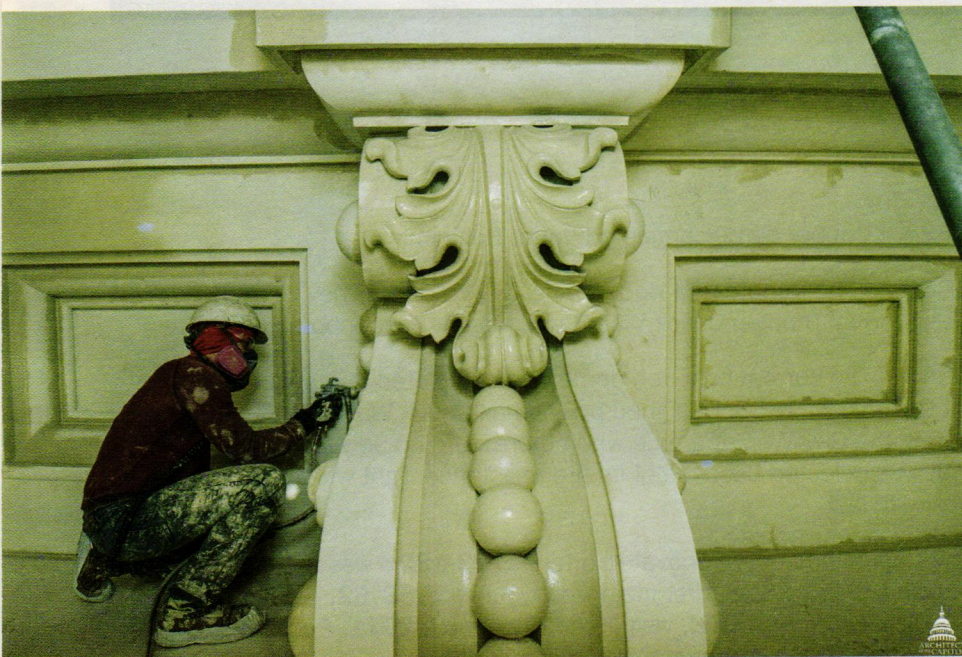
ABOVE: All of the ornament was repaired or replaced and re-installed on the dome.
