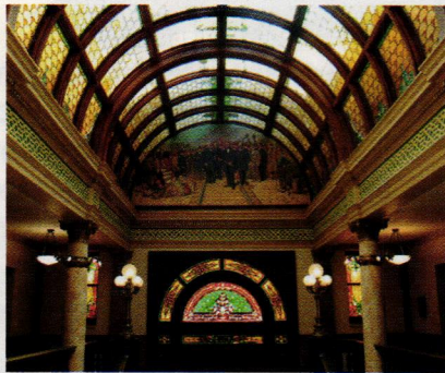
Bovard Studio reconstructed this historic stained-glass barrel-vault ceiling for the Montana State Capitol in Helena, MT.
