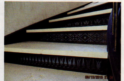
Pacific Register created the decorative metalwork for this staircase.
