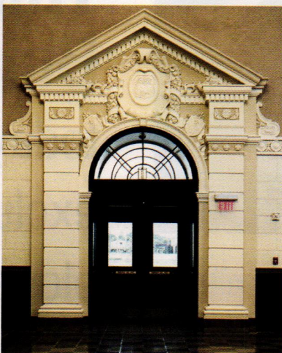
EverGreene Architectural Arts re-created the entrance to the Great Overland Train Station in Topeka, KS.
