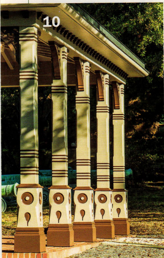
10: Reconstructed porch columns and trim were modeled on those in the historic photos and on other work done in the area in the same time frame.
