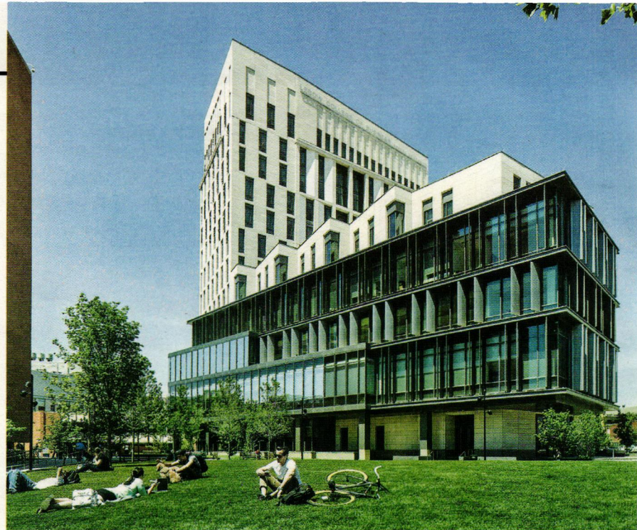
Context dictates architectural style: Departing from the style used at Marist College, at Drexel University in Philadelphia Graham Wyatt and Kevin Smith adapted the Modernist vocabulary of nearby urban buildings for LeBow Hall. LeBow’s triangular plan also helps define a new central quadrangle for the Drexel community.
