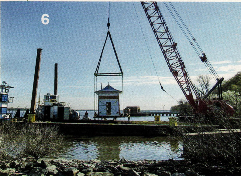
6: A construction barge being used on the historic pier project was "borrowed" for a few days to float the building back up river to the Washington Navy Yard.
