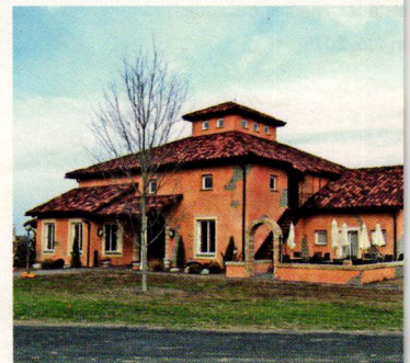
Weathered Mission tiles from Tile Roofs were used for the new roof with an aged look for the tasting room at Blue Sky Winery in Makanda, IL.
