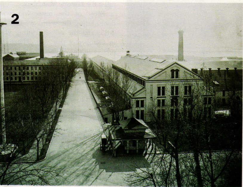
3: The Watchbox as it was found at the Indian Head facility. The porch had been removed and the lower height portion at the right had been added after it was moved in 1909. When the addition was removed, the materials were salvaged
