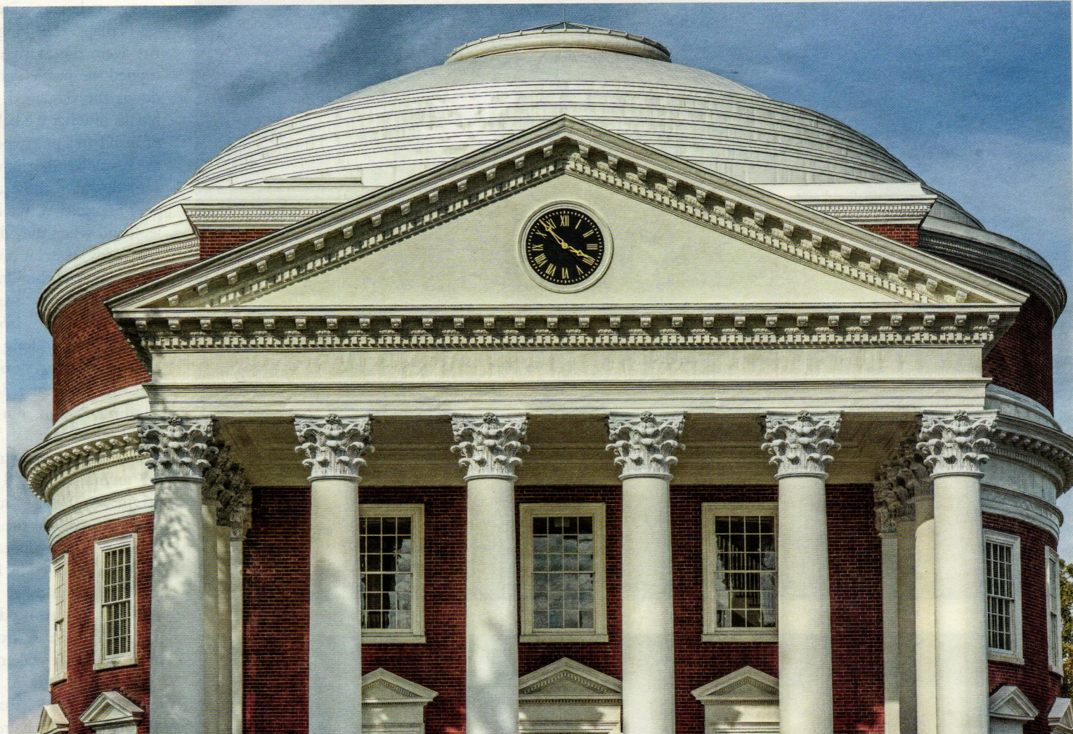
BELOW: Sixteen new Corinthian marble column capitals were carved to replicate Jefferson's capitals, ten for the south portico and six for the north portico, shown here. The capitals were carved of Carrara marble and weigh approximately 7,000 pounds each. The stone was quarried and carved in Carrara, Italy, as Jefferson's had been nearly 200 years before.
