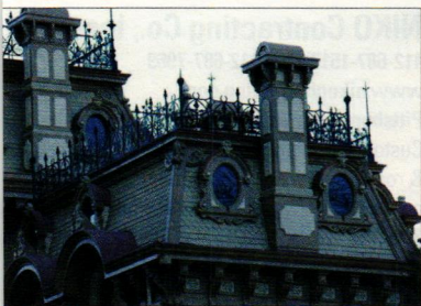
Allen Architectural Metals fabricated this ornate metal roof for the Stanford Mansion in California.
