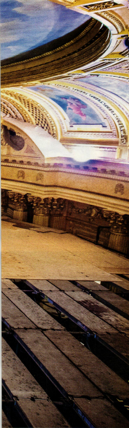
LEFT: The workers from Badger Ladder and Scaffolding constructed scaffolding in the theater so Evergreene Architectural Arts could work on the murals. This area became known as the dance floor.
