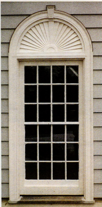
This reproduction 12/12 window with fan was manufactured by Architectural Components .
