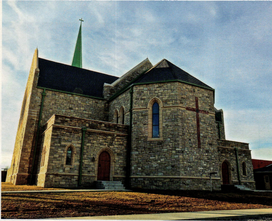
ABOVE: The church is made of Wisconsin limestone from a nearby quarry in Missouri. The shape of a cross is embedded in the stone in the apse.
