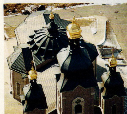
Heather & Little specializes in the restoration, reproduction and design of domes, cupolas, steeples and other sheetmetal elements.
