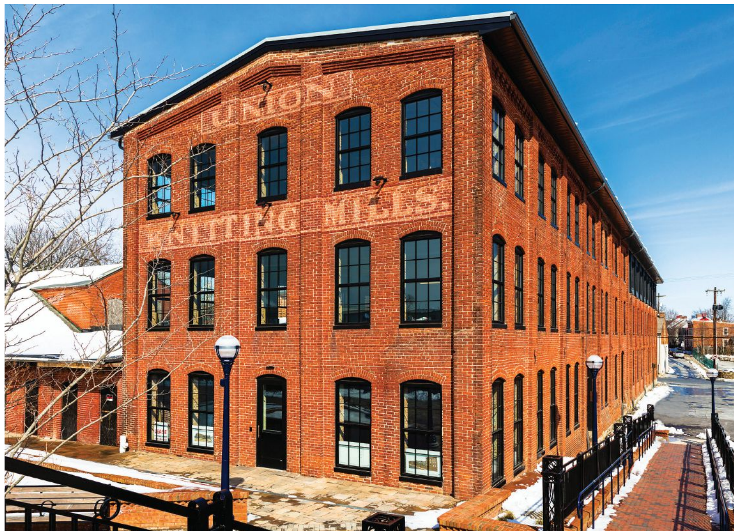
ABOVE Existing building facing Carroll Creek Park. New YKK storefront system windows. New roof and trim.
