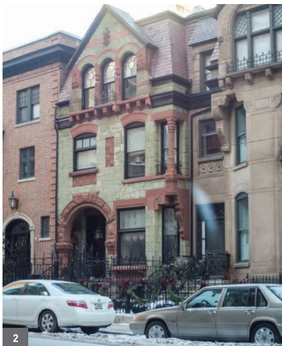
2 Matching the color of the mortar is important to the designed appearance of many buildings. Here the greenish stone and the contrasting red sandstone each have a different color of mortar to underscore the colors.
