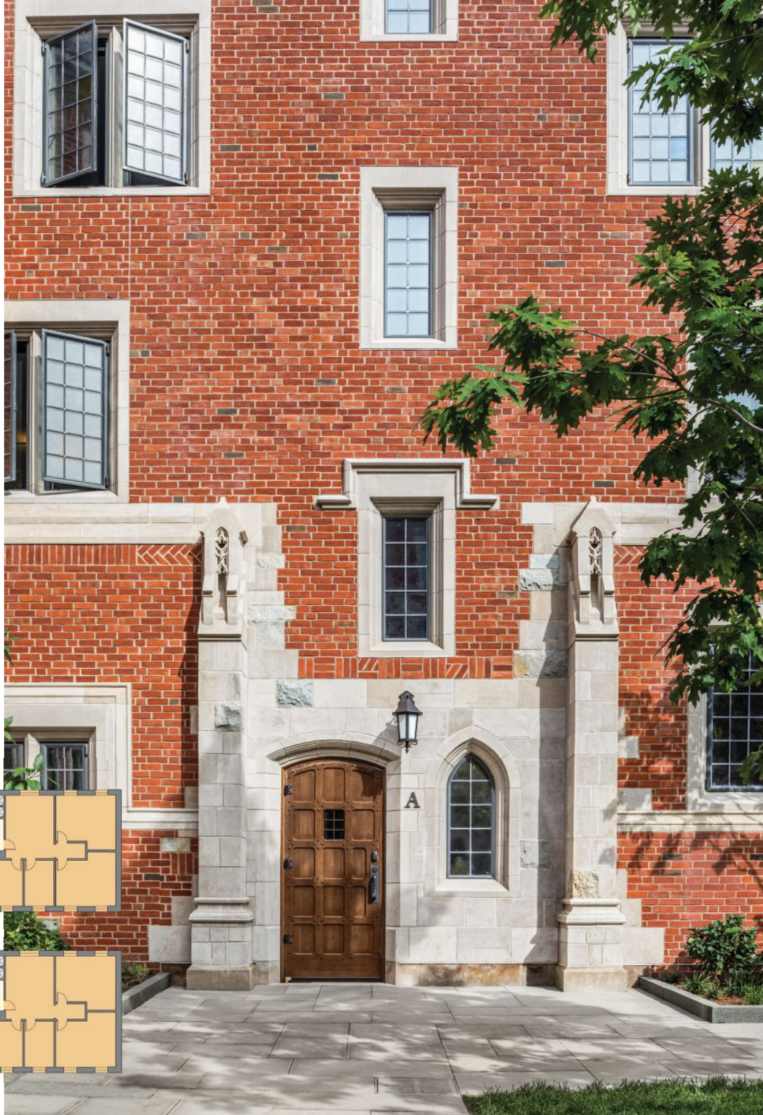
Benjamin Franklin College entryway A, view east from south courtyard.
