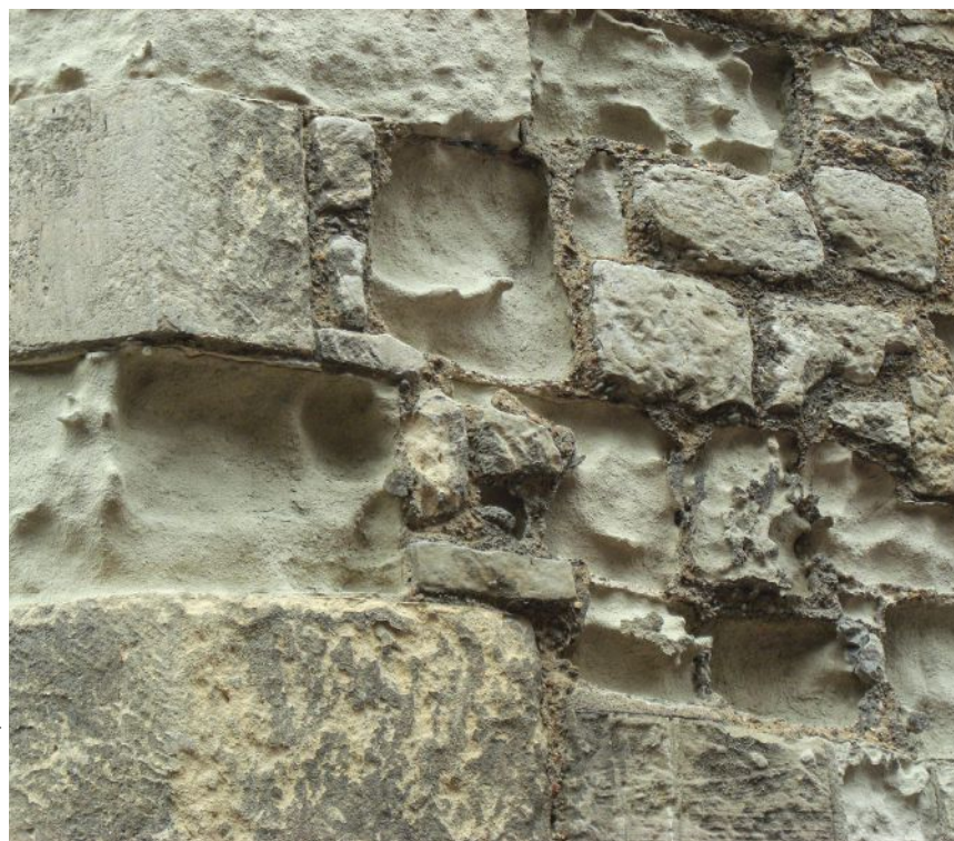
ABOVE Strong acids or high pressure aggregates can remove the surface of the stone, causing the erosion of profile and detail.
