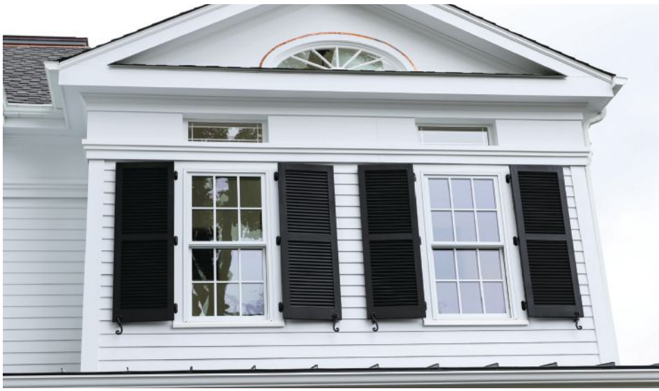
LEFT & ABOVE Aeratis Porch Products manufactures historically accurate, operable, high-density PVC shutters and tongue-and-groove porch flooring.
