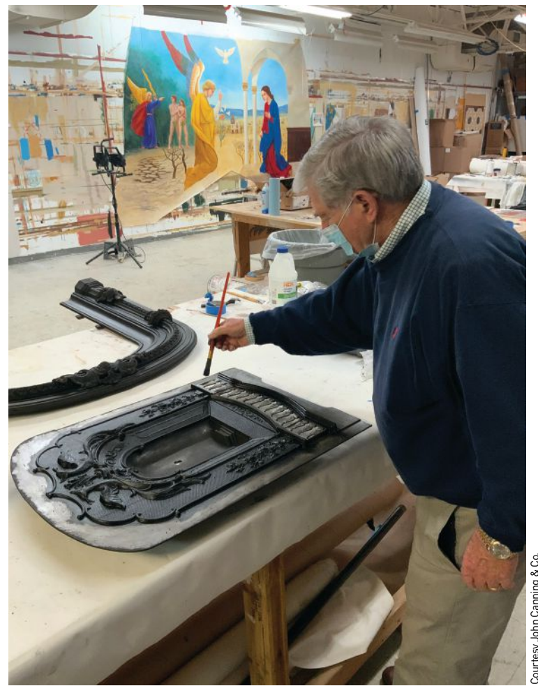
ABOVE Black lead is applied to cast-iron surrounds on a marble fireplace by John Canning.
