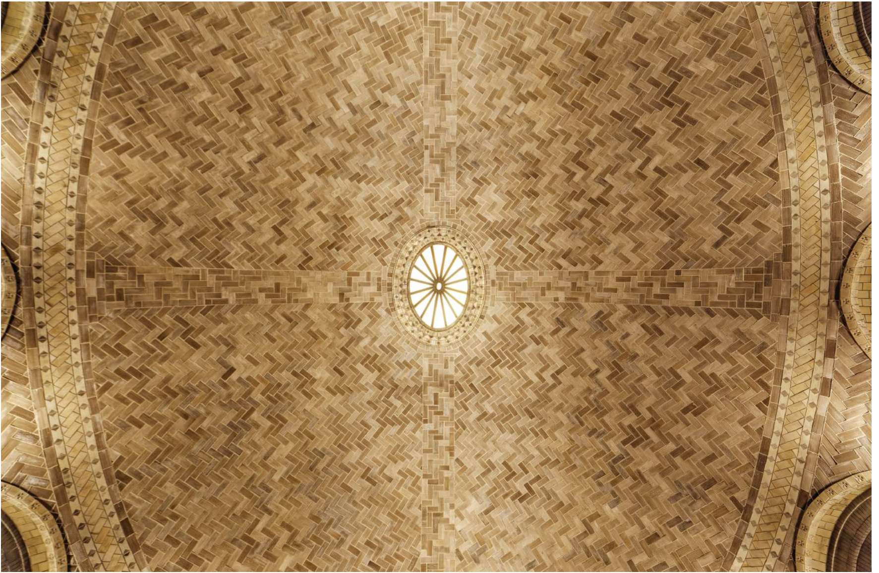
LEFT Chapel of Our Lady exhibits the Guastavino company's early exploration of colored tiles.
