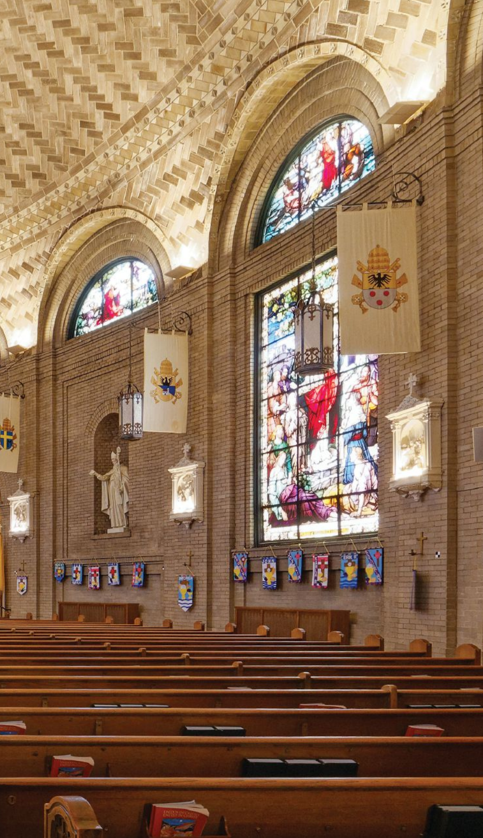
LEFT The dramatic 58-by-82-foot timbrel vaulted elliptical dome of the nave is built of overlapping layers of thin clay tiles. Walls, alcoves, and chapels are all of tile, the floors terrazzo.
