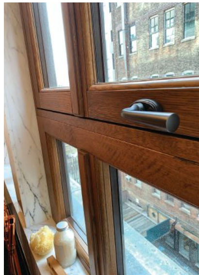
ABOVE Indoors, The Fitzroy windows present the warmth of white oak, quarter-sawn to maximize grain and protected in a light finish.
