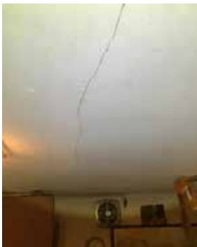
Plaster crack
