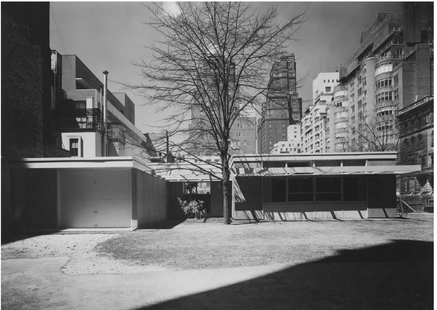
Ain's glass-walled house while it was on exhibit in the Museum of Modern Art's garden in 1950. Ezra Stoller/Esto
