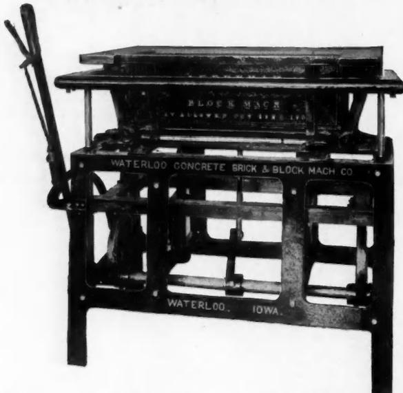
ONE movement of the lever operates the ENTIRE machine, consuming the least time for operation of any machine. Two men will make 250 blocks per day.
