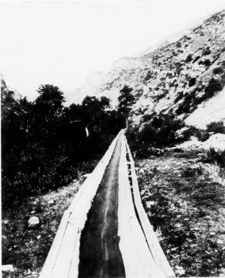
V Shaped Timber Flume, Sheridan County, Wyoming
