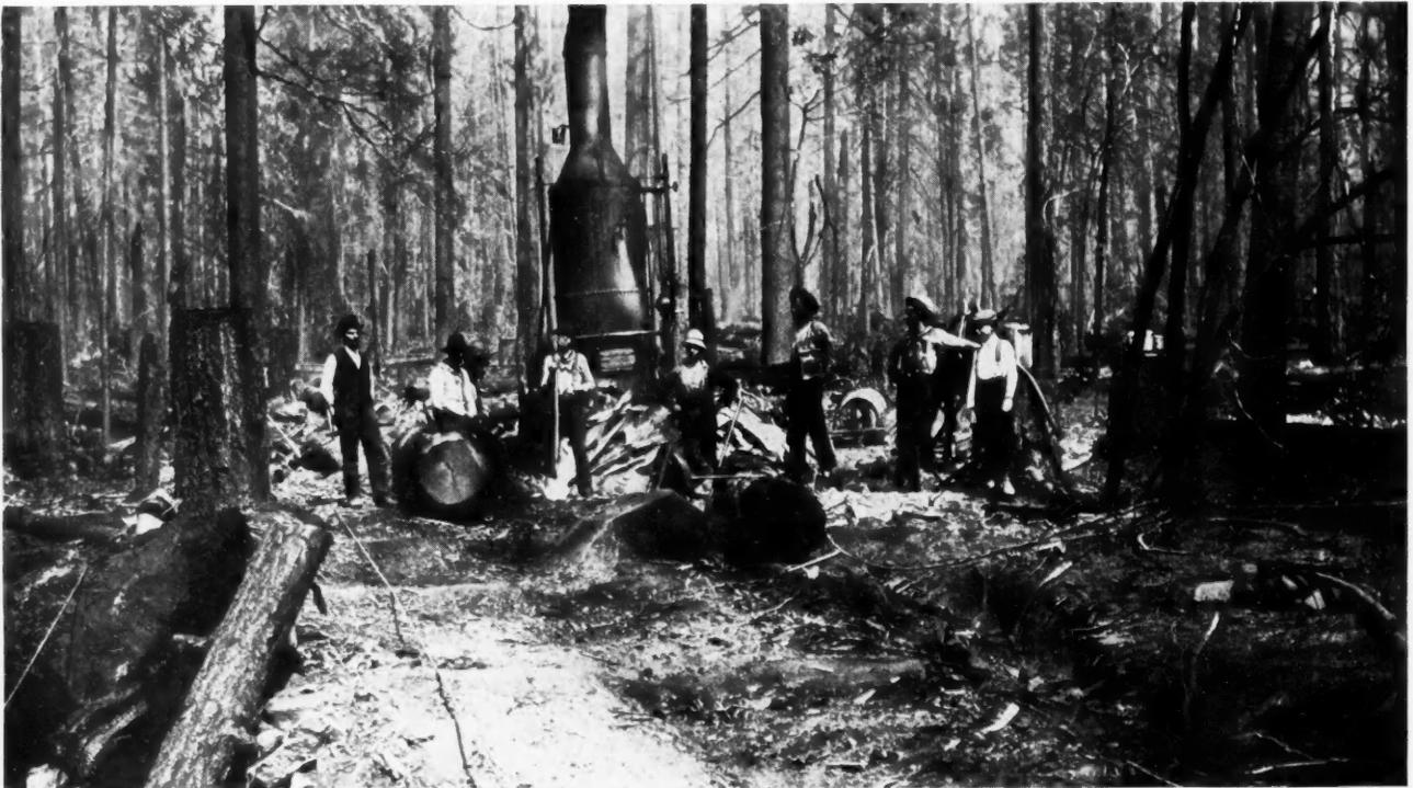
**Hauling Logs to Main Skid Road with Engine and Cable, Cascade, Oregon**
