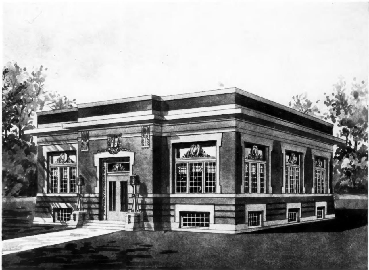
The walls are faced up on the outside with a good grade of vitrified brick, the body of the walls being composed of the common cheap building brick. About
