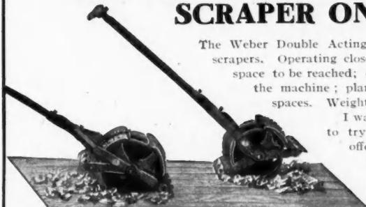
The Weber Double Acting Floor-Scraper has many advantages over other scrapers. Operating close to the base, it allows every square inch of floor space to be reached; can be sharpened without removing the blades from the machine; planes perfectly level and can be used in very confined spaces. Weight of machine 105 pounds.
