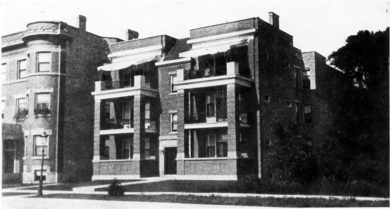
**No. 4. A new six-flat building on Sheridan Road. It represents the best and most fashionable type of flat construction. There are eight rooms and two bath rooms in each flat. Four solid brick walls extend through from front to back, and the construction is what is termed "slow burning." At the left is another six-flat building about two years older. Few private porches were built up to two years ago.**
