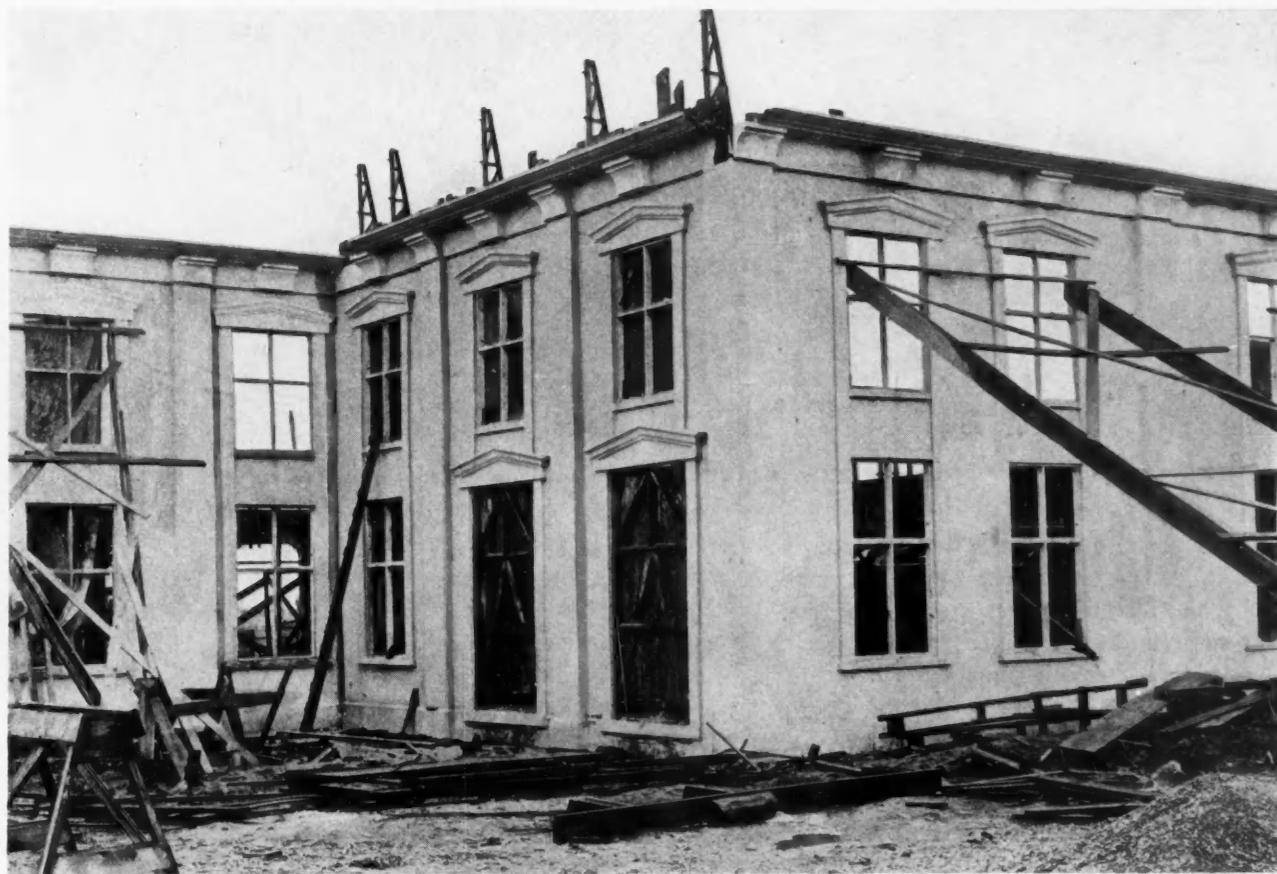
**Fig. 3. The Finished Walls Raised and Corners Locked—A Strong and Beautiful Structure**
