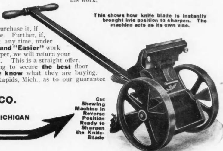
This shows how knife blade is instantly brought into position to sharpen. The machine acts as its own vise.
