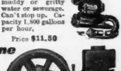
**Contractor's Ditch Pumps** and diaphragm sewer pump will handle any kind of muddy or gritty water or sewerage. Can't stop up. Capacity 1,800 gallons per hour. Price \$11.50
