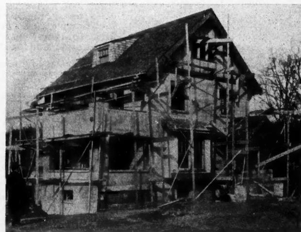
Concrete House Under Construction at New Rochelle, N. Y., for Lorillard Wise, Architect. Van Guilder Hollow-Wall System Used
