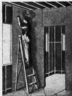
Nailing up panels, using flat-head nails  $\frac{1}{4}$ " from edges, 3" apart and bunn-head nails 6" apart for centers.
