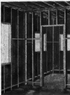
Room ready for Beaver Board construction, studs evenly spaced and headers in correct position to suit panel designs adopted.
