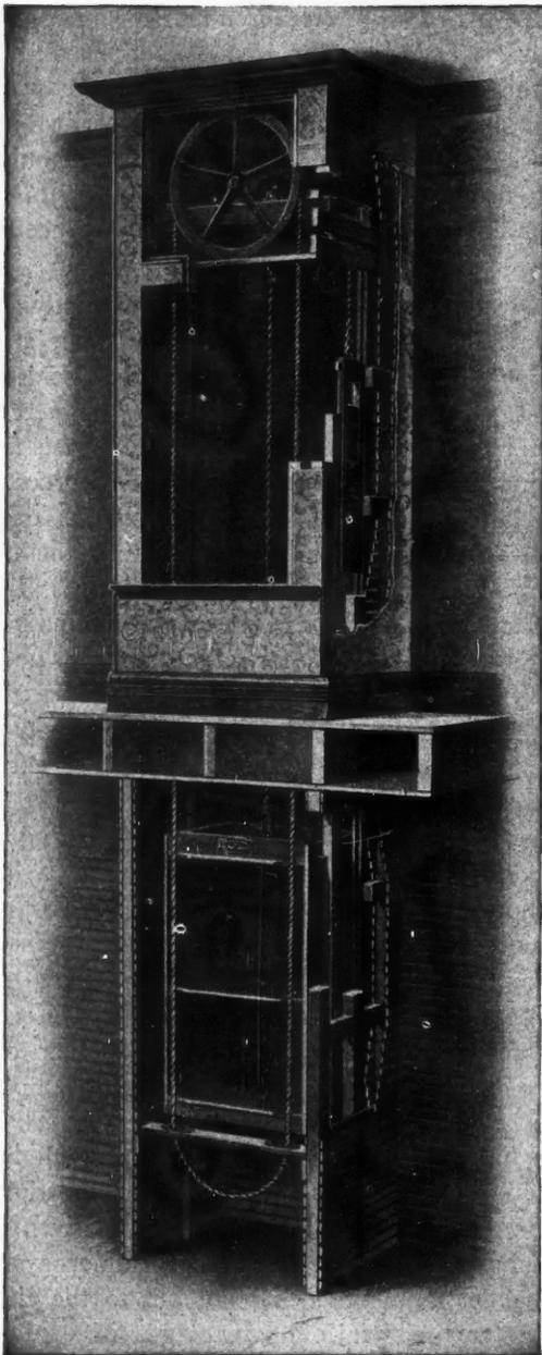
Automatic Brake Dumb Waiter Erected in Plastered Shaft; made by Sedgwick Mach. Works, New York City
