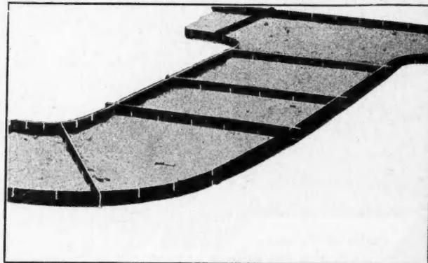
Showing Section of Curved Walk Set Up. Any desired angle in walks can be accomplished with the Ubbink Forms
