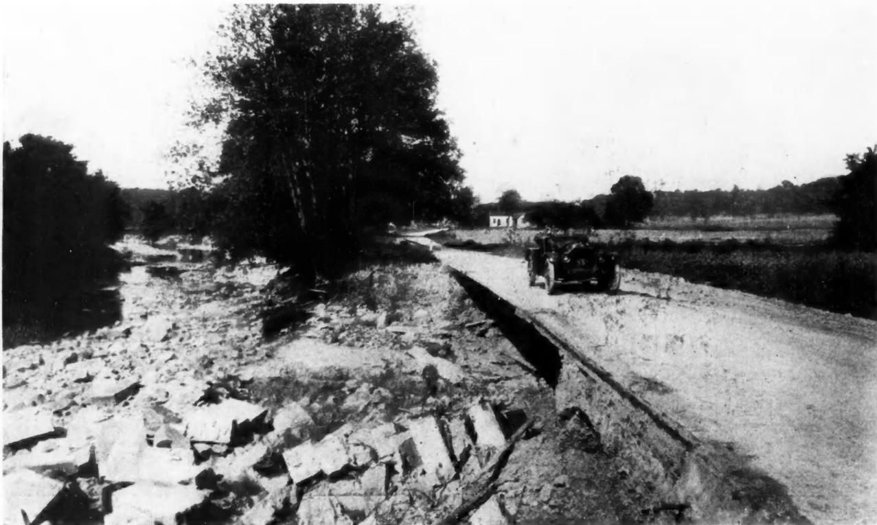
Washout of the Dunham Road Brick Pavement at Tinker's Creek, Near Cleveland, Ohio, in Which Strength of Grouted Brick Was Strikingly Demonstrated.
