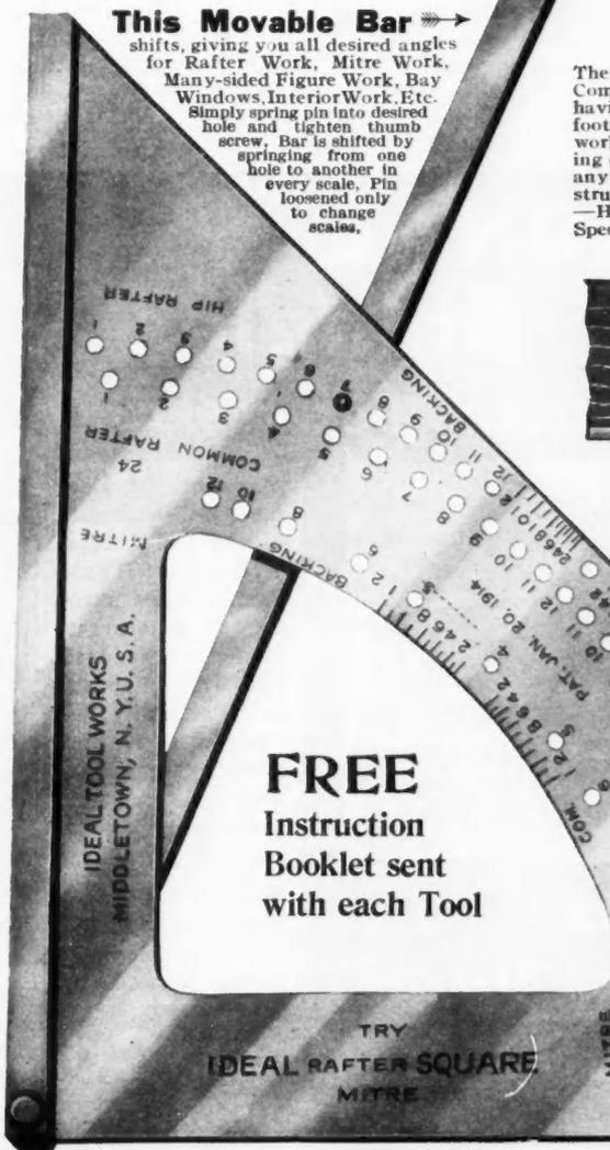
**This Movable Bar** shifts, giving you all desired angles for Rafter Work, Mitre Work, Many-sided Figure Work, Bay Windows, Interior Work, Etc. Simply spring pin into desired hole and tighten thumb screw. Bar is shifted by springing from one hole to another in every scale. Pin loosened only to change scales.
