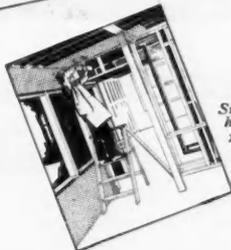
Support to hold ceiling panel in position while nailing.
