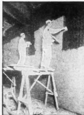
Hy-Rib steel sheathing combines in itself reinforcement, forms, lath and studs. Eliminates forms in concrete roofs and sidings, eliminates channels in partitions, ceilings, furring, etc. Also used in culverts, tanks, silos, etc.
