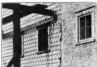
Illustration showing how easily Wyoming Asbestos Stucco is applied as overcoating on clapboards. Simply nail on chicken wire or metal fabric and apply. A Durable, Lasting Finish is the result.
