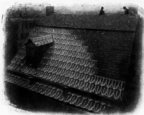
Old Wooden Roof Covered Over with National Sheet Metal Shingles.
