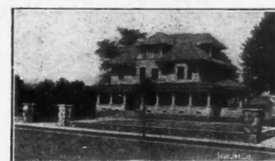
J-M Transite Asbestos Shingles are far more artistic than wood shingles, as they are made with ragged or smooth edges,  $\frac{1}{4}$  and  $\frac{1}{2}$  inch thick, in gray, mottled brown, or Indian red. They possess none of the disadvantages of wood shingles, such as inflammability, warping, splitting and rotting.
