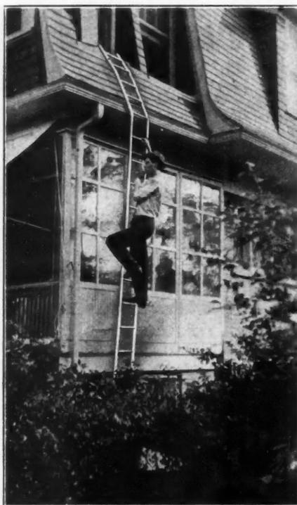
**A Second-floor Ladder Weighs about 25 Pounds; a Third-floor Ladder Weighs About 40 Pounds.**
