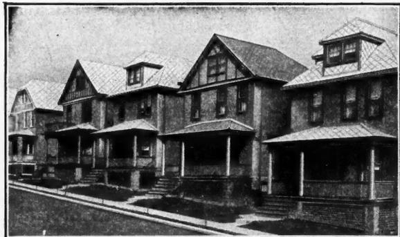
*Houses at Woodcliff, N. J. Roofed with J-M Transite Asbestos Shingles, by James Thompson, Woodcliff, N. J.*
