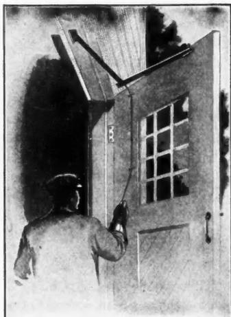
**M**ADE of 1-inch angle iron it has great strength and leverage. Throwing the door open, sets the stay and a slight pull on attached chain releases the lock and draws door shut. Weight 8½ pounds per pr. Write for descriptive circular "A."
