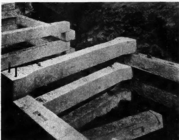
Fig. 1. Concrete Cribbing Units Are Cast Like Fence Posts. Iron Dowels Loose Fitting Into Holes Lock the Ends in Place When in Use.
