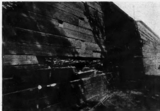
Fig. 2. Short Lived Timber Cribbing at Liberty Avenue and Water Street, Pittsburgh, Replaced with Concrete Cribbing.
