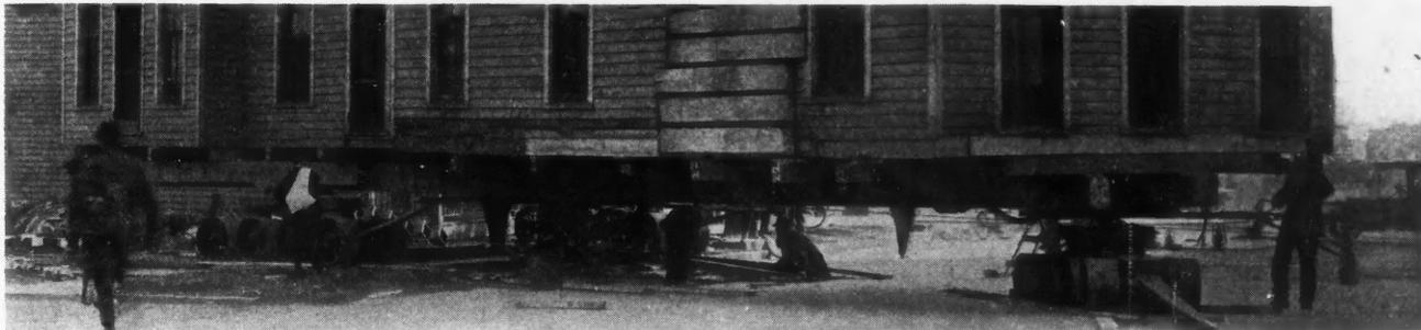
**Fig. 3. Building Entirely Off Foundation. The Front Truck Has Turned and the Rear Truck is Starting to Turn. The Pulling Line is at the Corner and Thus Saves the Time of Resetting the Capstan.**
