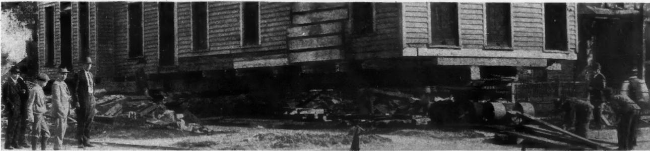
**Fig. 2. Building Half Way Off of Its Foundation. The Track from Curb to Street Does Not Have to be Exactly Level as the Three Point Method of Loading Takes Care of This.**
