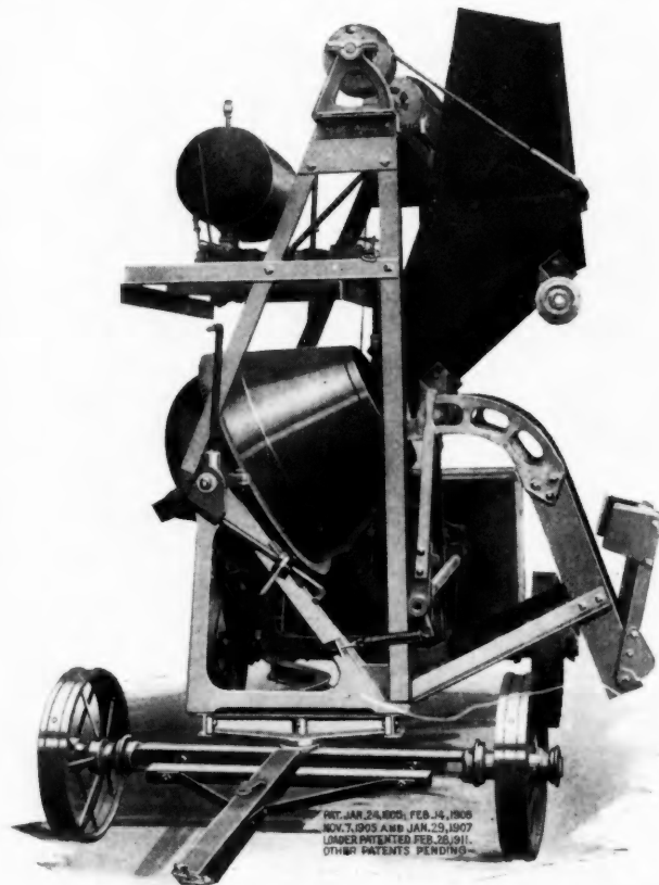
"Wonder" Mixer Equipped with Track Power Loader.
