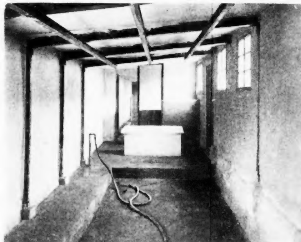
Interior View of Hog House Illustrated Above Built with Metal Lath and Plaster on the Inside and Outside.
