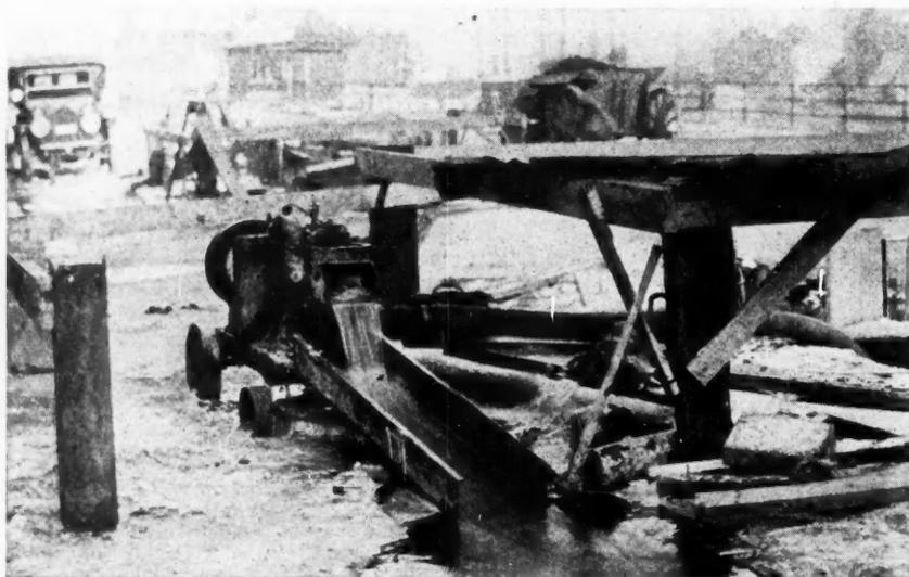
Small Gas Engine and Bilge Pump Are Mounted Together on Low Truck.
