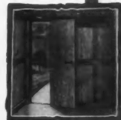
Swinging section of Louden-Hung garage door permits individual entrance and exit without moving entire door.
