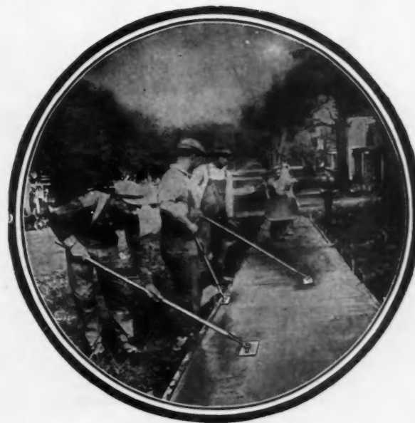
The Easy Working Positions of Men Using Long Handled Tools.
