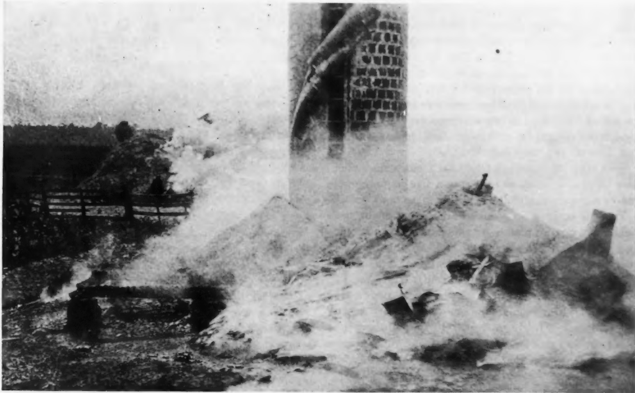
Unusual Photograph of Fire Near Freeport, Mich., Where Two Large Barns and a Straw Stack Burned, Leaving Practically Unharmed the Clay Tile Silo. The Doors and Feed Shute Were Burned Off; That Was All.
