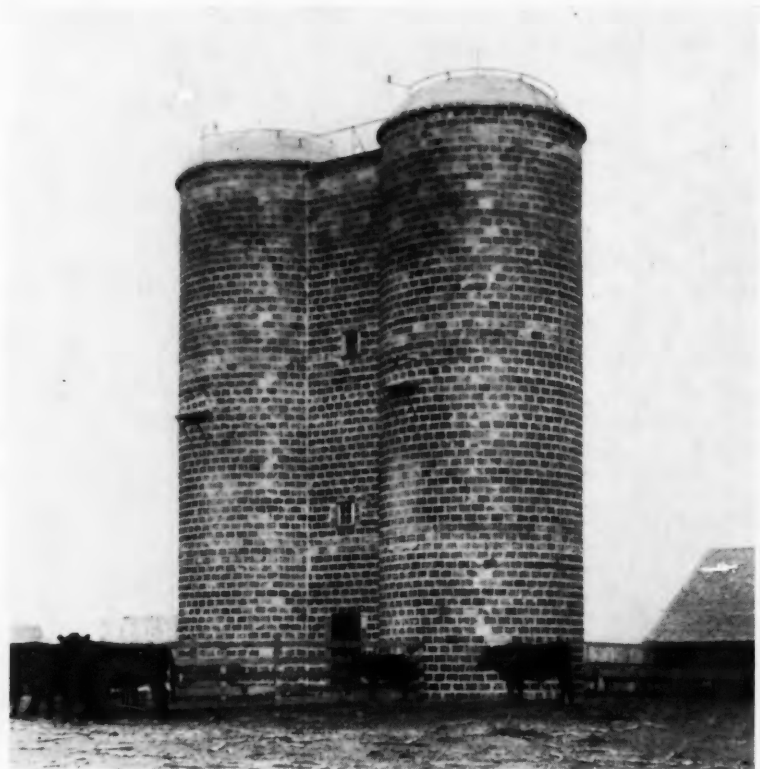
Big Double Silo with Feed Chute, All of Hollow Clay Blocks.
