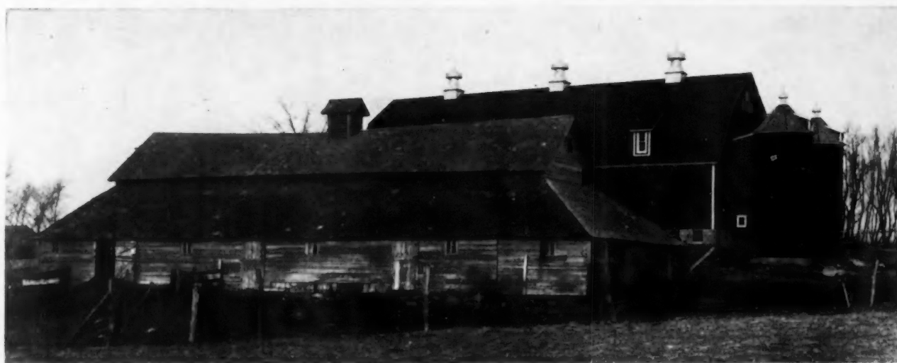
The Old and the New. A Striking Contrast in Barns on the Farm of P. F. Coggins, Blooming Prairie, Minn. Notice Particularly the Difference in Cupola Ventilators. The Modern Air-Tight Barn Requires a Scientific Ventilating System with Permanent Aerators on the Roof.
