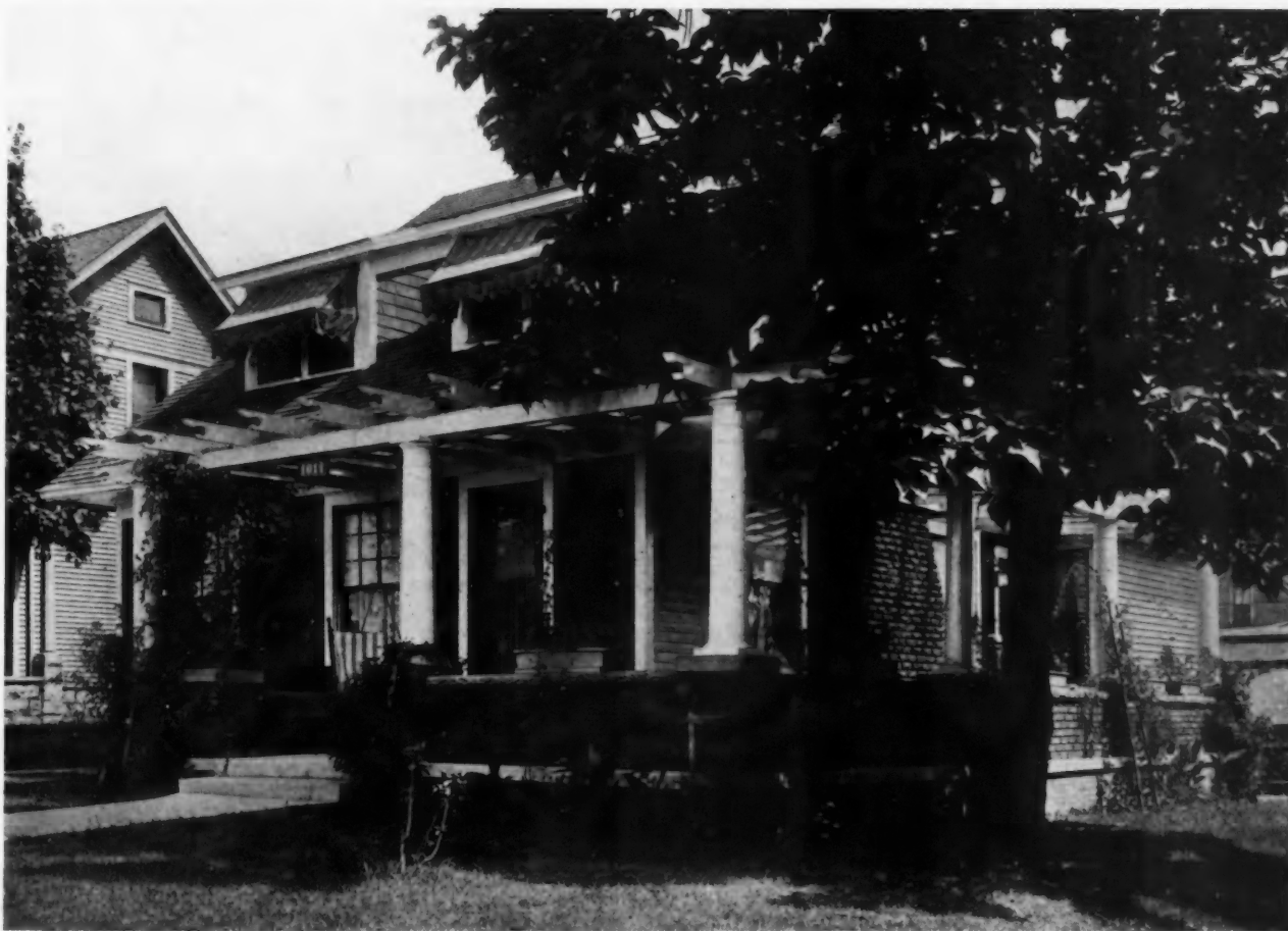
The Transformation Brought About by the Construction of a Pergol Porch with Face Brick Base and Wire Glass Roof is Clearly Evident in This View.
