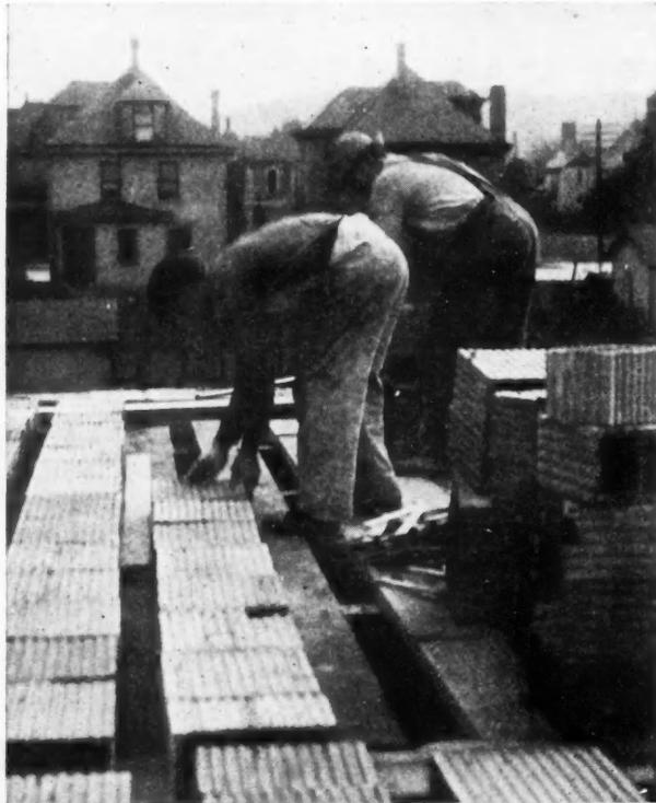
Placing Hollow Tile on 2 by 10-Inch Plank Centering. Note That Solid Centering Is Not Required.
