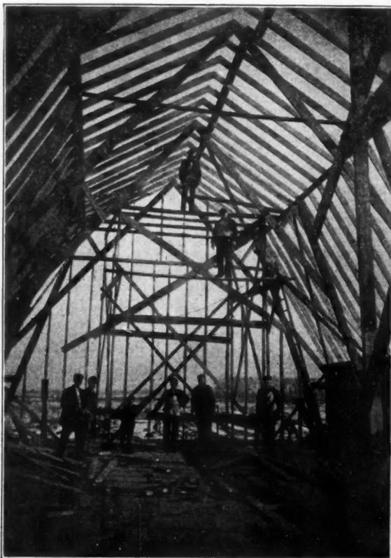
Fig. 2. Method of Framing Roof Timbers.
