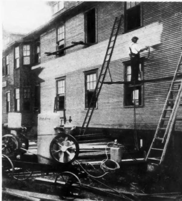
By the Use of This Portable Equipment, Paint Is Forced Thru the Tubing and Sprayed on the Wall by Compressed Air.
