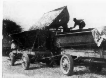
Materials Are Shoveled From the Car Into the Loader and Only a Few Seconds Are Required to Load the Truck or Trailer.
