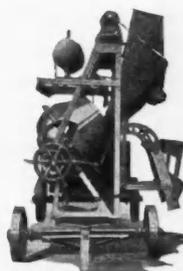
See perfect balance of machine when the loader track is folded for moving. Note the quick emptying skip.
