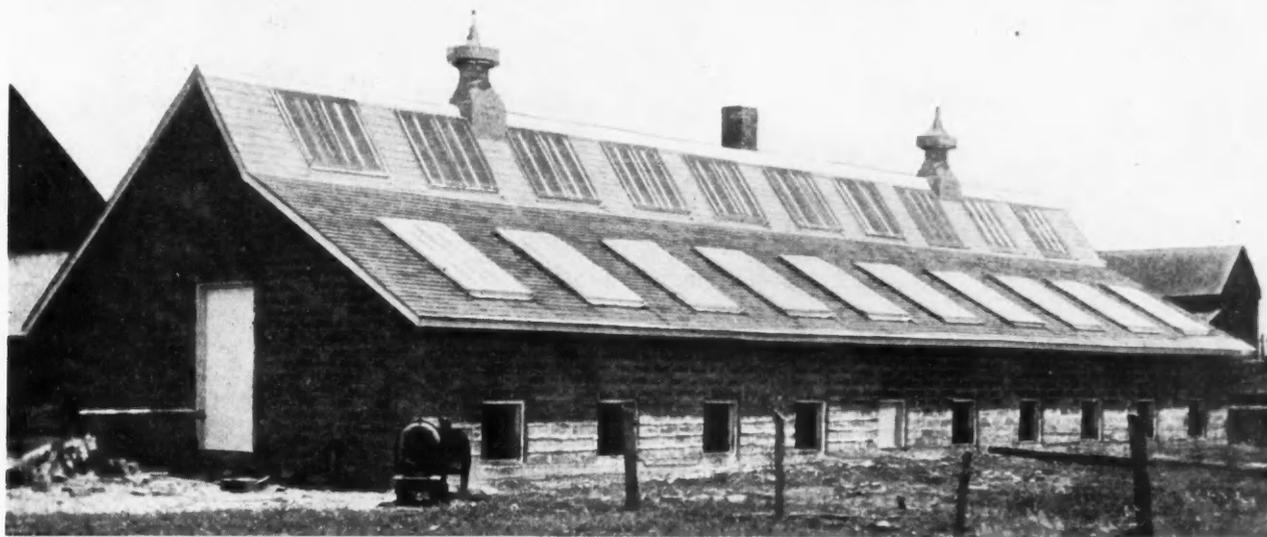
Excellent Winter Hog House Design of Concrete Blocks With Roof Windows and an Efficient System of Ventilation.
