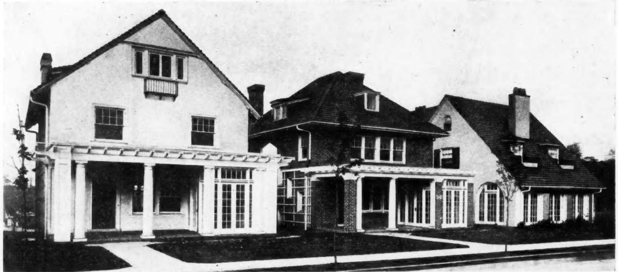
A Good Example of Tile Roofing on Tile Houses Faced with Stucco and with Brick; Location, Darlington Road, Pittsburgh, Pa.; Harry S. Bair, Architect.
