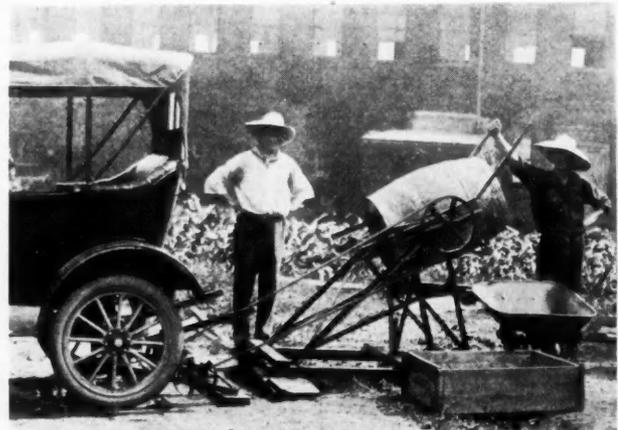
Auto Power Plant Operating Barrel Concrete Mixer.
