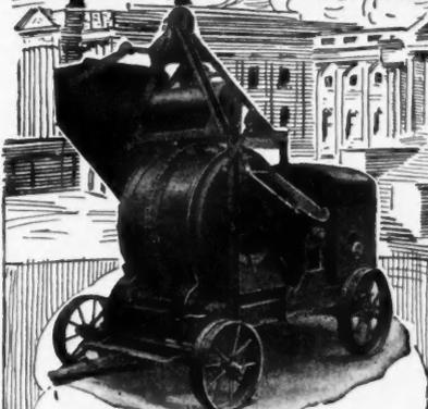
Building Mixers with Automatic Power Loader and Measuring Water Tank.
