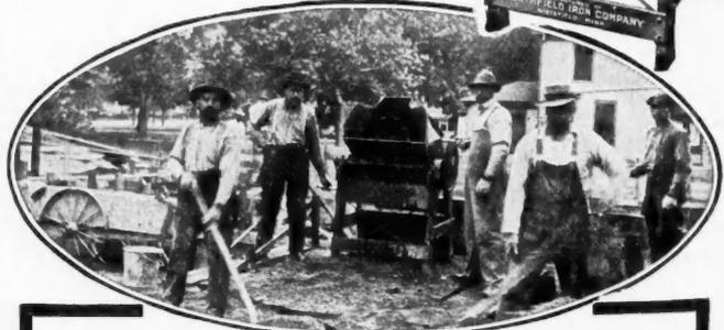
The above is just a good, fair showing of what the NORTHFIELD Hand Mixer will do—not an unusual or record performance by any means. It turns out a 4 ft. batch of perfectly mixed concrete every minute and will mix 30 to 40 yards of slush concrete a day under any ordinary working conditions.
