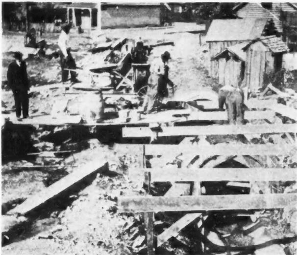
The Bell Construction Co., putting in a 7-foot storm sewer at Lexington, Ky., found a great saving by moving their special light mixer with end discharge right up to the forms. They much prefer this to wheeling the wet concrete.
