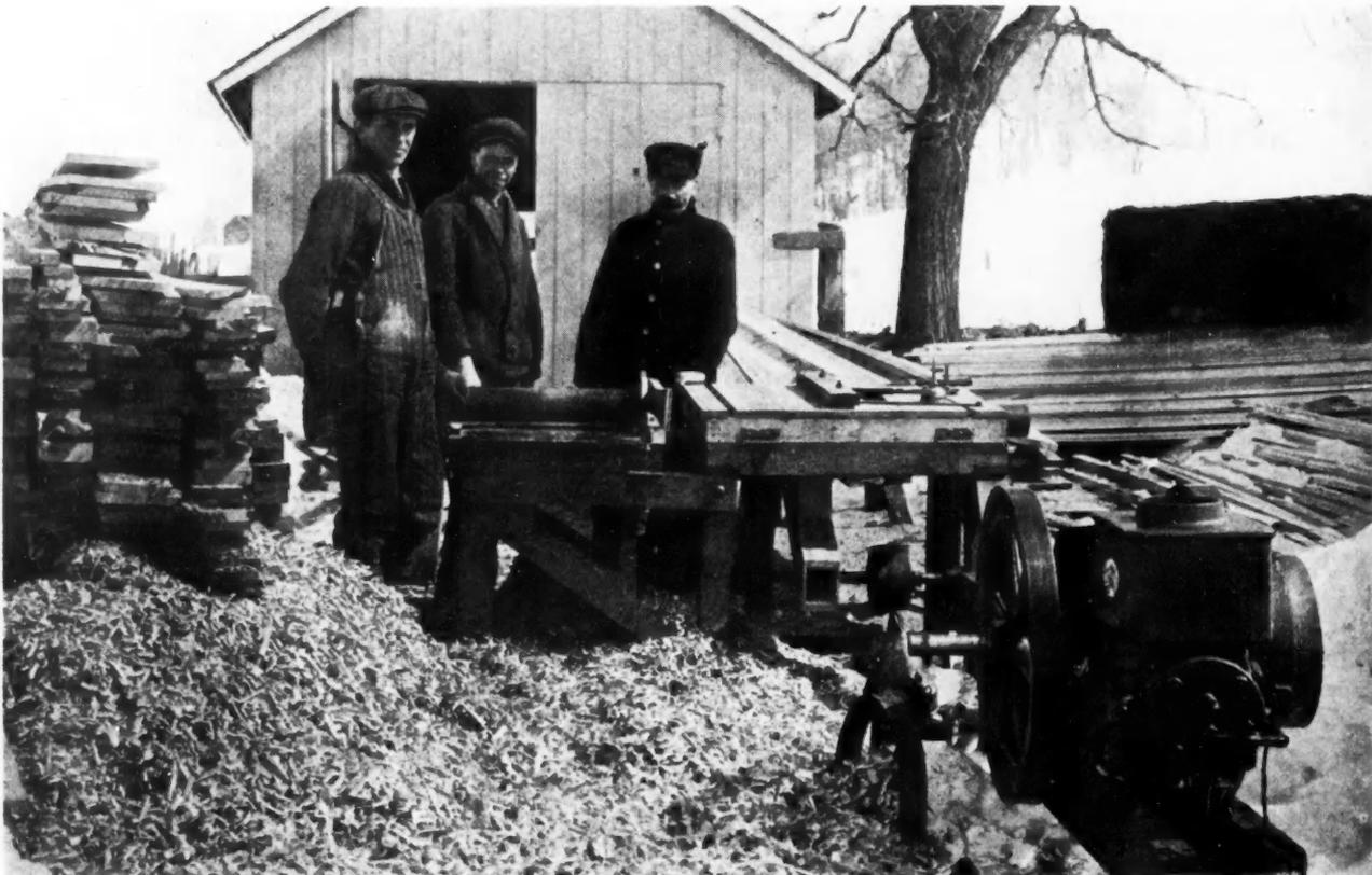
Jointer Head Mounted on Home-Made Table Planed 6,000 Feet of Green Cottonwood.
