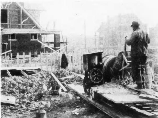
Concrete mixers have been perfected for builders' use. Note how convenient this loading platform is for charging the mixer by wheelbarrow. The mixer is often placed to discharge directly into the forms.
