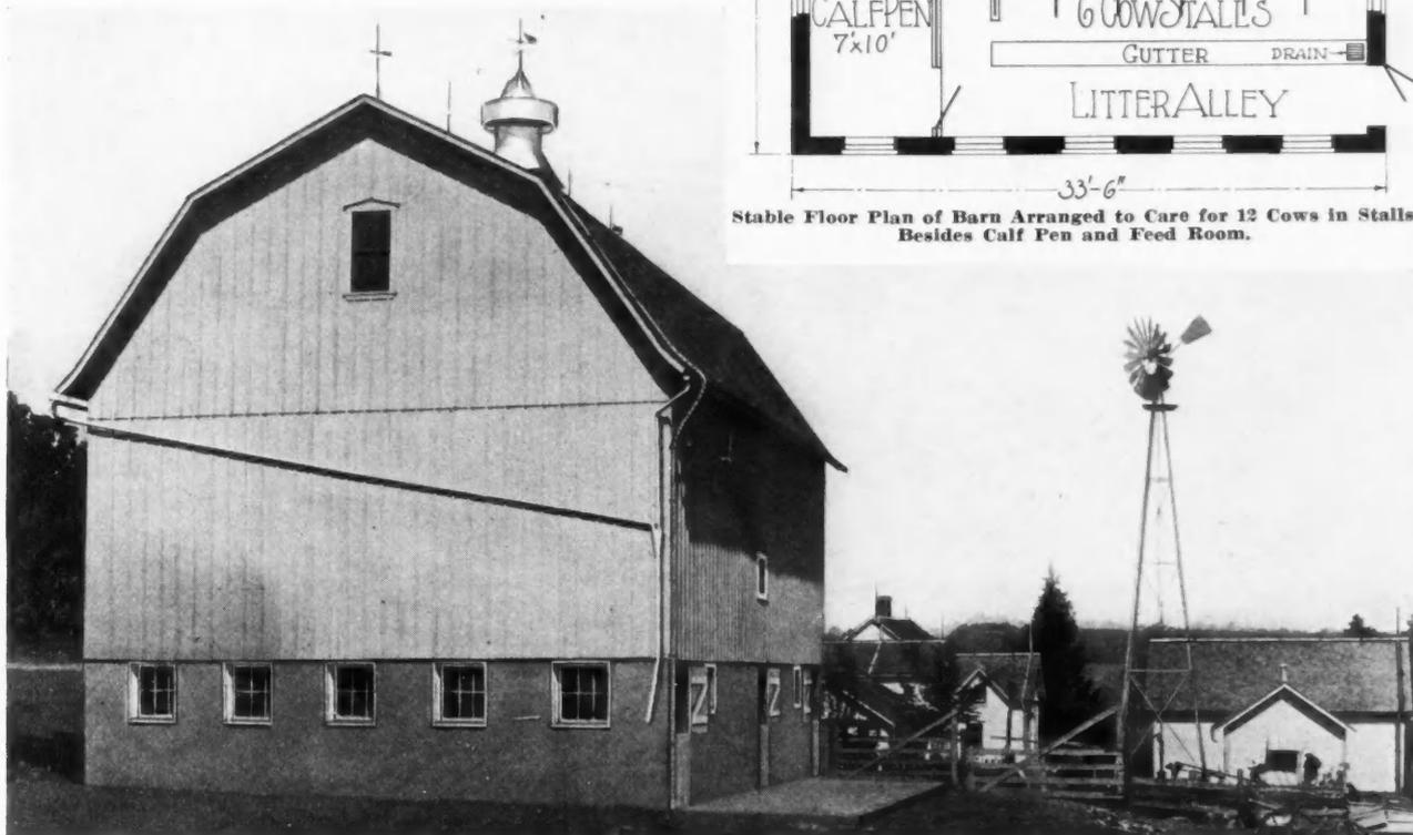
Photograph of Barn, Size 33 Feet 6 Inches by 34 Feet, that Has Been Remodeled to the Extent of Concrete Stable Floor and Approach, and Basement Walls. Ventilating System Was Put in and All Buildings Rodded for Lightning Protection.
