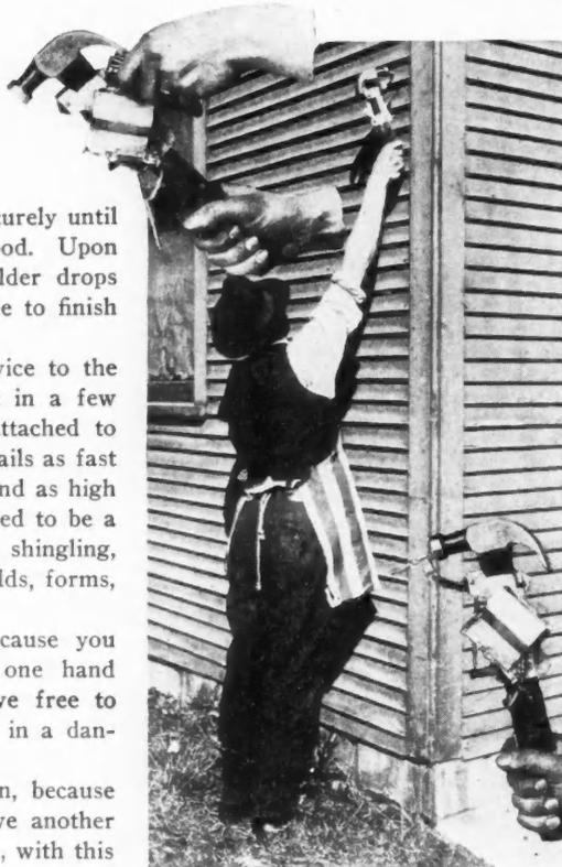
Nail Feeder Being Loaded and Used for High Nailing.
