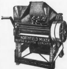
**THE** Little Mixer with an enormous capacity. Easily mixes 30 to 45 cu. yds. of finished concrete per day. 6 to 9 cu. yds. per hour is possible under favorable conditions. It hoes, plows and stirs breaking up all the tiny cement globules and giving a quick, thorough uniform, dependable mix. Can always be set to discharge direct into form.
