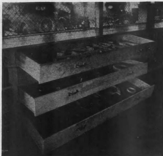
Gaskets Filled in Long Drawers to Prevent Parts from Getting Mixed Up. This Arrangement Saves Much Time and Labor.
