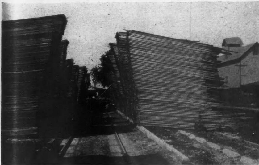
Lumber Yard with Concrete Supports for Piles and Combination Trackway for Yard Trucks and Push Carts. The Rails Are Set on Concrete Slabs Which Are Wide Enough to Serve as Wagon Wheel Track.
