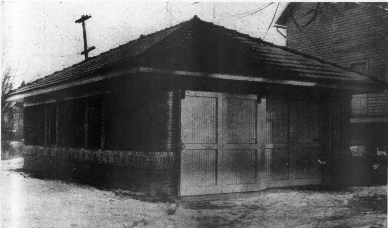
Two-Car Garage of Hollow Tile Construction with Brick Veneer. The Roof Is Clay Tile. Two Kinds of Brick Were Used—Yellow, Rough Texture Brick Up to the Soldier Course and Red Brick Above. Size, 26 by 26 Feet.
