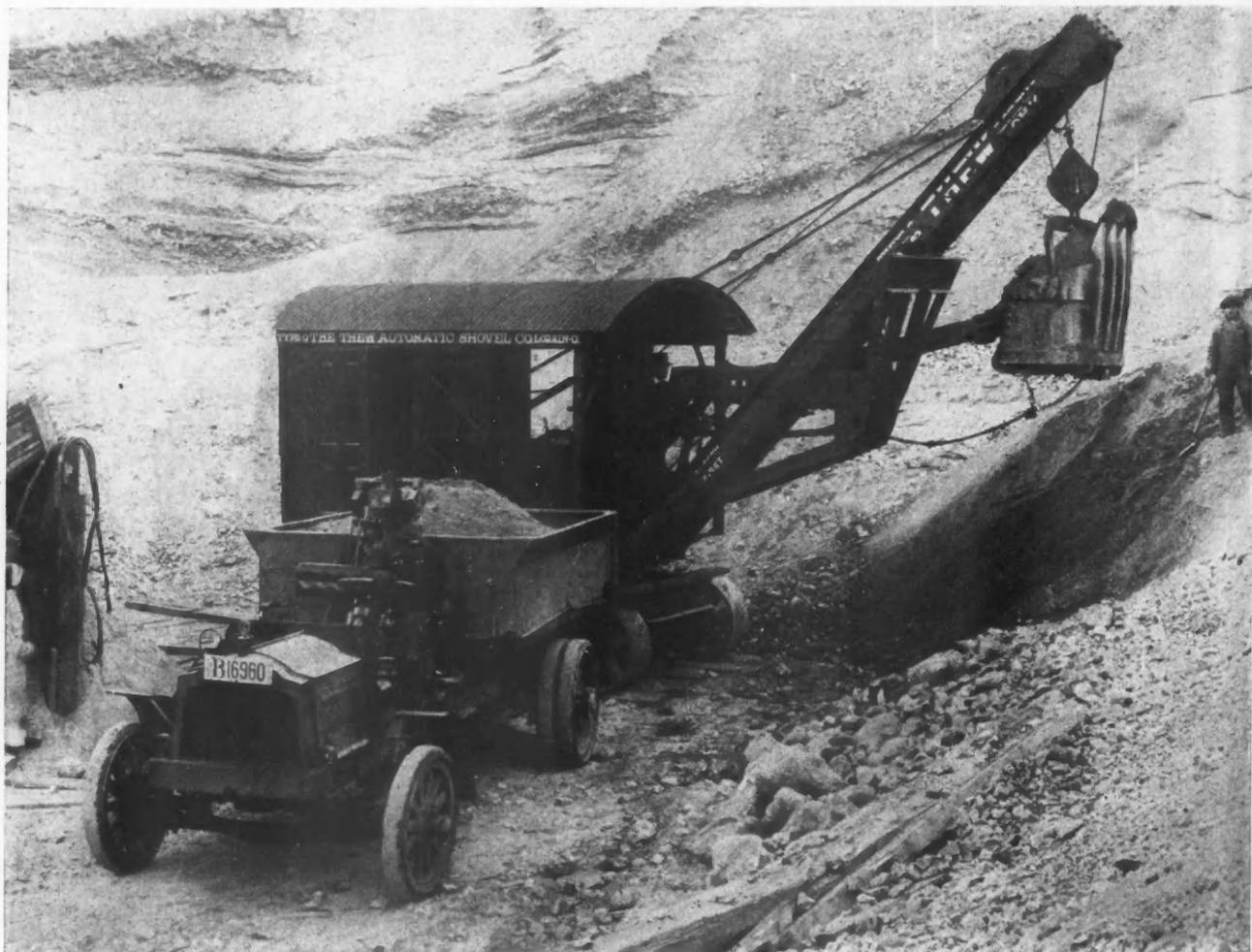
Four-Ton "Packard" Truck Getting Heavy Load of Gravel for Concrete Foundations. This Truck Is Owned by the Beaver Brook Foundation Co., Waltham, Mass., Who Make a Special Business of Foundation Work. This Is the Type of Heavy Truck That Will be Used Extensively for Hauling Bulky and Heavy Material This Spring.
