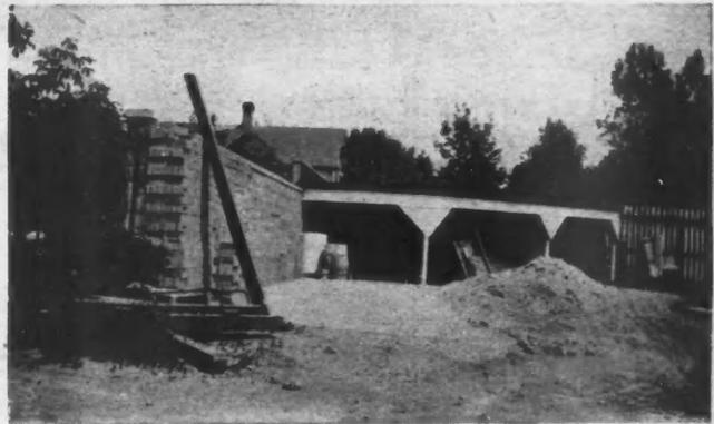
Builders' Supply Yard Equipped with Concrete Platform for Mixing Concrete to Be Worked Up in Spare Time Into Concrete Block.
