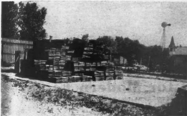
Stacking Place for Shingles Made of Concrete.
