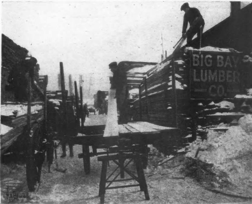
Starting a New Load While the Other "Martin Rocking Fifth Wheel" Semi-Trailer Is Being Hauled to the Job. The Use of Trailers Has Made the Hauling of Lumber 15 and 20 Miles an Everyday Occurrence.
