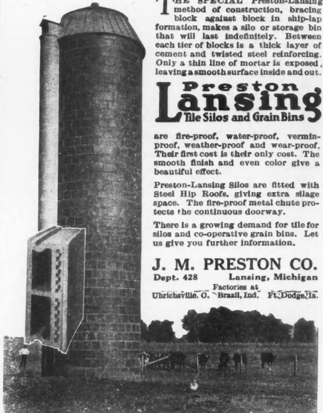
THE SPECIAL Preston-Lansing method of construction, bracing block against block in ship-lap formation, makes a silo or storage bin that will last indefinitely. Between each tier of blocks is a thick layer of cement and twisted steel reinforcing. Only a thin line of mortar is exposed, leaving a smooth surface inside and out.
