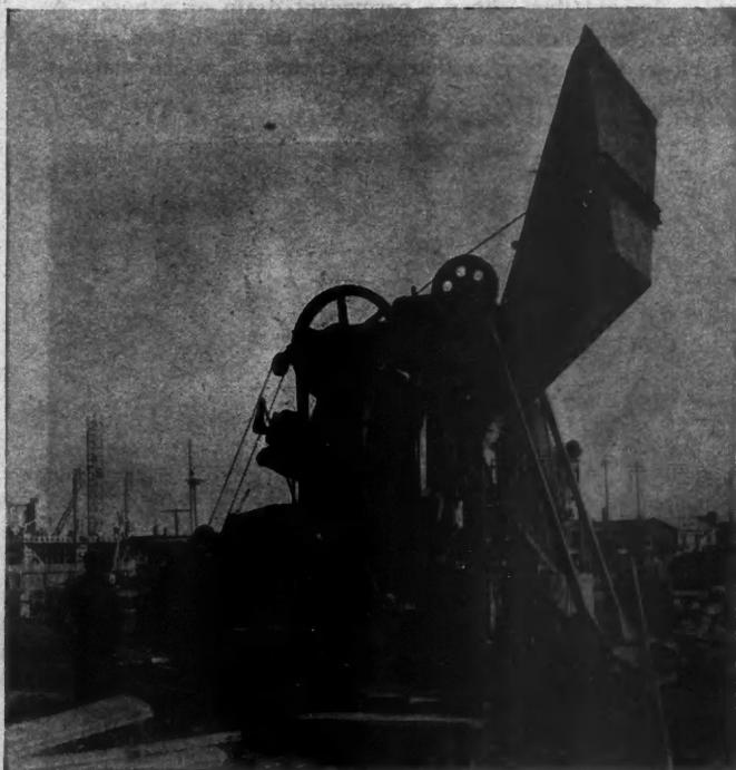
This Paving Mixer Poured the Footings of the Columns in the New Cadillac Plant Erected in Detroit. It Was Used in a Variety of Ways in the Construction Work.
