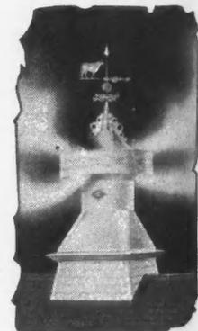
The King Aerator drawing moisture out of a building. The steam can easily be seen in cold weather.
