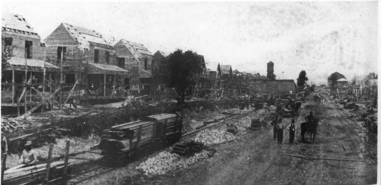
**Whole Row in Course of Construction. This Picture Shows How Lumber and Material Were Hauled to Scene of Operations on Narrow Gauge. Speedy Hauling Prevented Many Delays.**
