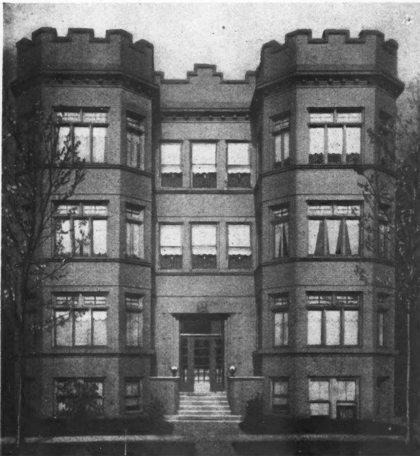
Six-Apartment Building of Brick Construction with Veneer of Light Face Brick. Four Apartments Have Six Rooms Each, the Two Lower Ones Have Five.
