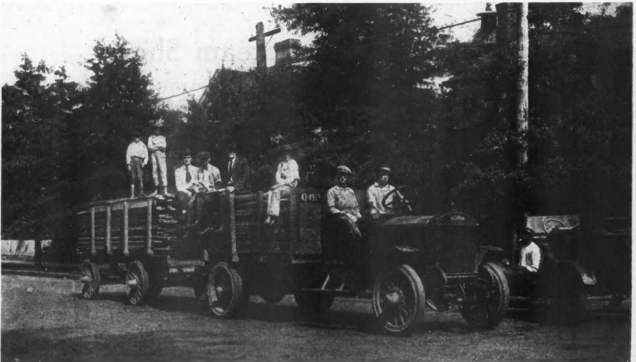
Two-Ton "Indiana" Truck and Trailer Loaded with 3,000 Feet of Lumber for a Job Out in the Country. The Sipsey River Lumber Co., Aliceville, Ala., Have Been Using This Combination for a Year. They Carry a Double Load on One Trip by Using the Trailer.
