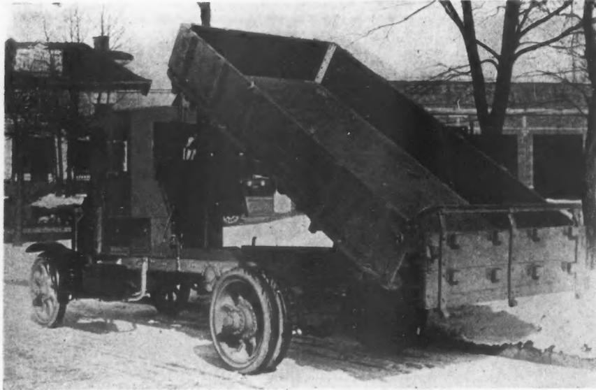
This "Federal" Truck Owned by Eggert Bros., General Contractors, Akron, Ohio, Has a Utility Dump Body That Is Very Useful. This Picture Shows It with the Side Boards Fitted for Hauling Gravel and Bulky Material. It Is Dumped by Means of a Hydraulic Hoist.
