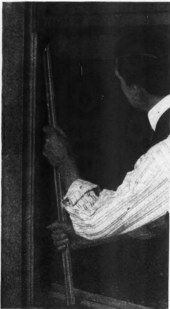
Installing Parting Bead in Weatherstrip Job. Builders Find This Work a Source of Extra Income in the Fall.
