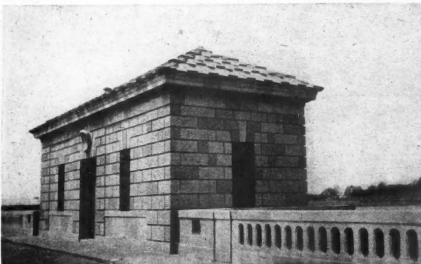
Figure 10. Concrete Block Structure of Hand Tooled Blocks, Made with Marble and Granite Aggregates. The Surface Texture Is Unusually Attractive.
