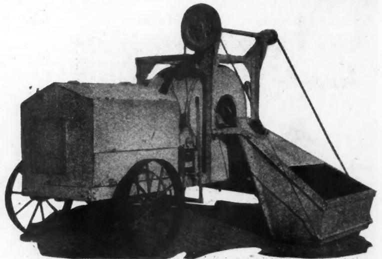
Mixer Which Discharges Batch in Ten Seconds. It Is Built for Size and Speed and Has a Capacity of 7 cu. ft.
