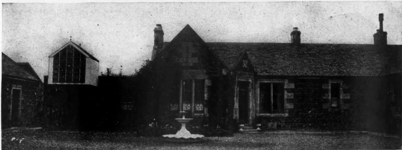
Stone Workman's Cottage at Ayrshire, Scotland. Durability Is One of the First Considerations of the Builder. Climate Determines the Thickness of the Walls. Note the Shingle Roof Which Is Rapidly Displacing the Thatch Formerly So Popular
