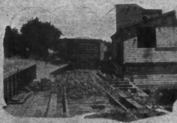
TODAY—The Kissel engineered way. Empties a 50-ton carload in 10 minutes by dumping through bottom of car into bins inside loading shed, saving 14 hours, 50 minutes.
