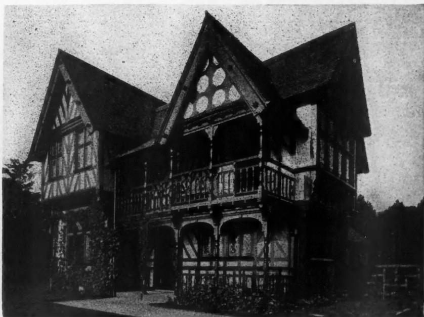
Half Timber Type of House at Largs, Scotland. In This Construction Heavy Timbers Are Framed Together and the Panels Filled with Brick, Then Coated with Stucco. Note the Sharp Gables
