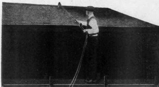
Applying Paint on a Roof. By Adding Sections Scaffolds and Ladders Can be Eliminated in the Painting Job. This Machine Will Apply Waterproofing Material.
