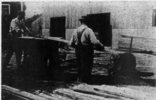
One Machine of the Type Shown Here Will Perform Many Operations, Such as Jointing, Grinding, Mitreing, Rabbeting and Dadoing. Many Lumber Dealers Are Installing Saw Rigs in Their Yards.
