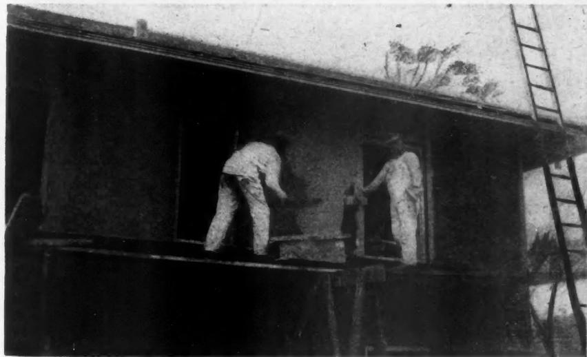
Figure 5. Applying Portland Cement Stucco to Concrete Block Surface. The Dash Coat Is Applied Directly to the Base Coat.
