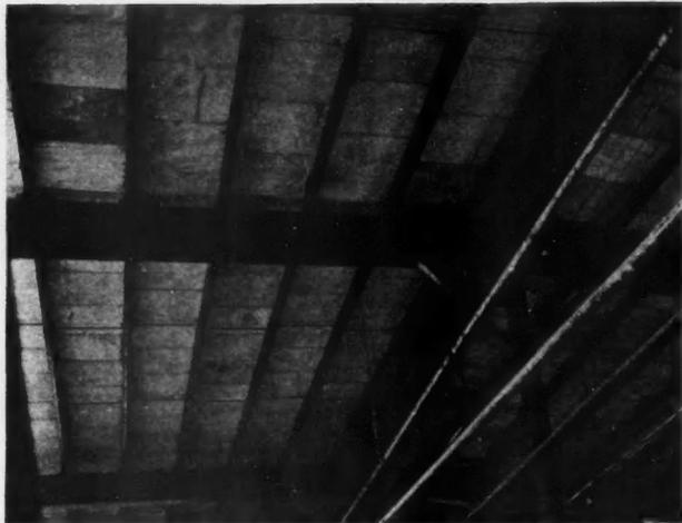
Underside of Roof Over Which Concrete Slabs Have Been Laid as Sheathing. This Material Can Carry Fairly Heavy Loads. Nails Can Be Driven Thru This Material to Wood Studs.
