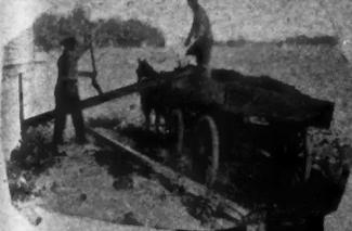
TODAY—Unloading 2 1/2 tons of coal from Kissel dump and motor truck takes 2 minutes, saving 28 minutes.
