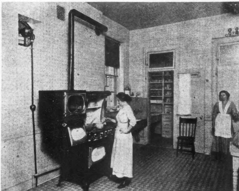
Carrying Away the Odors and Warm, Impure Air of the Kitchen, This Small Kitchen Ventilator Prevents the Smudge from Collecting on Curtains and Walls and Keeps the Kitchen Clean.
