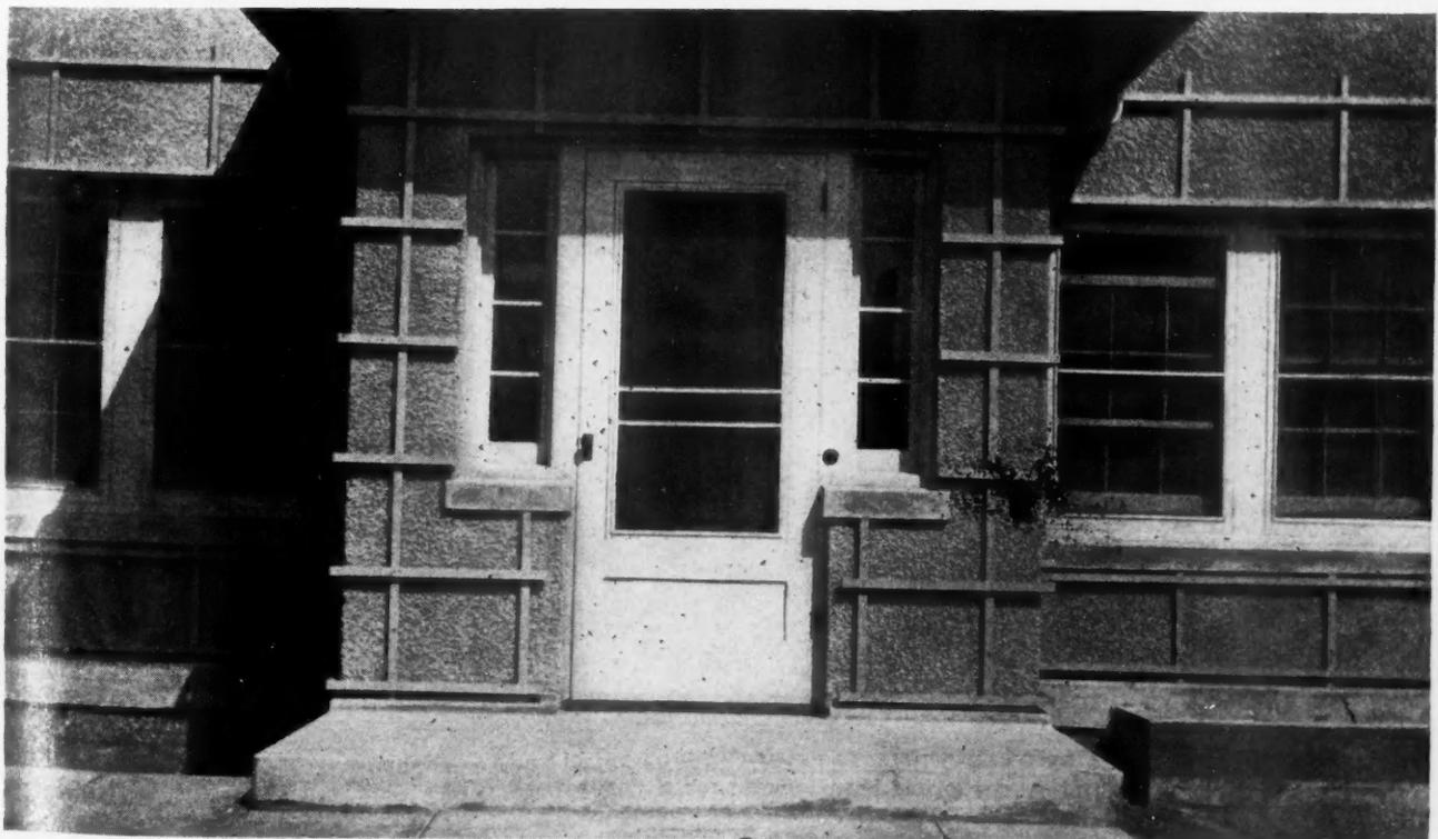
Detail of Front Entrance of Finished House, Showing Final Texture of Cement Stucco Finish. The wood lattice was added to soften the lines until shrubbery and vines have time to grow to do this work better.
