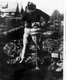
in trenches, removing granite block, removing wood block, drilling foundations, drilling through walls.
