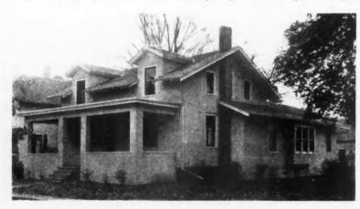
House Finished with Magnesite Stucco. Magnesite Is a Nonconductor of Heat and Cold; Keeps House Warm in Winter, Cool in Summer.
