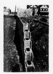
Retaining wall in course of construction built of ACME INTER-LOCKING TILE, showing con-tinuation of air spaces and interlocking features.
