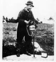
Upper Right Illustration Shows Gasoline Hammer Drill Used for Ramming Back Fill. Lower Left Shows Complete Drilling Unit Operating.
